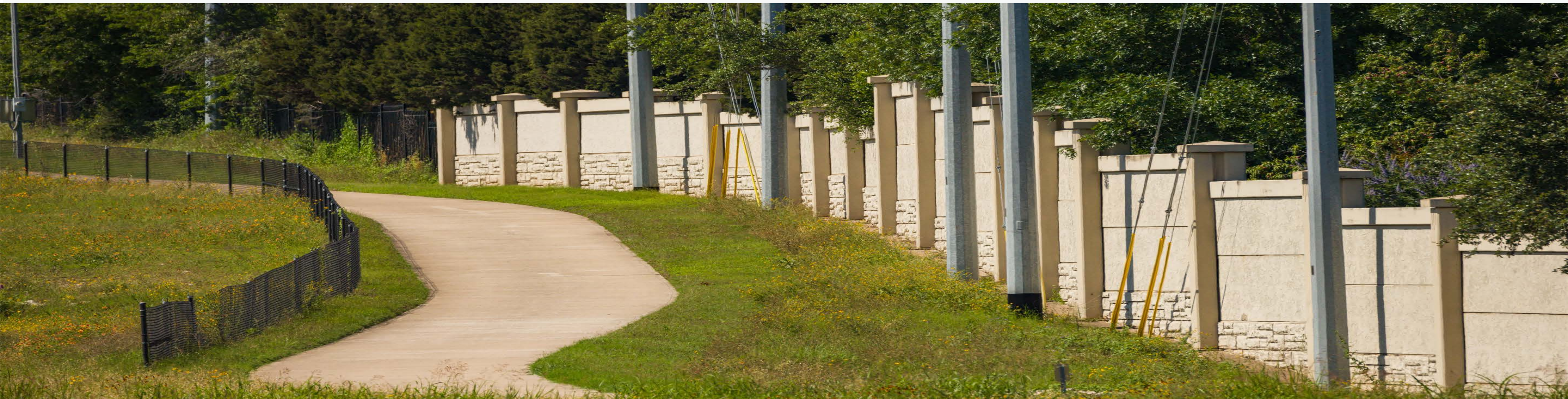
Pictured above: Existing noise barrier on 183A Toll, located between Brushy Creek Road and Park Street.
