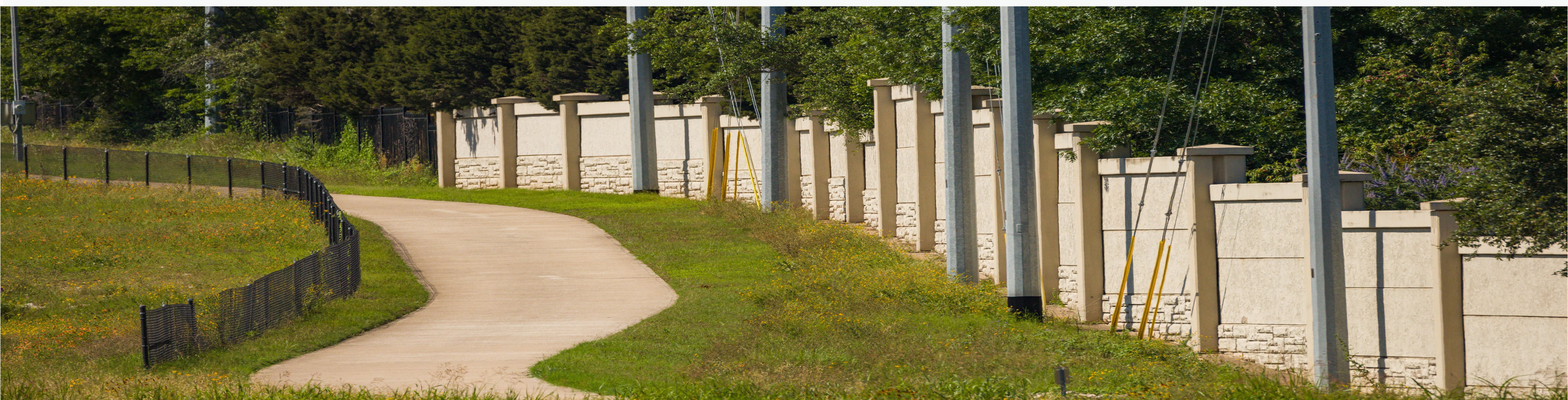
Pictured above: Existing noise barrier on 183A Toll, located between Brushy Creek Road and Park Street.
