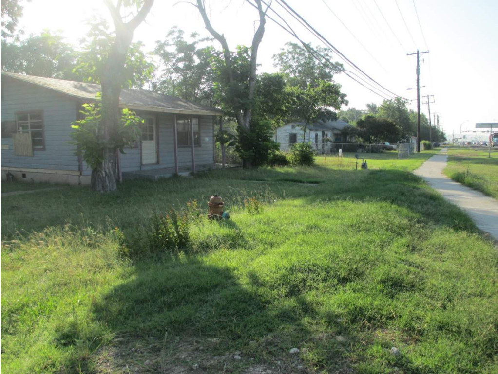
View of previously surveyed dwellings along SH 71 from Royster, camera facing west
