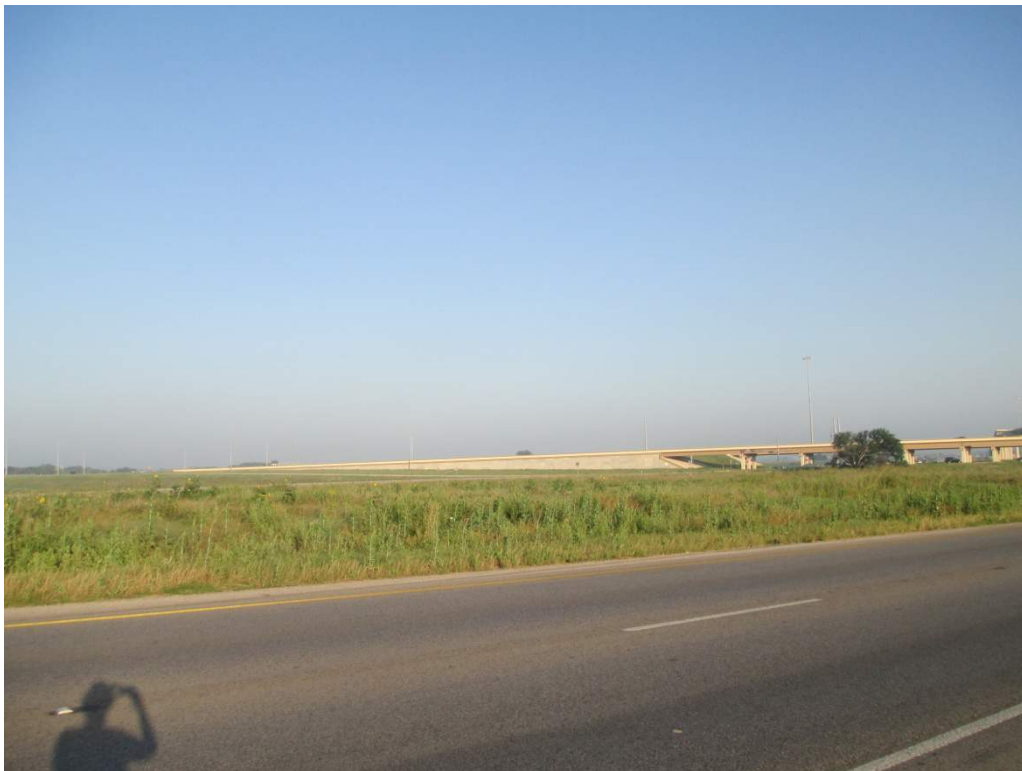
Setting view from project's eastern terminus towards SH 130, camera facing southwest
