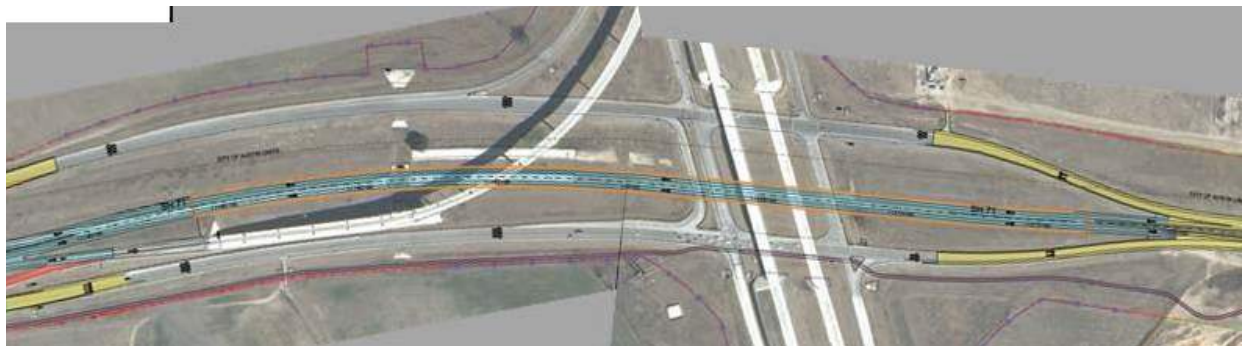
Figure 1-18: Aerial View at SH 130
