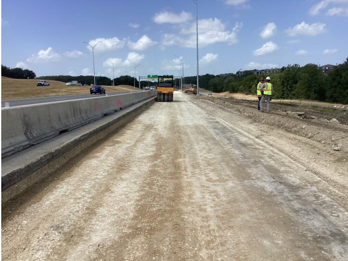
South of Barton Skyway July 2023
