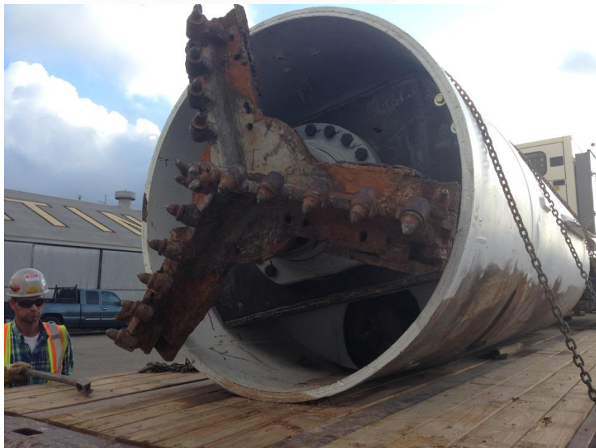
42-inch Waterline Boring Machine and Pit
