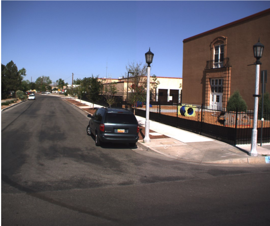
Sample image of street lighting collected with MAC LRIS system
