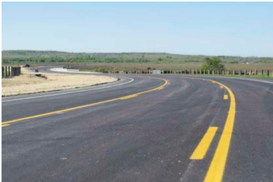
Kellam Rd. open to traffic
