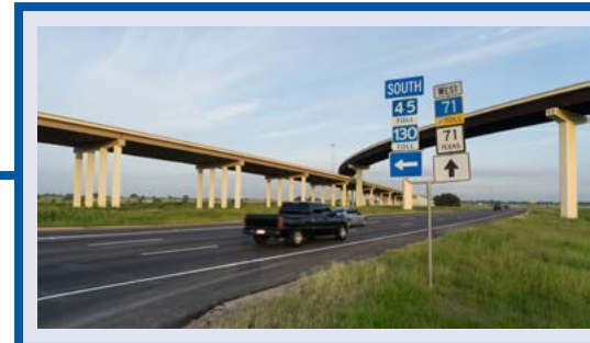
71 Toll Lane Opens
