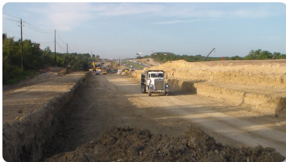
Excavation Work between Little Walnut Creek and Loyola Lane
