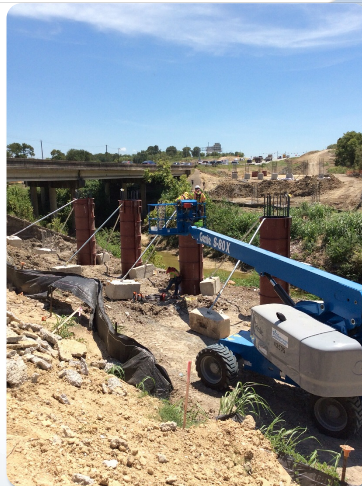
Setting Forms and Columns at Little Walnut Creek
