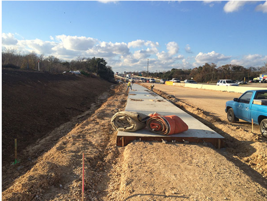
Ongoing construction of shared-use pathway along SH 71
