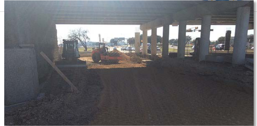
Ongoing construction of new westbound-to-eastbound U-turn at Presidential Boulevard
