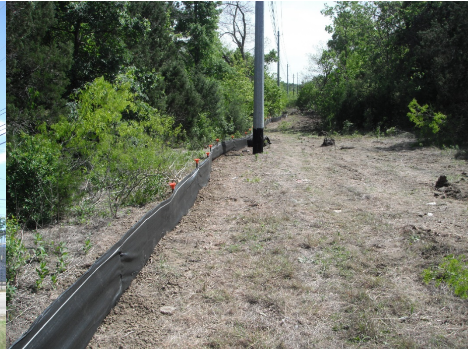
Erosion Control Installation/ Clearing and Grubbing
