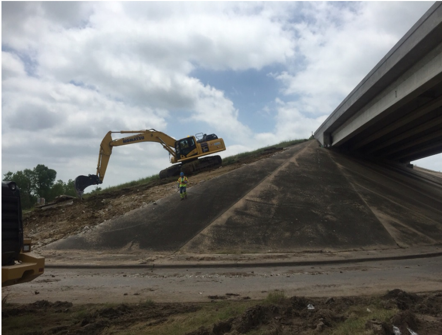
Clearing and Grubbing
