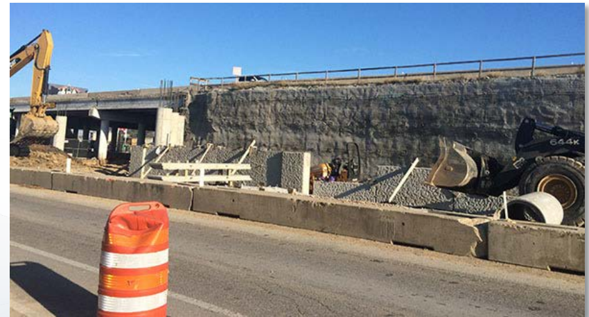
Construction of retaining wall at Presidential Boulevard
