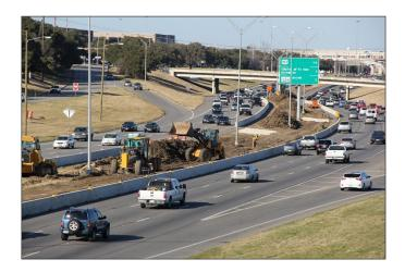
Work continues on clearing of vegetation, placement of erosion control devices, temporary lighting, rough grading, and removal of guard fence and existing railing.
