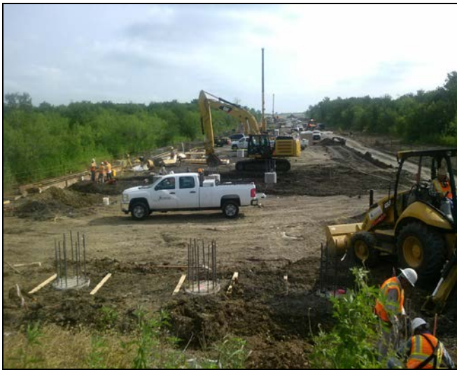
Maha Loop Construction
