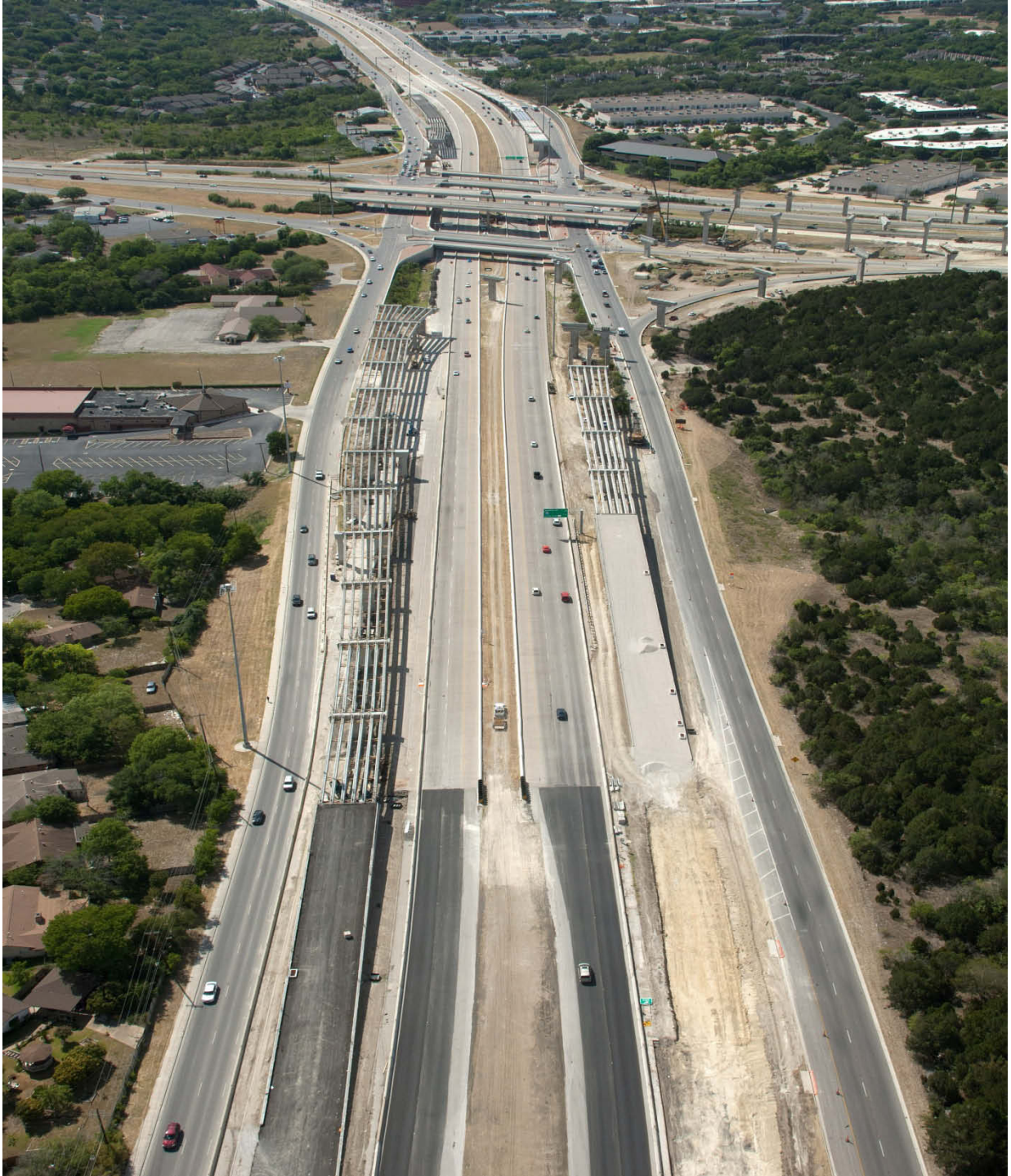
Interchange construction looking north (Taken 7/12/2011)
