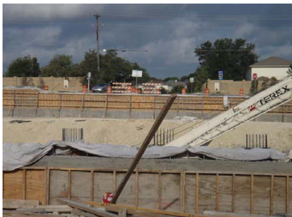
Excavation at Scottsdale Drive, looking west
