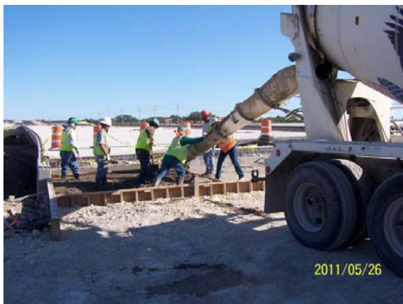
Placing supporting concrete for a bridge structure at Block House Creek
