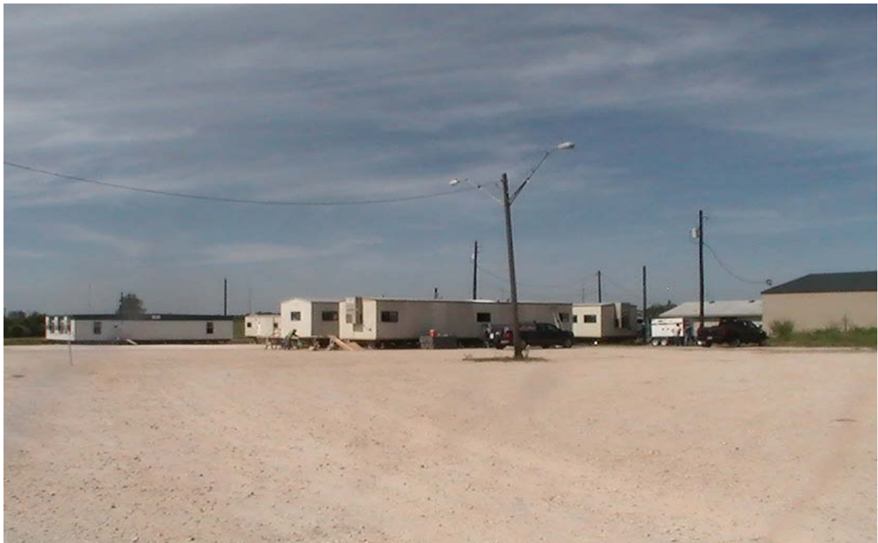
Mobilization of the Project field office along the existing US 290 East facility [taken July 14, 2011]
