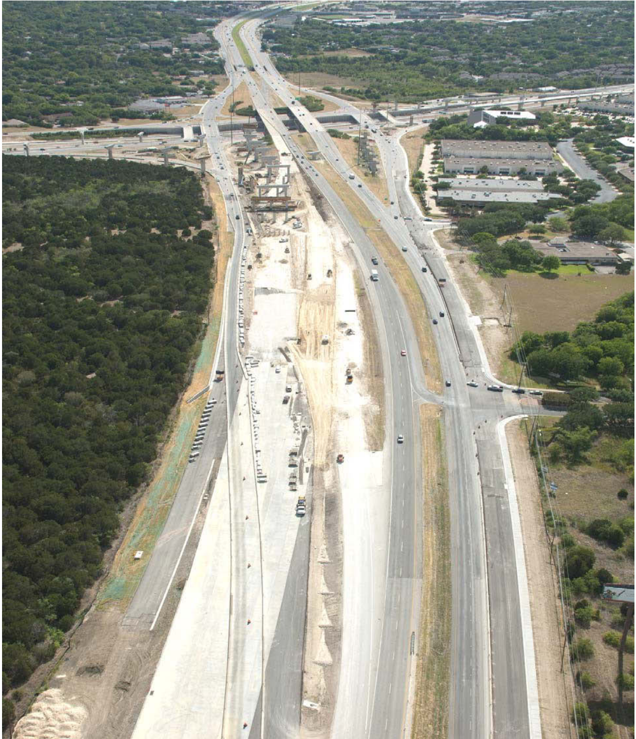
Interchange construction looking west (Taken 7/12/2011)
