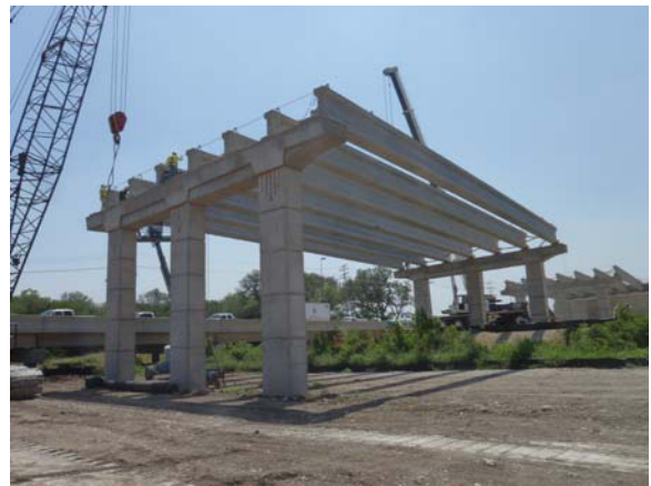
Concrete bridge beams at RM 2243
