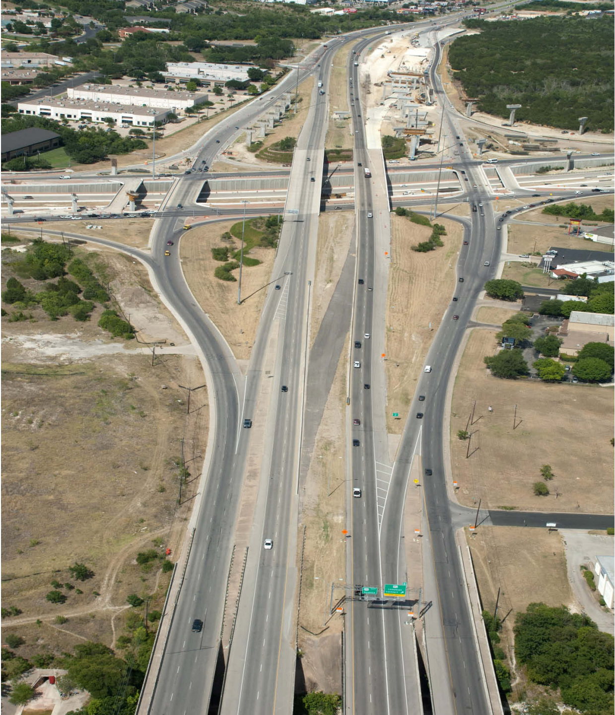
Interchange construction looking east (Taken 7/12/2011)
