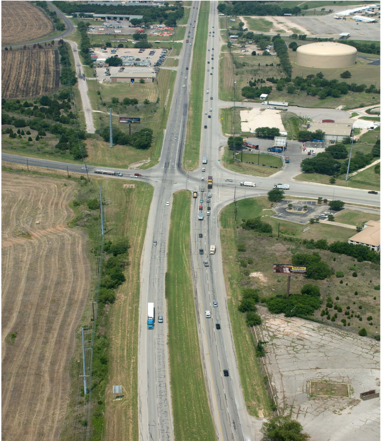
US 290 East at Giles Road Intersection looking west (Taken 6/7/2011)
