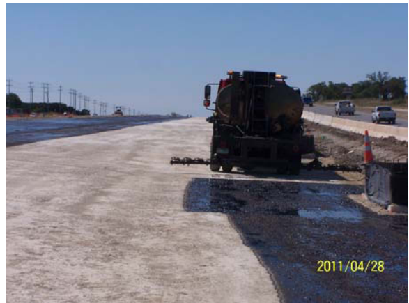
Placing asphalt on the cement-treated base near Block House Creek
