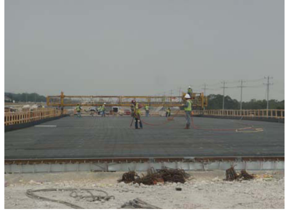
Preparing bridge deck for concrete placement at Block House Creek
