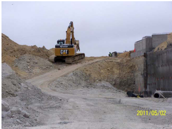
Excavation at the Scottsdale Drive Underpass
