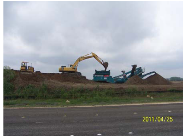
Sifting top soil near the north end of the project
