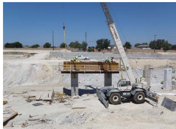
Bridge construction at Scottsdale Drive
