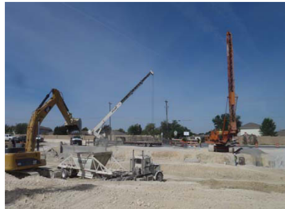
Drilled shaft construction at future Scottsdale Drive bridges
