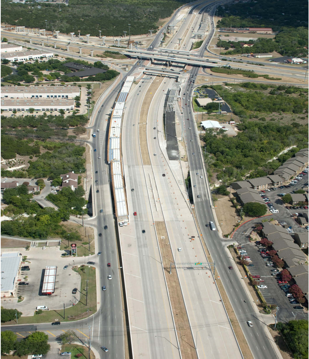
Interchange construction looking south (Taken 7/12/2011)
