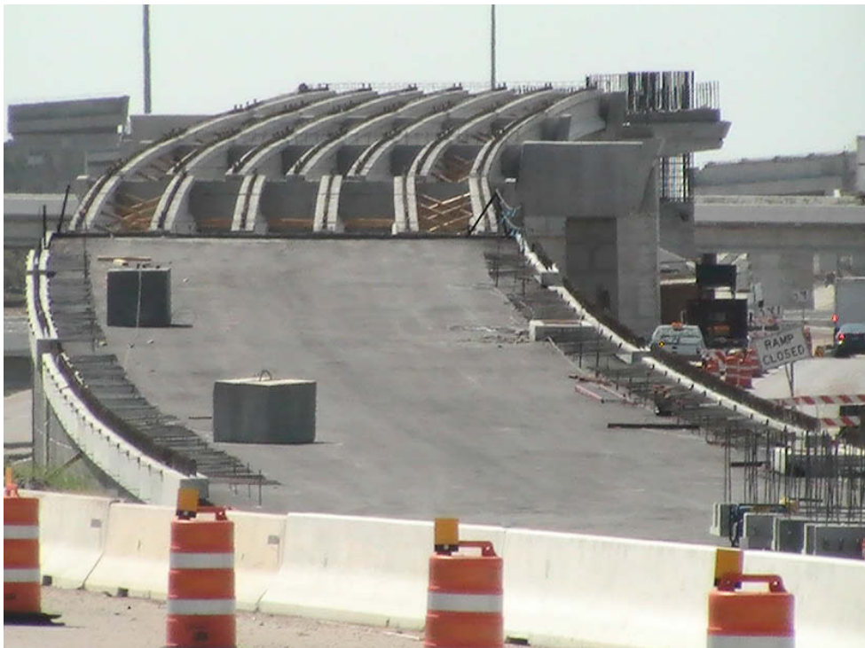
South to East direct connector approach looking south (Taken 7/6/2011)
