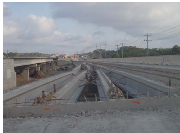
Widening the bridge at Block House Creek
