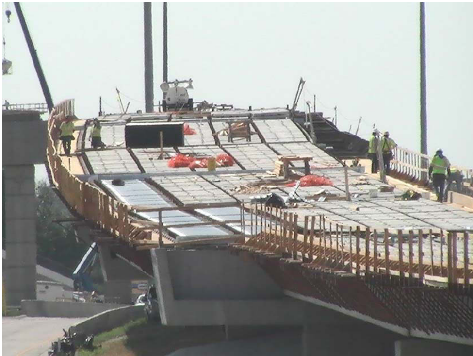
West to North direct connector Spans 5 & 6 (Taken 7/6/2011)
