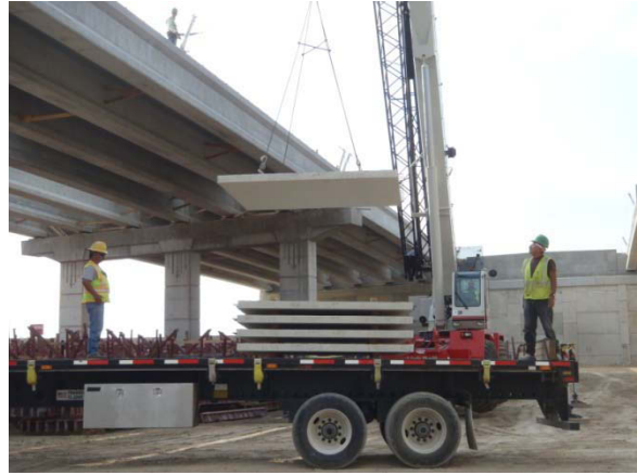
Placing concrete deck panels at Crystal Falls Parkway
