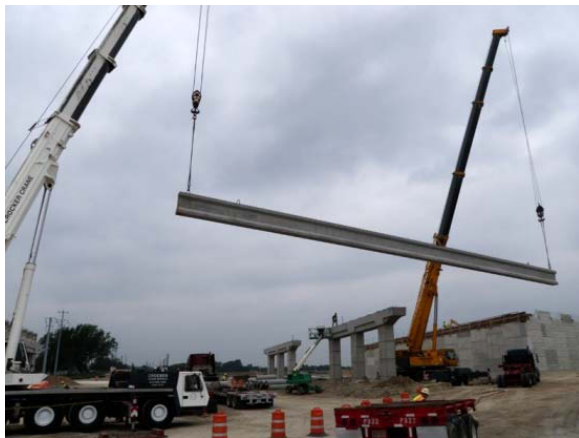
Placing beams at the 183A bridges over Hero Way
