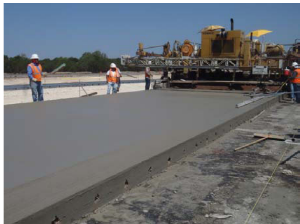
Applying surface finish to concrete pavement
