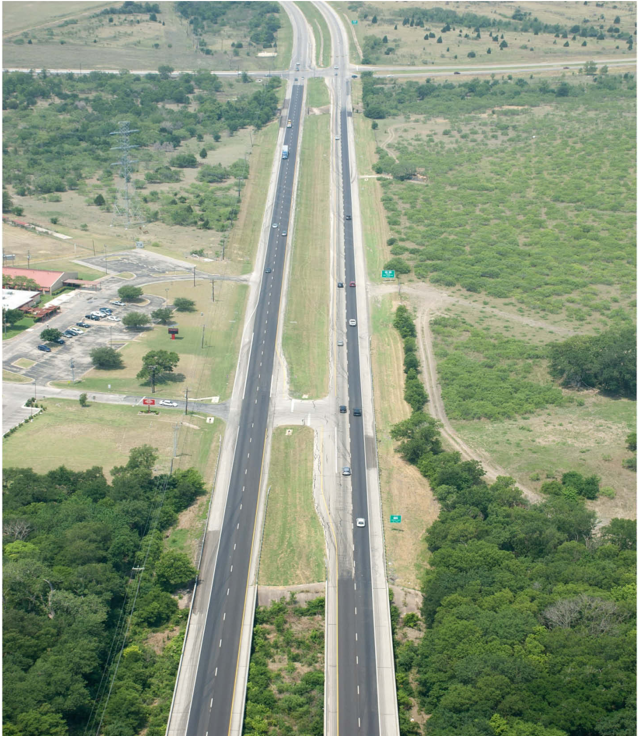
US 290 East looking west from Gilleland Creek (Taken 6/7/2011)
