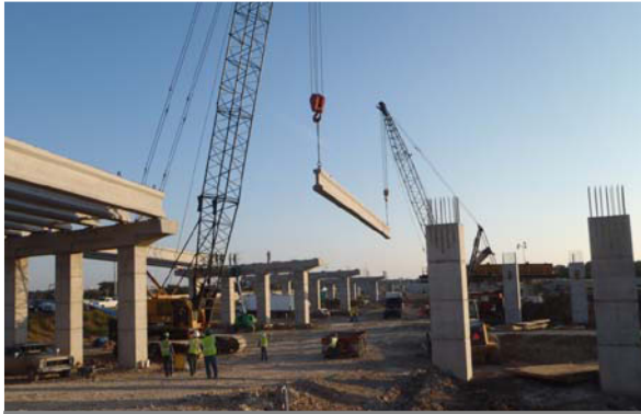
Beam Placement at New Hope Drive in October
