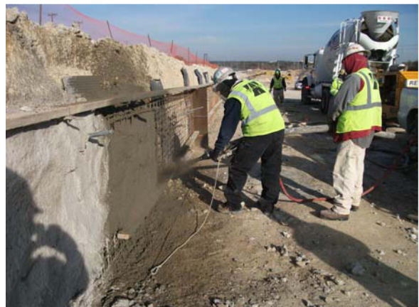
Soil nail wall installation at Scottsdale Drive
