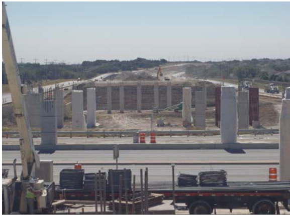
Progress at Crystal Falls Parkway. Left: Columns in October – facing south, Right: Cap placement on columns in anticipation of beams in December – facing south
