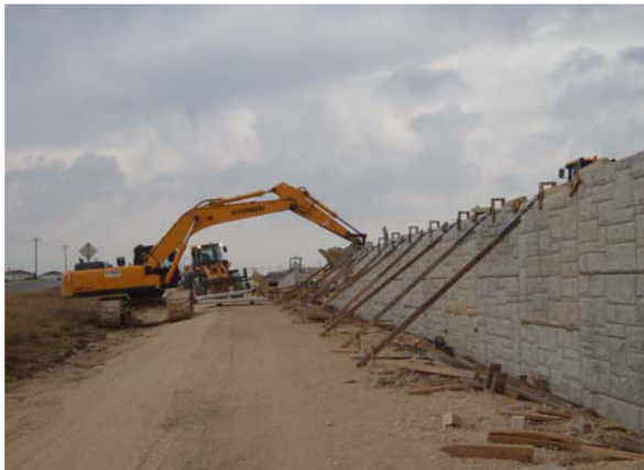
Placing MSE walls and structures north of New Hope Drive
