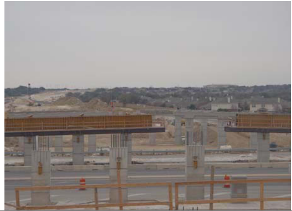
Progress at Crystal Falls Parkway. Left: Columns in October – facing south, Right: Cap placement on columns in anticipation of beams in December – facing south
