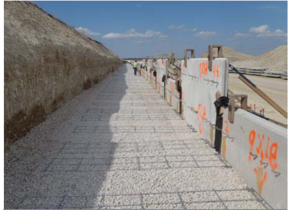
Placing MSE wall and structures south of RM 2243
