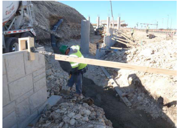
Placing MSE wall and structures south of Crystal Falls Parkway
