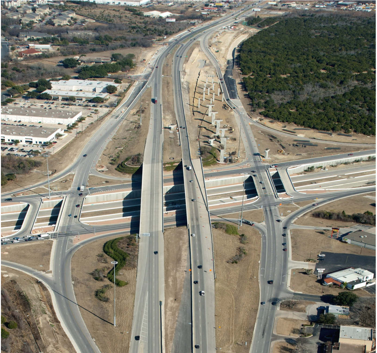
Interchange construction looking east (Taken 1/11/2011)
