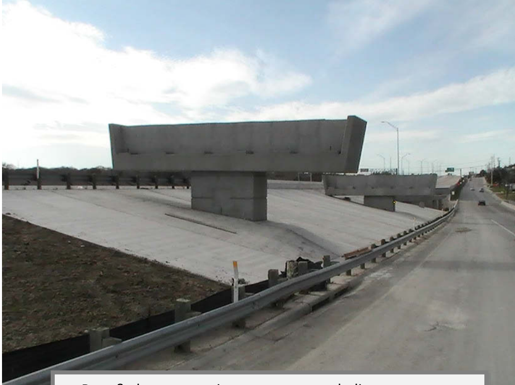
Bent & slope protection at west to north direct connector (Taken 1/14/2011)
