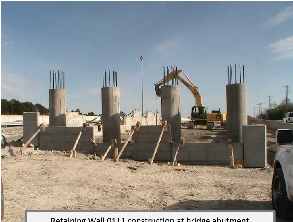
Retaining Wall 0111 construction at bridge abutment (Taken 1/14/2011)
