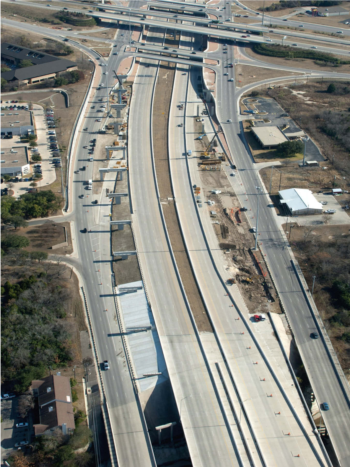
Interchange construction looking south (Taken 1/11/2011)
