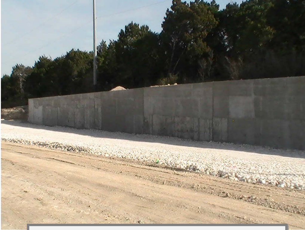
Retaining Wall 0117 & eastbound frontage road construction (Taken 1/14/2011)
