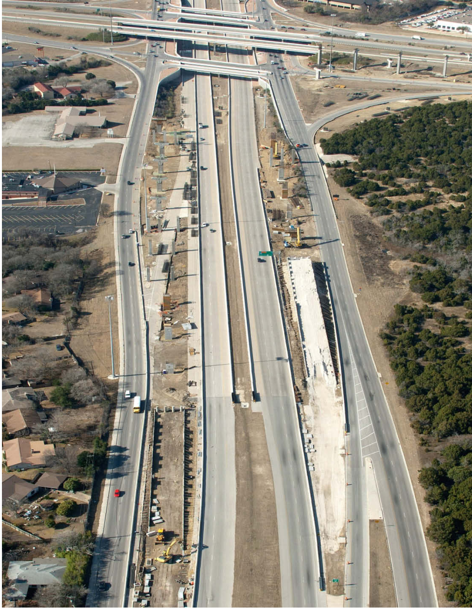
Interchange construction looking north (Taken 1/11/2011)
