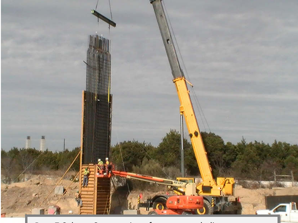
Bent 7 Column Construction of west to north direct connector (Taken 1/14/2011)
