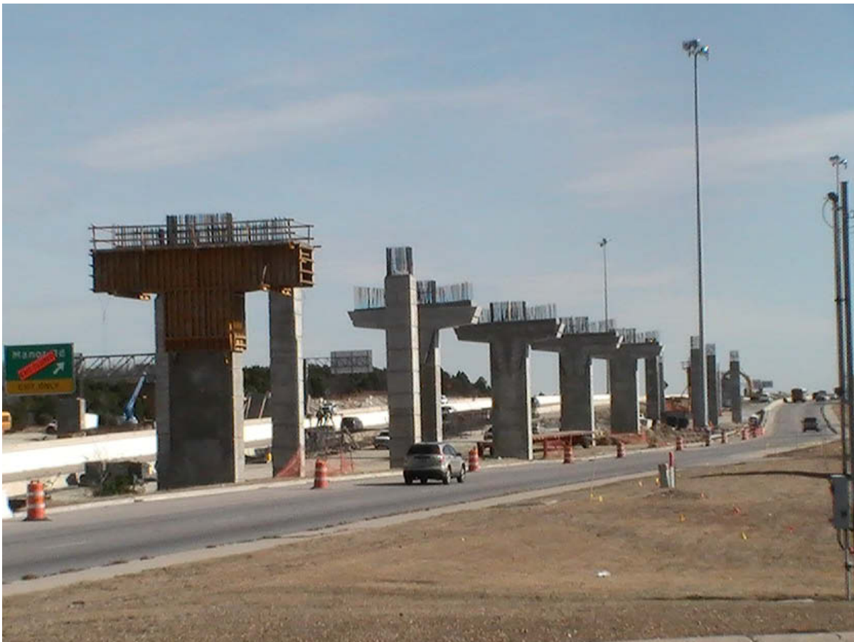
Bents 5 thru 13 on south to east direct connector [taken January 7, 2011]
