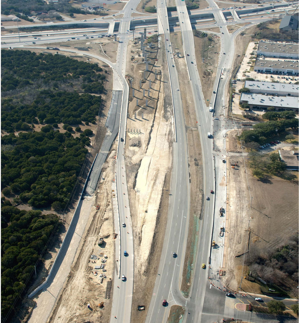
Interchange construction looking west (Taken 1/11/2011)
