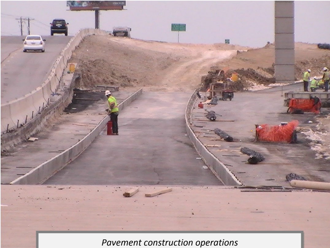
Pavement construction operations (Taken 4/14/2011)
