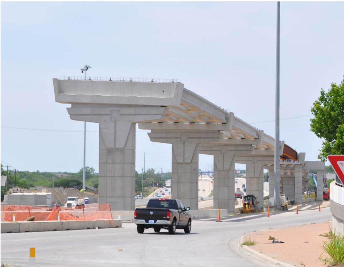
Ongoing construction work at the west to north direct connector [taken April 13, 2011]
