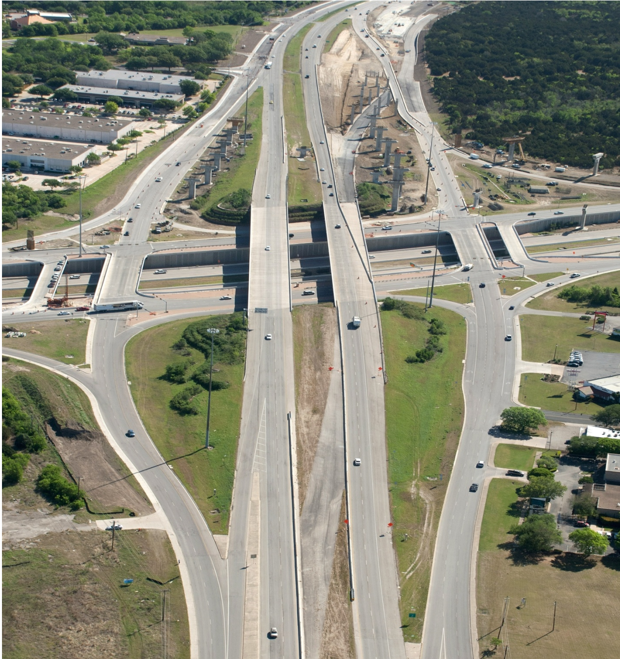
Interchange construction looking east (Taken 4/11/2011)
