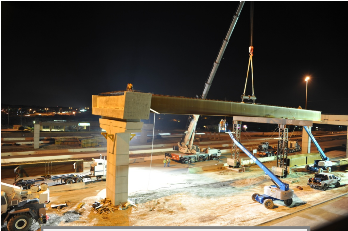
Setting of steel beams at west to north direct connector (Taken 1/27/2011)
