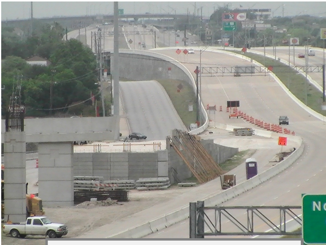
Direct connector abutment construction (Taken 4/14/2011)
