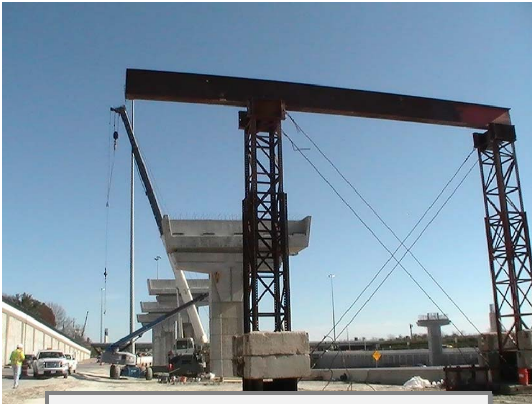
Beam setting preparation (Taken 4/14/2011)
