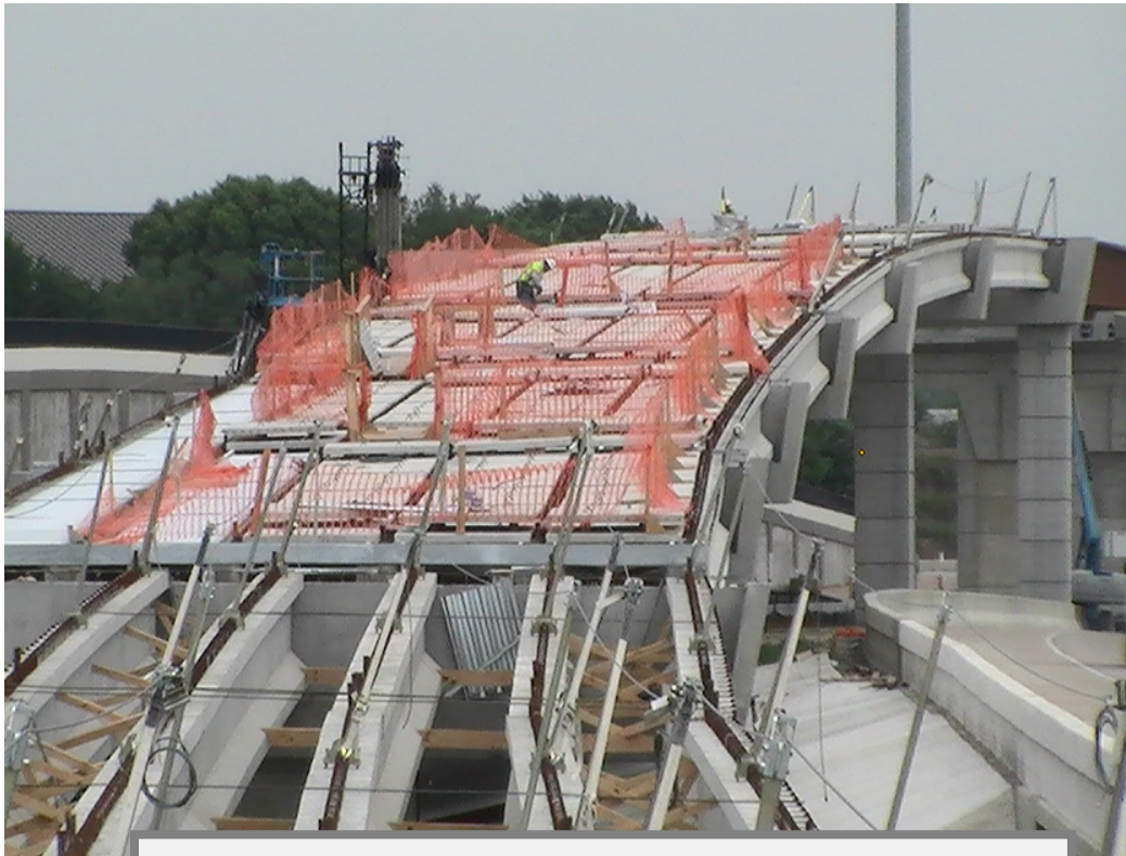
Bridge deck preparation at west to north direct connector (Taken 4/14/2011)
