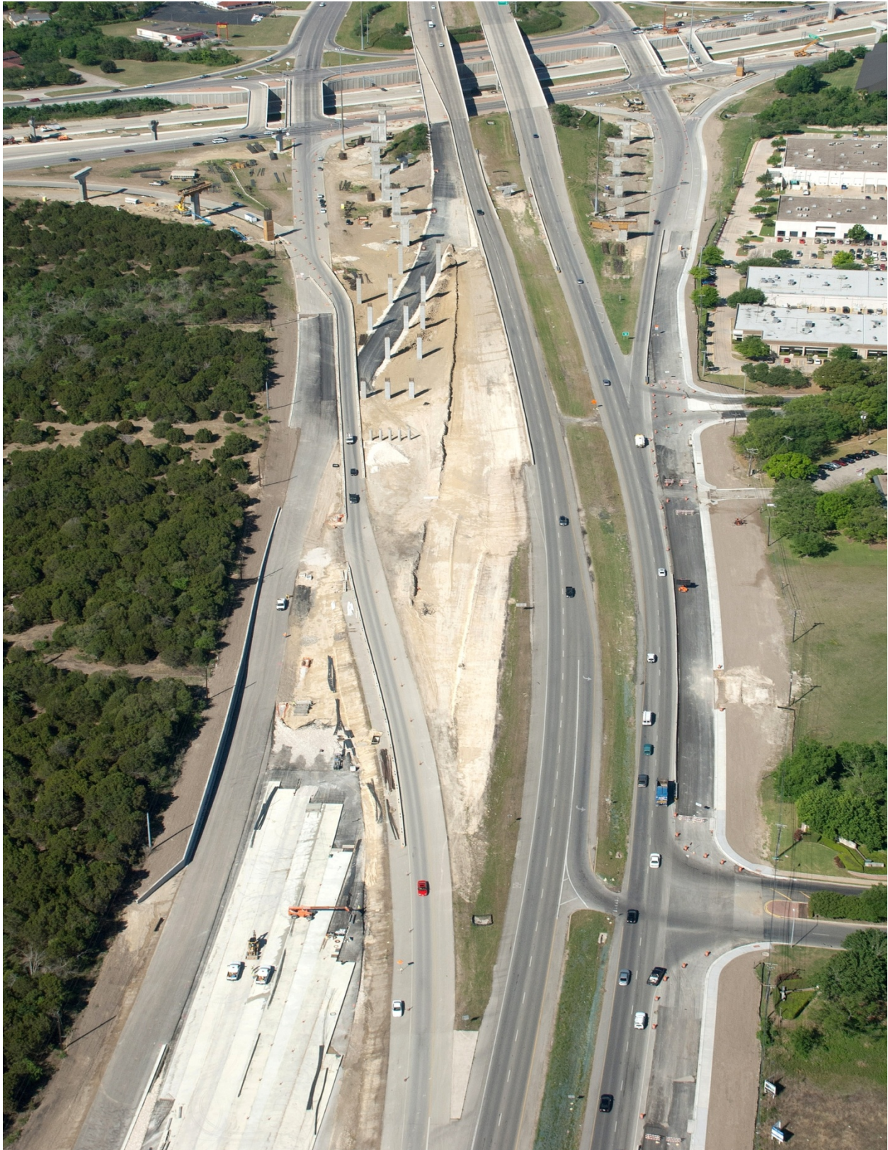
Interchange construction looking west (Taken 4/11/2011)
