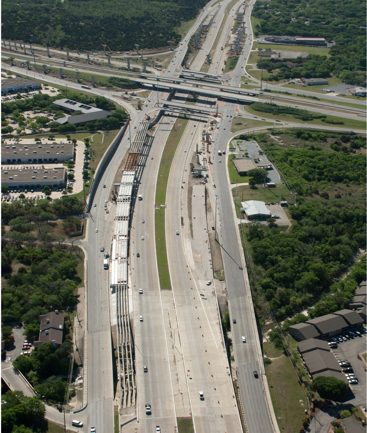
Interchange construction looking south (Taken 4/11/2011)
