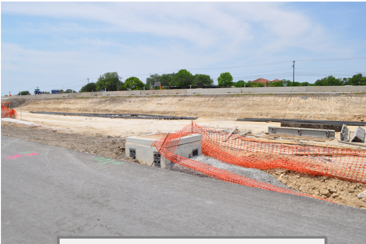
Roadway appurtenance construction (Taken 1/14/2011)
