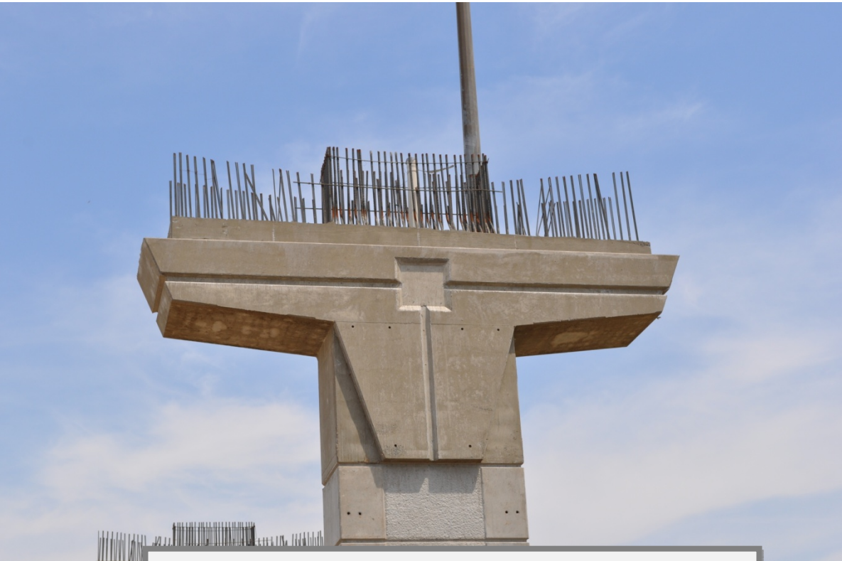
Bent construction at west to north direct connector (Taken 4/14/2011)
