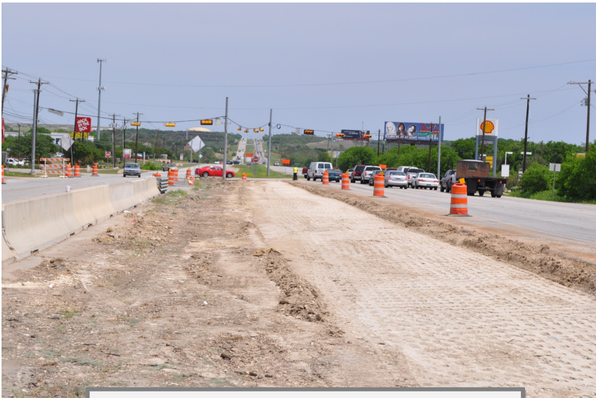
Earthwork near Tuscany Way intersection (Taken 4/14/2011)
