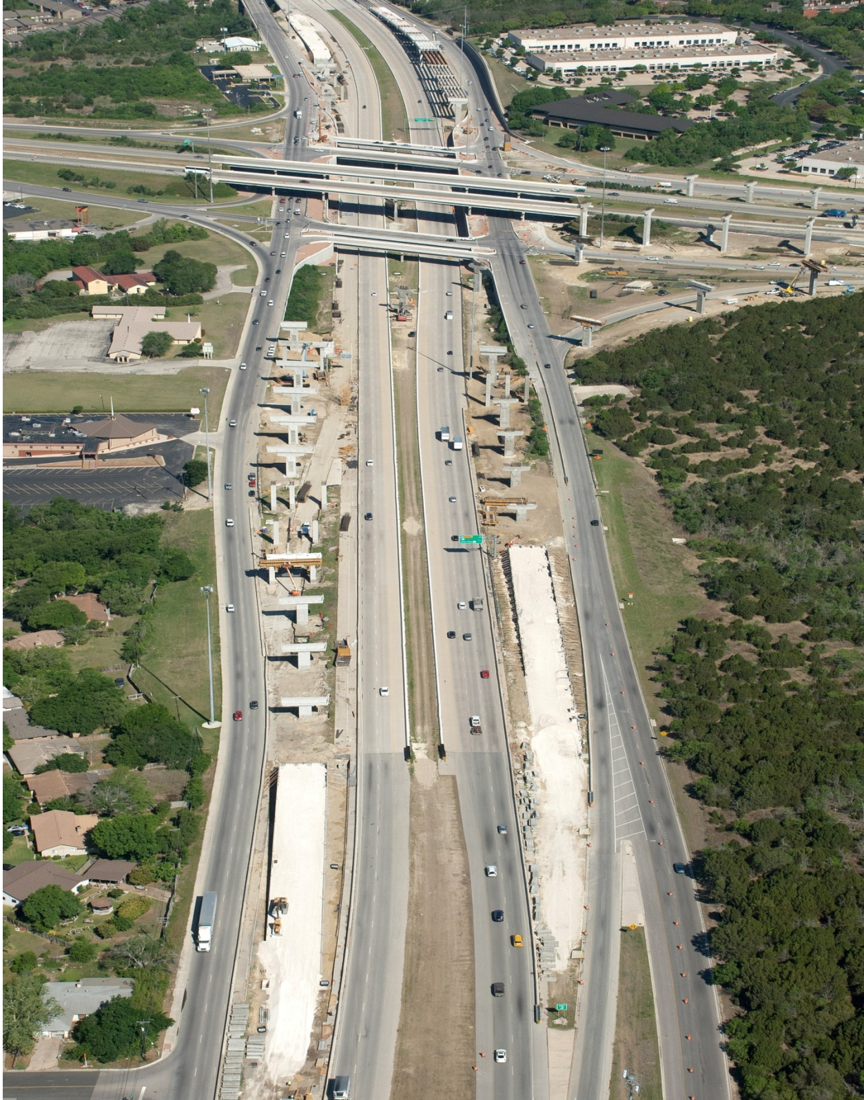
Interchange construction looking north (Taken 4/11/2011)
