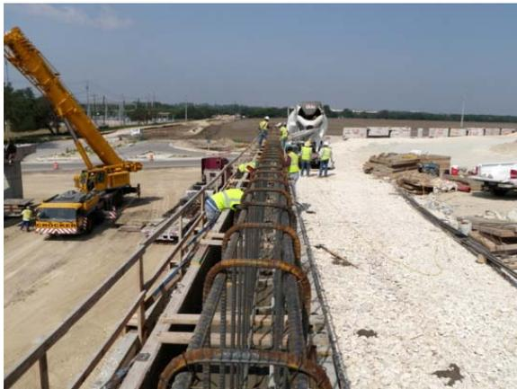
Placing concrete at a back wall for the 183A bridge over Hero Way
