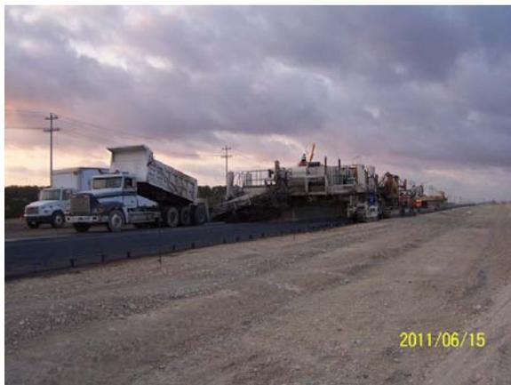
Placing concrete for paving on the mainlanes north of Crystal Falls Parkway
