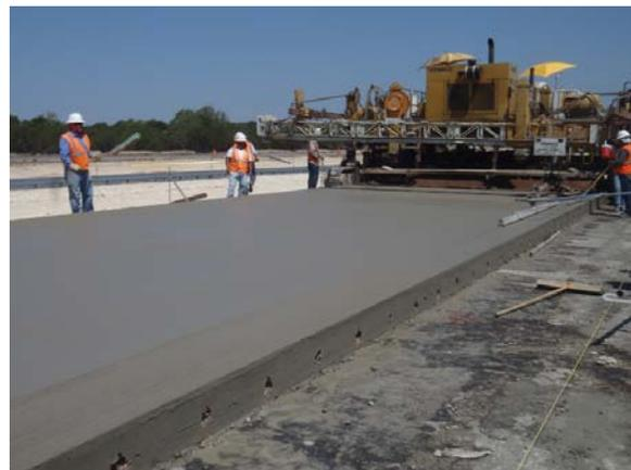
Applying surface finish to concrete pavement
