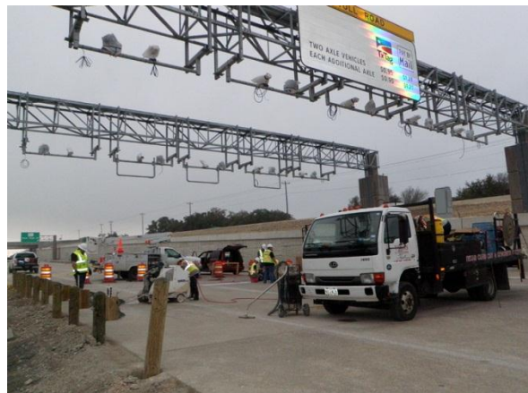
Toll system construction at Scottsdale Drive
