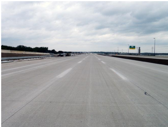
Striping on the new 183A mainlanes
