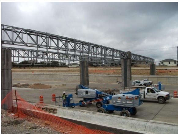
Construction of the mainlane toll gantries north of Scottsdale Drive
