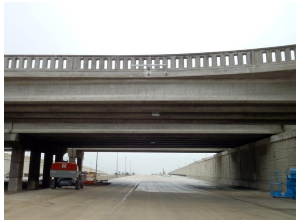
At Scottsdale Drive, the sign mount for the bridge clearance sign
