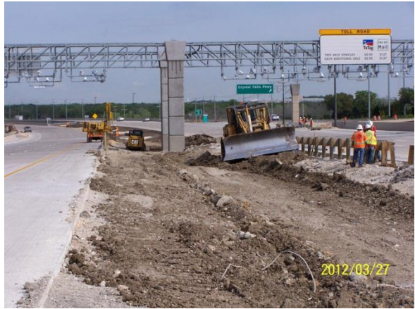
Installing metal beam guard fence at the Crystal Falls Mainline Plaza
