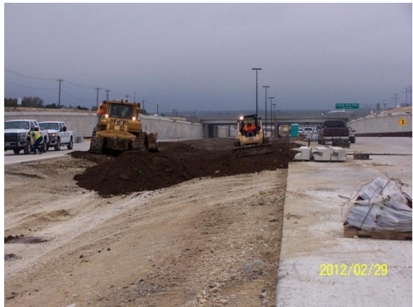
Placing topsoil in the median between the mainlanes
