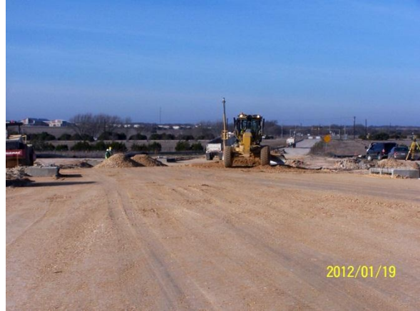
Construction of the future intersection of 183A and San Gabriel Parkway
