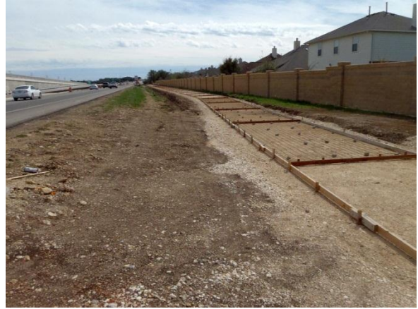
Placed forms in anticipation of laying concrete on the path
