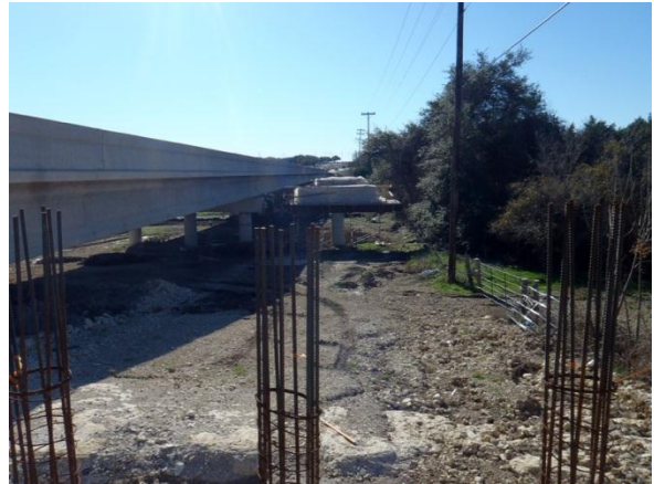
Drilled shaft construction at the pedestrian bridge over Brushy Creek
