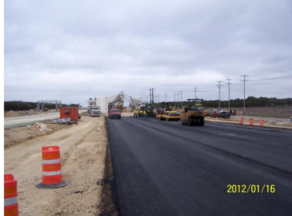
Placing a layer of asphalt pavement on the future northbound mainlanes
