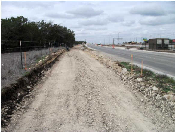
Preparation of the ground for the path
