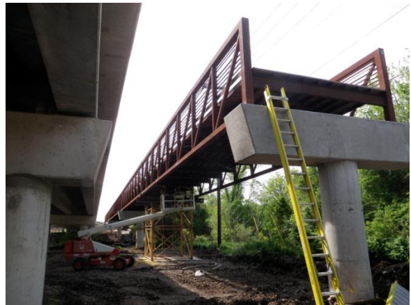
Construction and assembly of the pedestrian bridge over Brushy Creek
