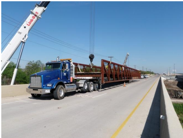
Preparing for placement of the pedestrian bridge over Brushy Creek
