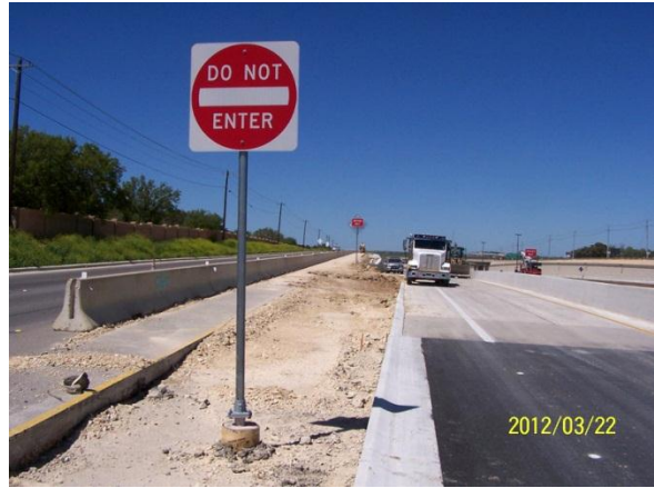
Placement of permanent roadway signs along the project
