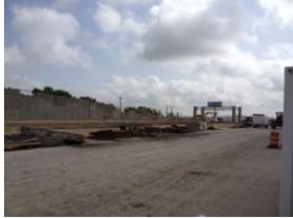
Retaining Wall for West-North Direct Connector (Looking North)
