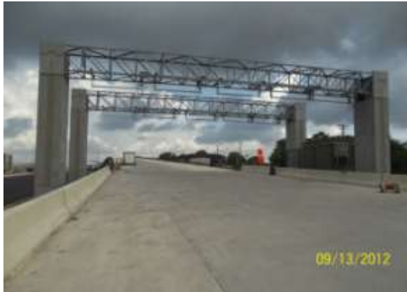
West to North Toll Gantry Columns (Looking West)
