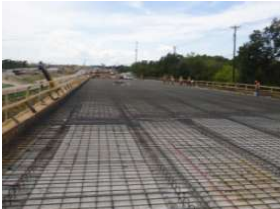
Westbound frontage road bridge construction at Walnut Creek (Looking West)
