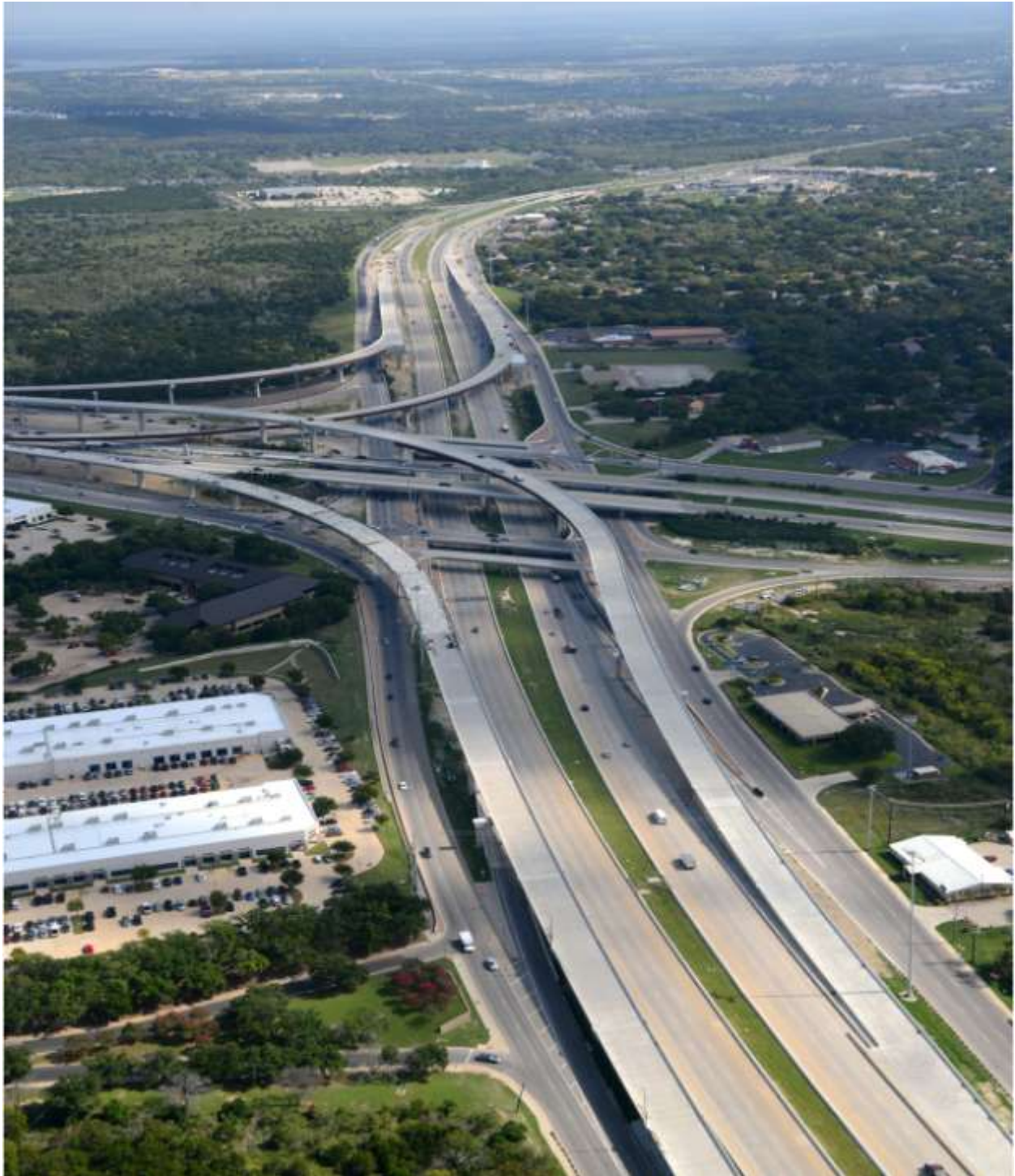
Manor Expressway Phase I Project (Looking South from US 183) (Taken 10/04/2012)
