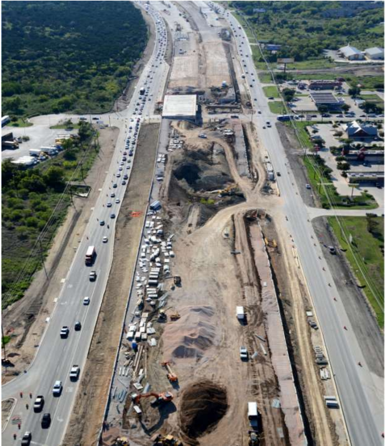
US 290 East at Springdale Road looking west (Taken 9/21/2012)
