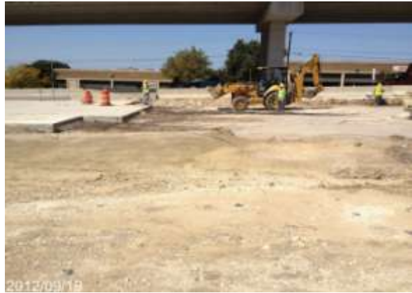
Completed US 290 Mainlane Concrete Paving (Looking North)
