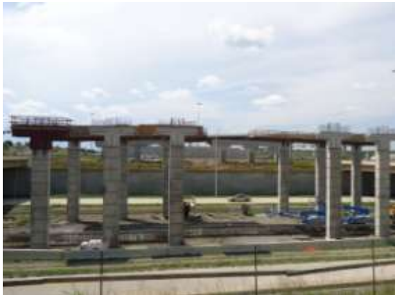
Construction of bridge columns for eastbound mainlanes at SH130 (Looking West)
