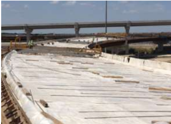
Curing Blankets Placed After Bridge Deck Pour (Looking North)
