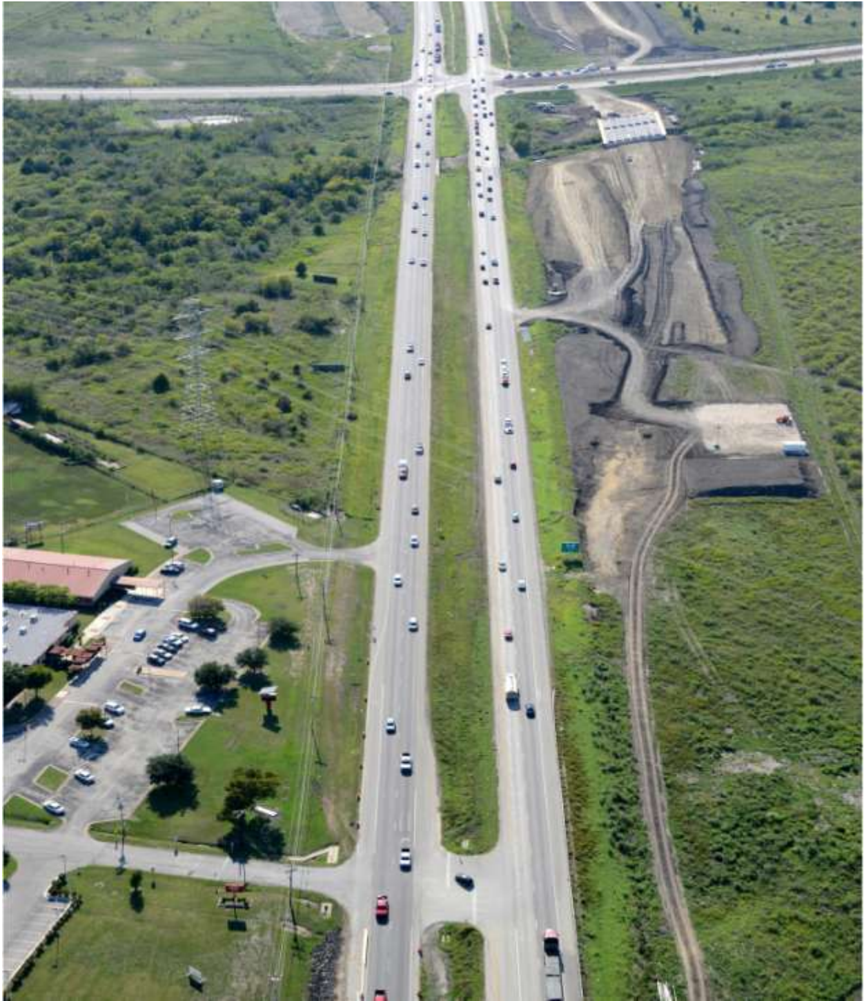
US 290 East looking west from Gilleland Creek (Taken 9/21/2012)
