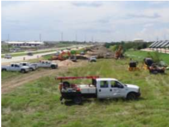
Duct bank construction west of Harris Branch Parkway (Looking West)
