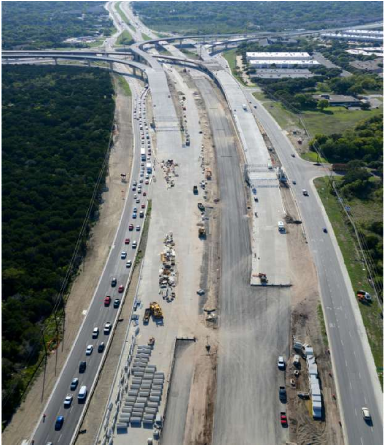
US 290 East at Tuscany Way looking west (Taken 9/21/2012)
