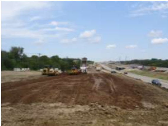
Embankment on the westbound frontage road at Tributary #5 (Looking East)
