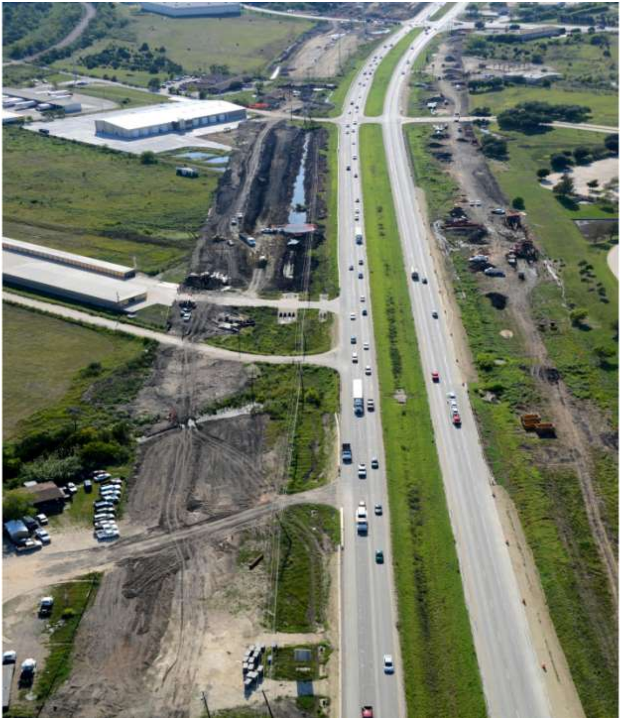
US 290 East at Crofford Lane Intersection looking west (Taken 9/21/2012)
