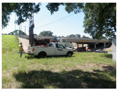
**Daytime Drill Rig Operation to Obtain Soil Samples**
