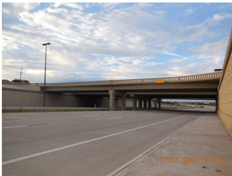
Scottsdale bridge over Mainlanes
