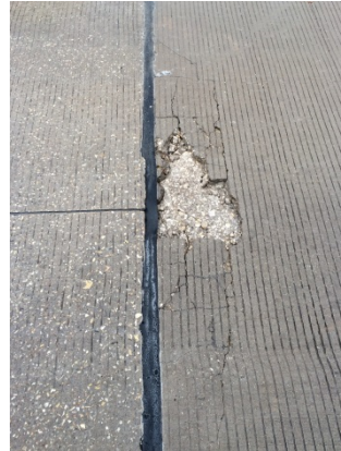
Southbound Entrance Ramp at Brushy Creek Loop
