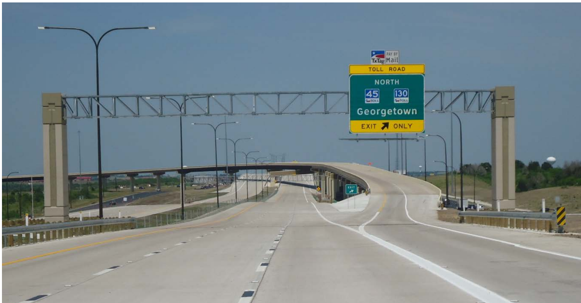
Overhead sign structure eastbound approaching SH 130
