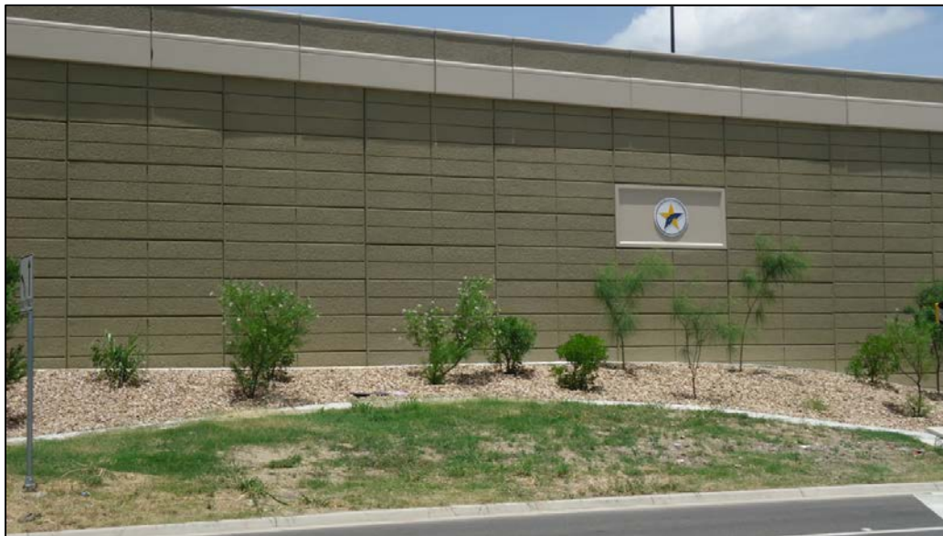
Retaining wall along the eastbound Manor Expressway west of Springdale Road
