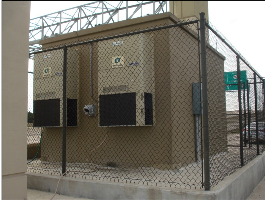
ILP building located at the WNDC toll location
