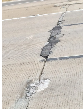
Southbound Mainlanes North of RM 1431
