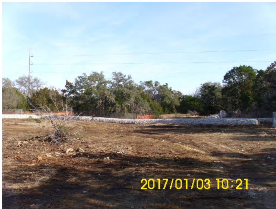
At GS2: Environmental Protection Device at Culvert 4 and F29D
