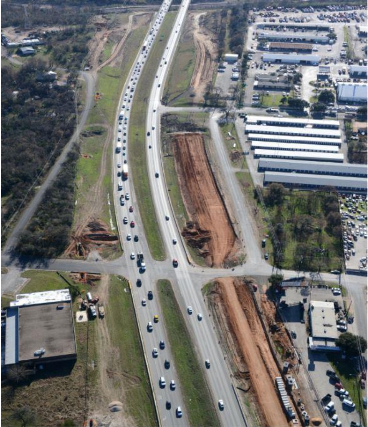
183 at Hudson St and Harold Ct (Looking South)
