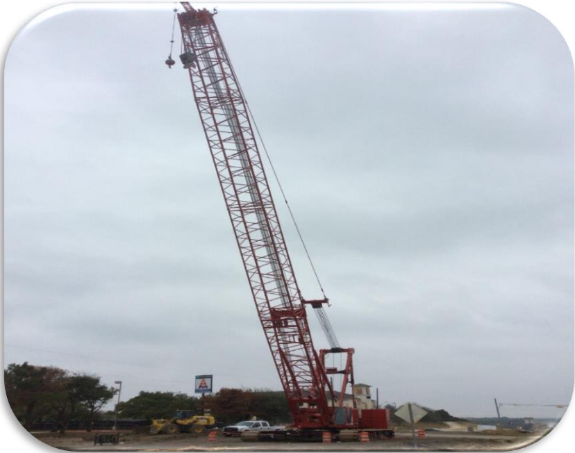
Contractor completed delivery and assembly of Manitowoc 2250 Crane [December 15, 2016]
