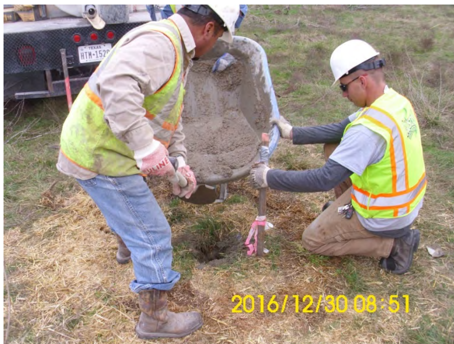
At GS1: Filling PF-001 (Borehole B-9) with Concrete Grout
