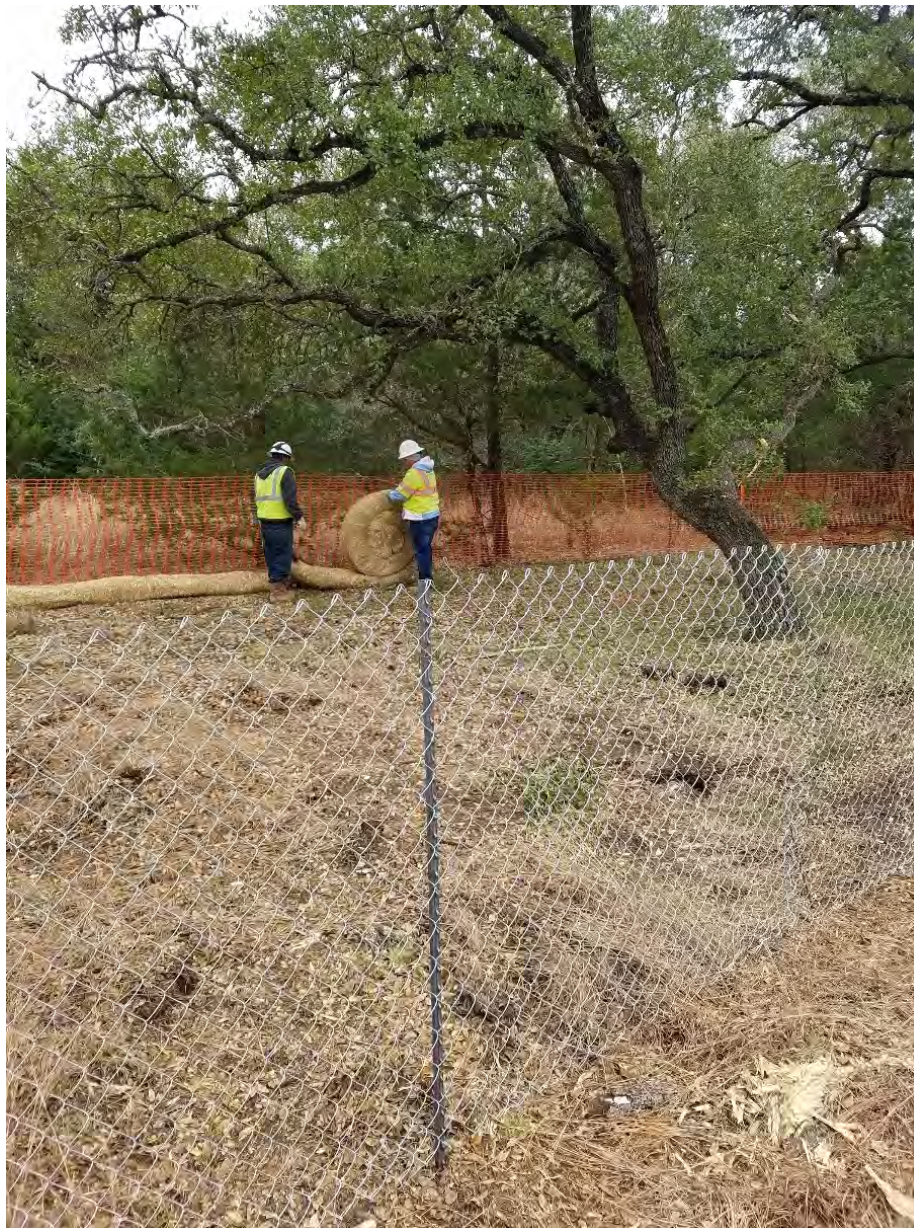
At GS2: Placing Biodegradable Erosion Control Logs
