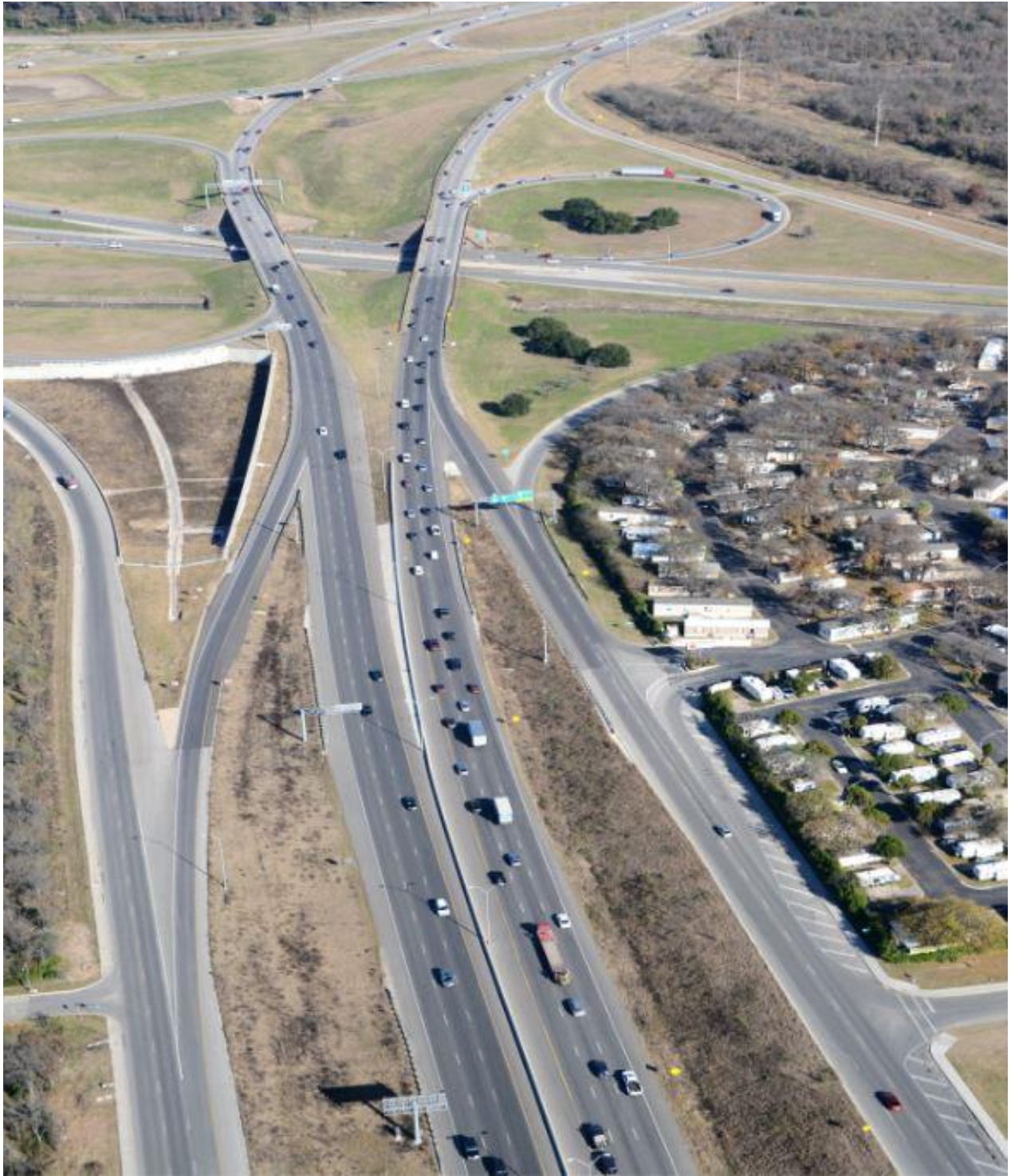
WB/EB SH 71 at 183 Interchange (Looking East) [December 22, 2016]
