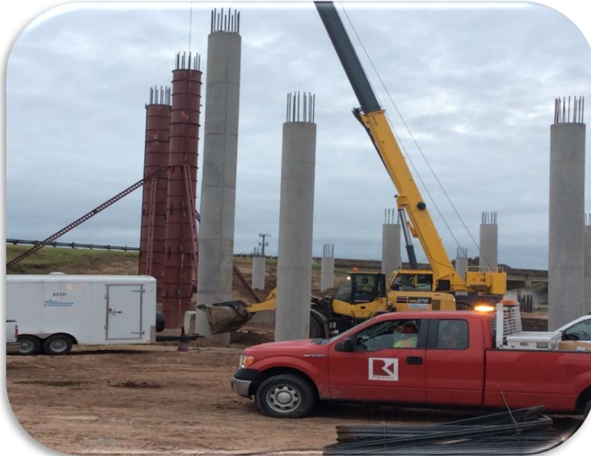
Southbound Main Lanes Bridge Construction near Levander Loop [December 2, 2016]
