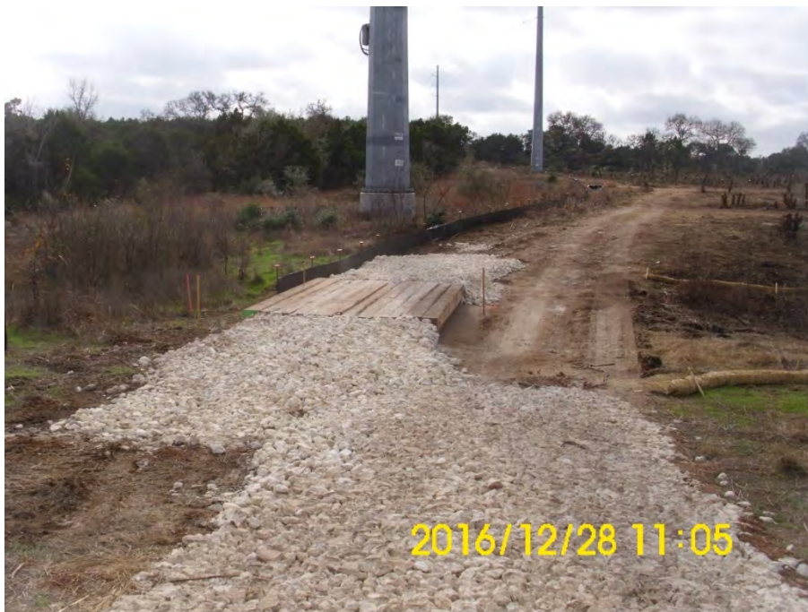
At GS2: Temporary Crossing at Danz Creek Area
