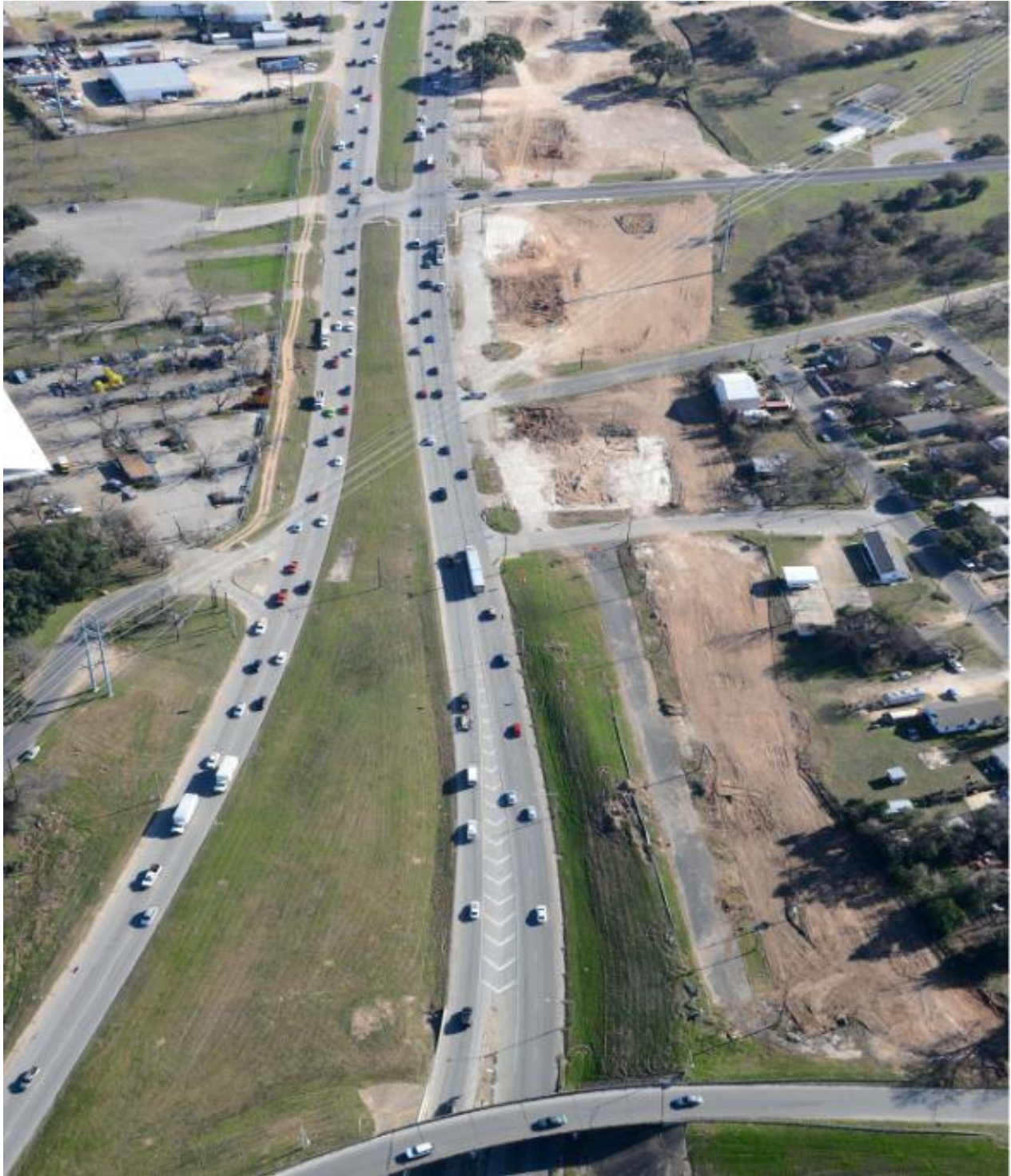
183 Near Vargas Rd (Looking South)
