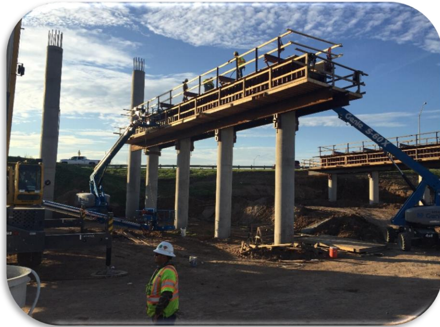
Cesar Chavez Street Bridge Construction at Southbound 183
