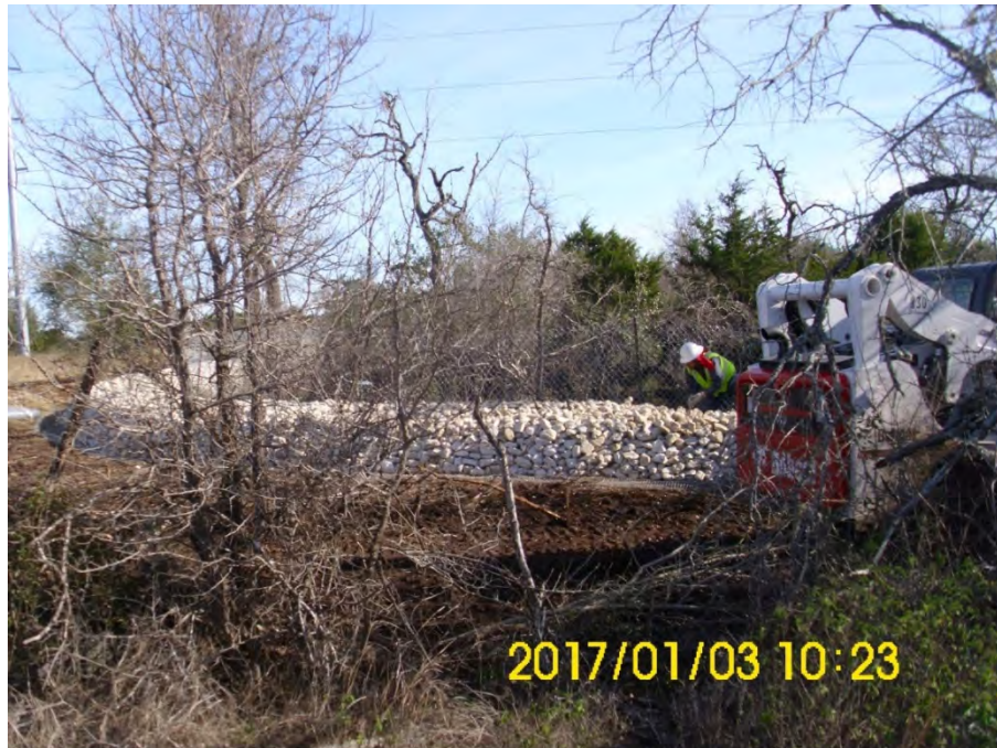
At GS2: Rock Filter Dam Installation at Sensitive Feature F41
