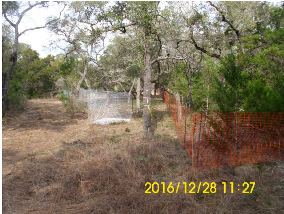
At GS2: Perimeter and Tree Protection Fencing
