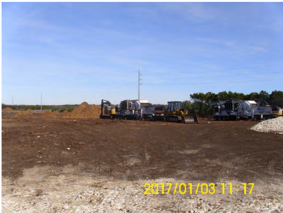
At GS1: Clearing and Mulching Complete in GS1
