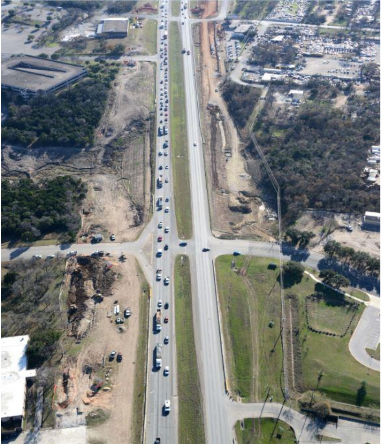
183 at Central Ave (Looking South) [December 22, 2016]
