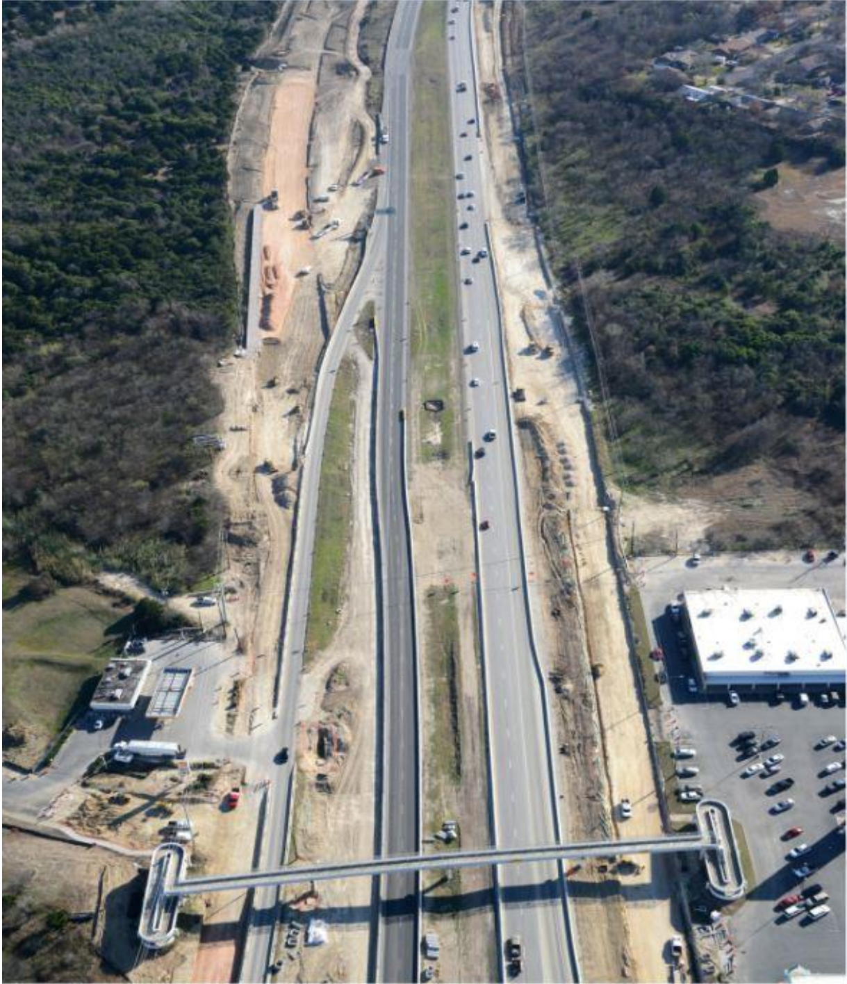
183 at Purple Sage Pedestrian Bridge (Looking South)
