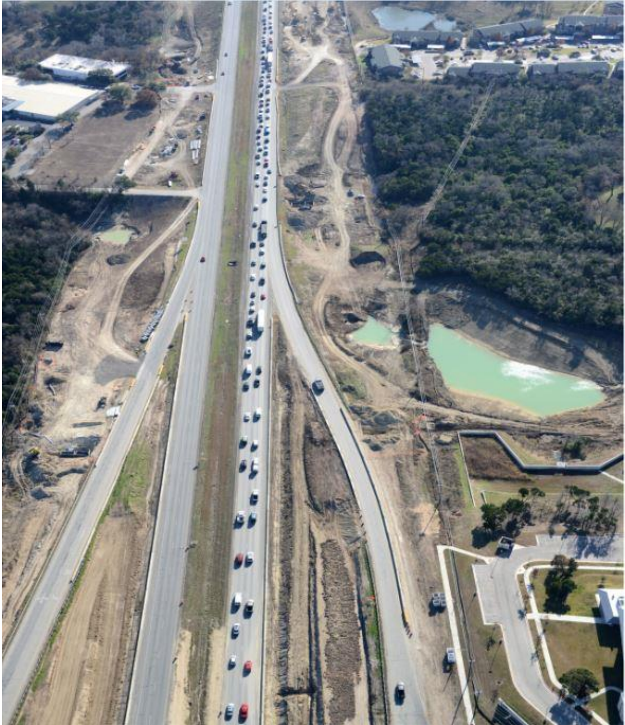
183 just South of FM 969/MLK Jr Blvd (Looking South)
