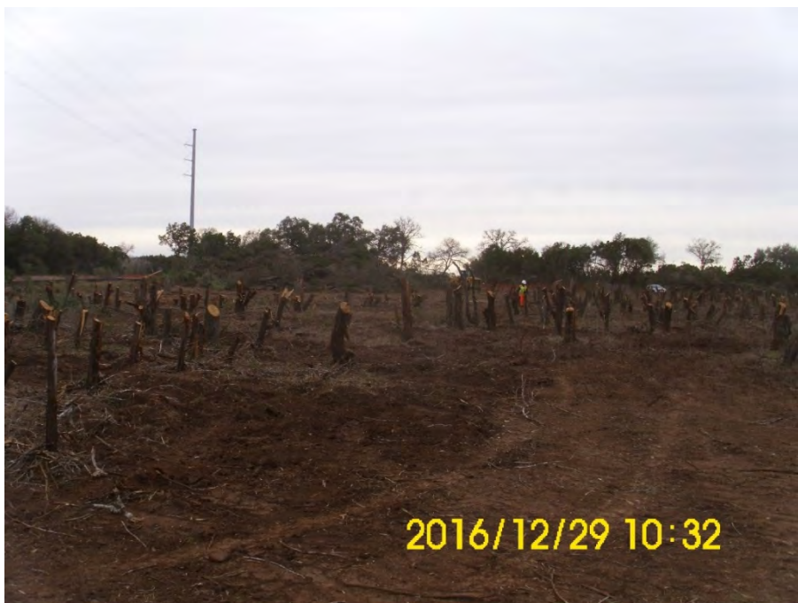
At GS2: Initial Clearing East of Danz Creek
