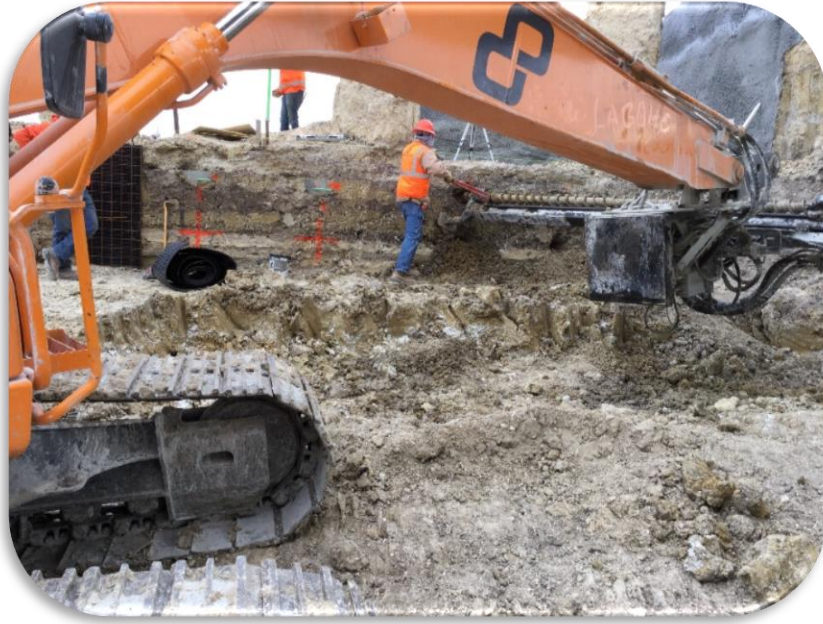
Soil Nail Wall Construction Southbound Near MLK Boulevard [December 29, 2016]
