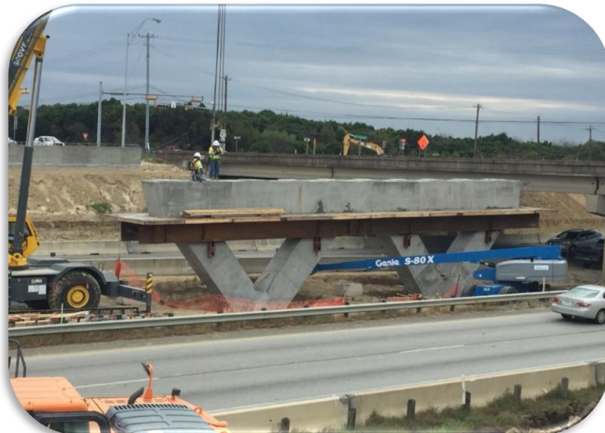
MLK Blvd U-Turn Bridge Construction
