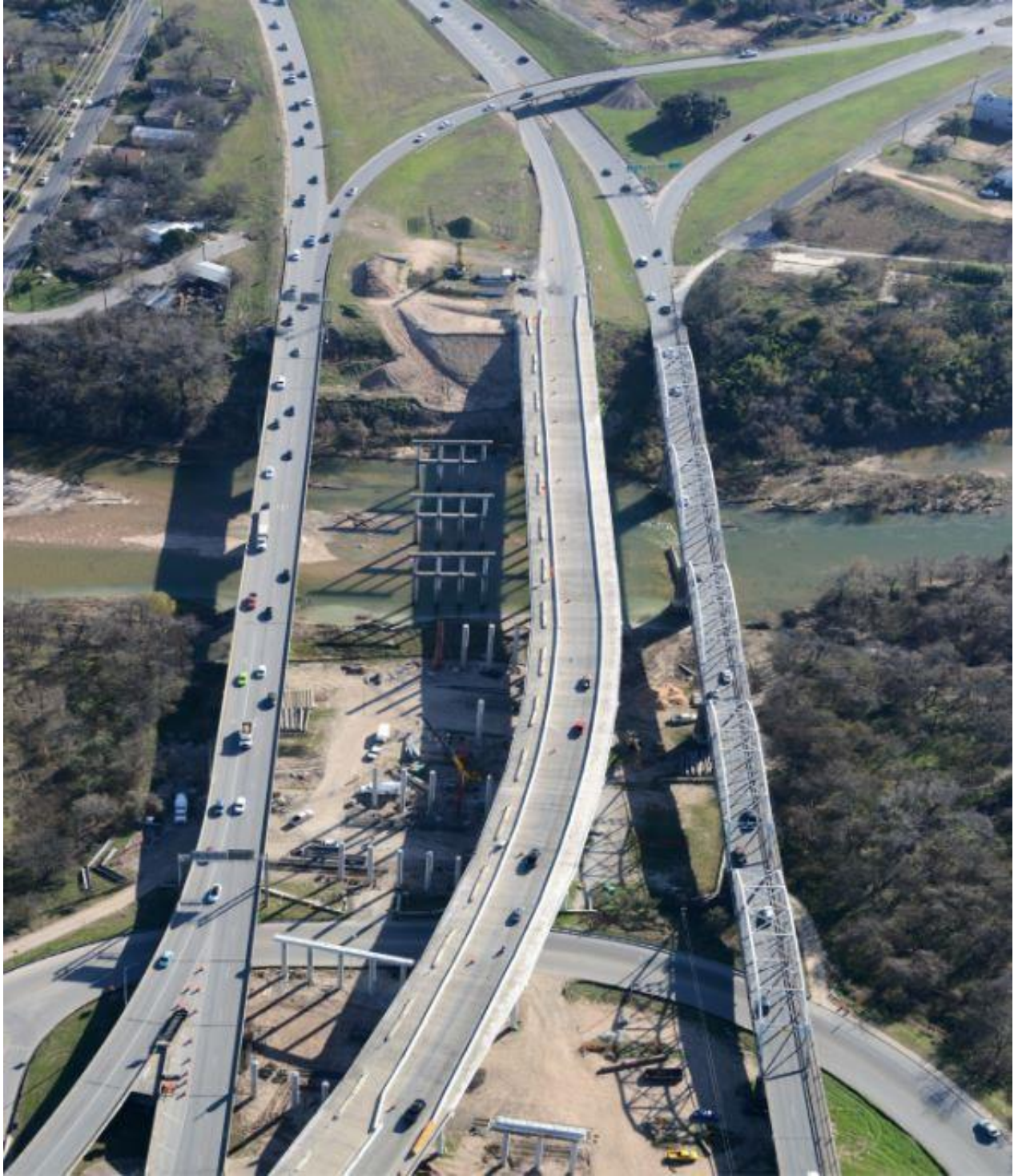
183 near Colorado River Bridge (Looking West)
