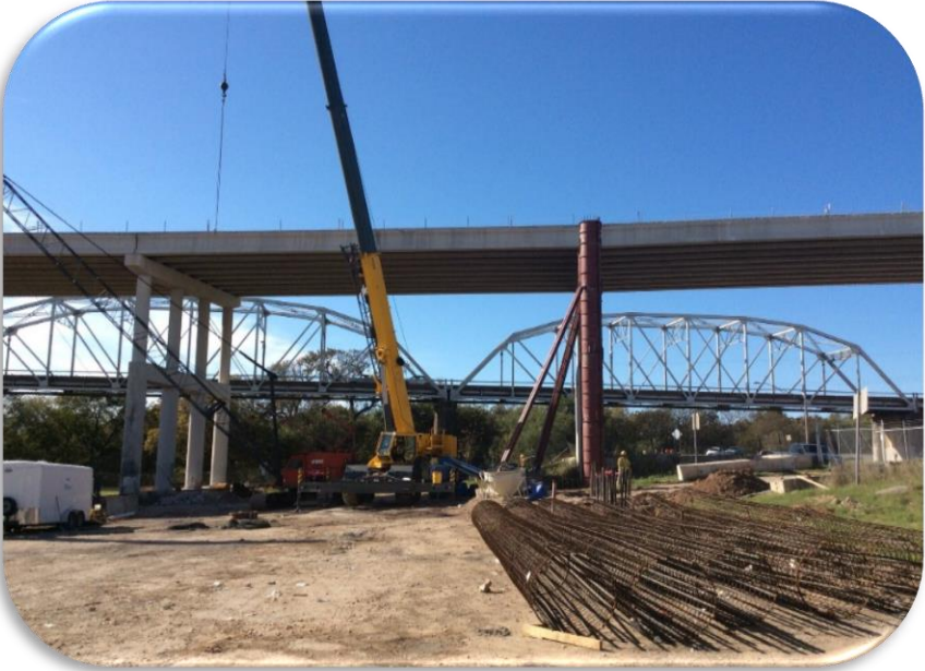
Colorado River Bridge Work [December 1, 2016]
