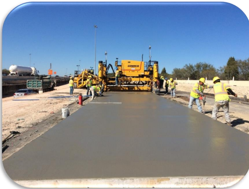
Roadway Paving Northbound Main Lanes Beginning of Project to Manor/Springdale Road
