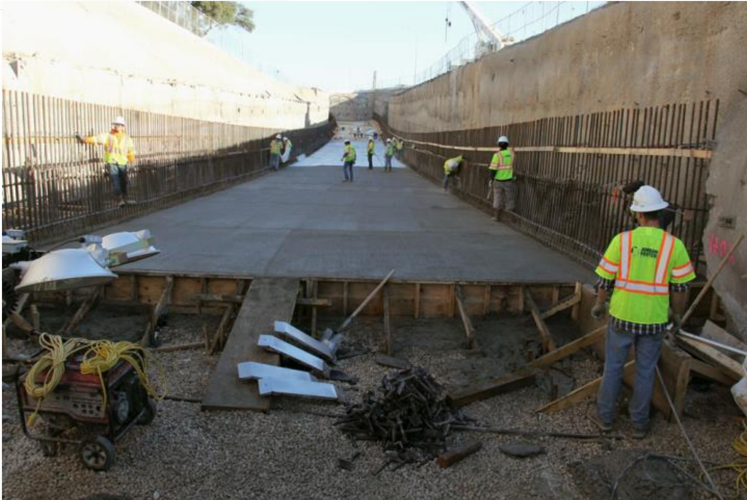
Paving at the Southbound Express Lane Underpass – January 2015
