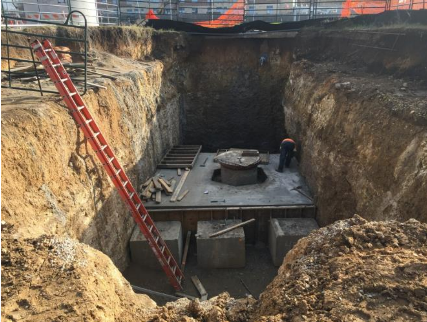
Boring for 42” Waterline at Camp Mabry – December 2015
