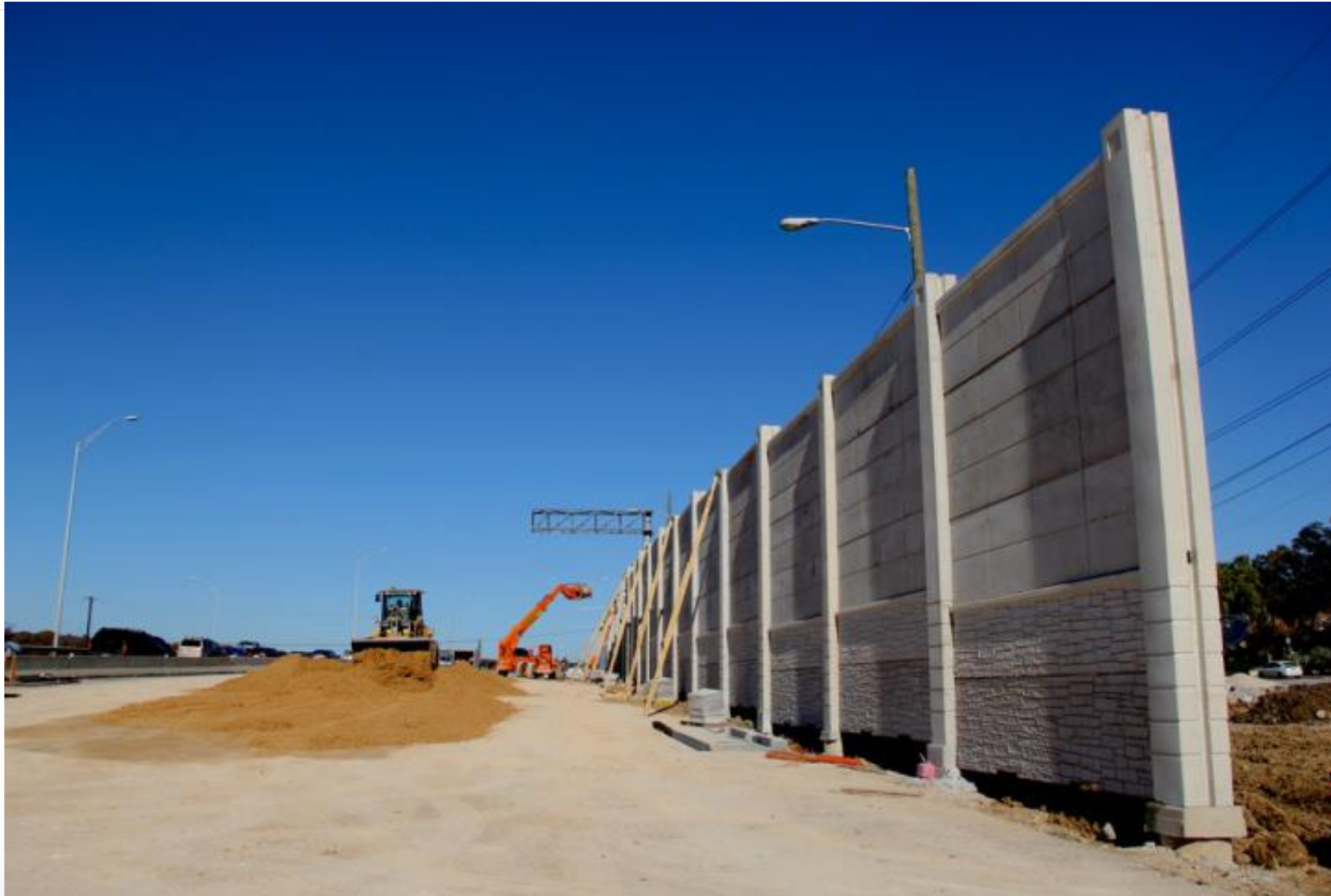
Sound Wall Construction Along Newfield Lane – December 2015
