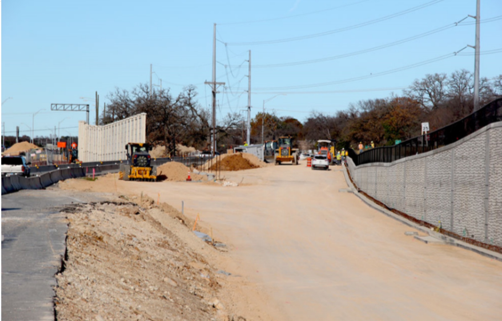
Roadway Construction for Northbound Traffic Shift – December 2015
