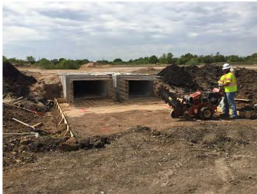
Crews working on cross drainage culverts
