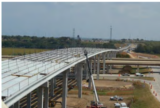
Bridge deck forming completed over SH 130
