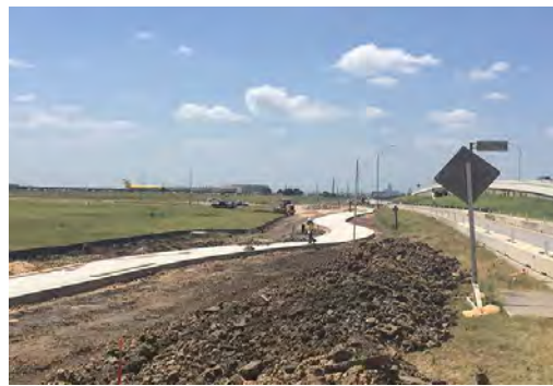
Shared use path being installed
