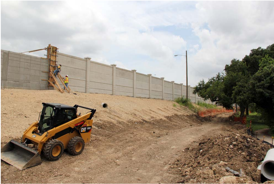
Sound Wall Construction near Enfield Road and Johnson Creek Trail
