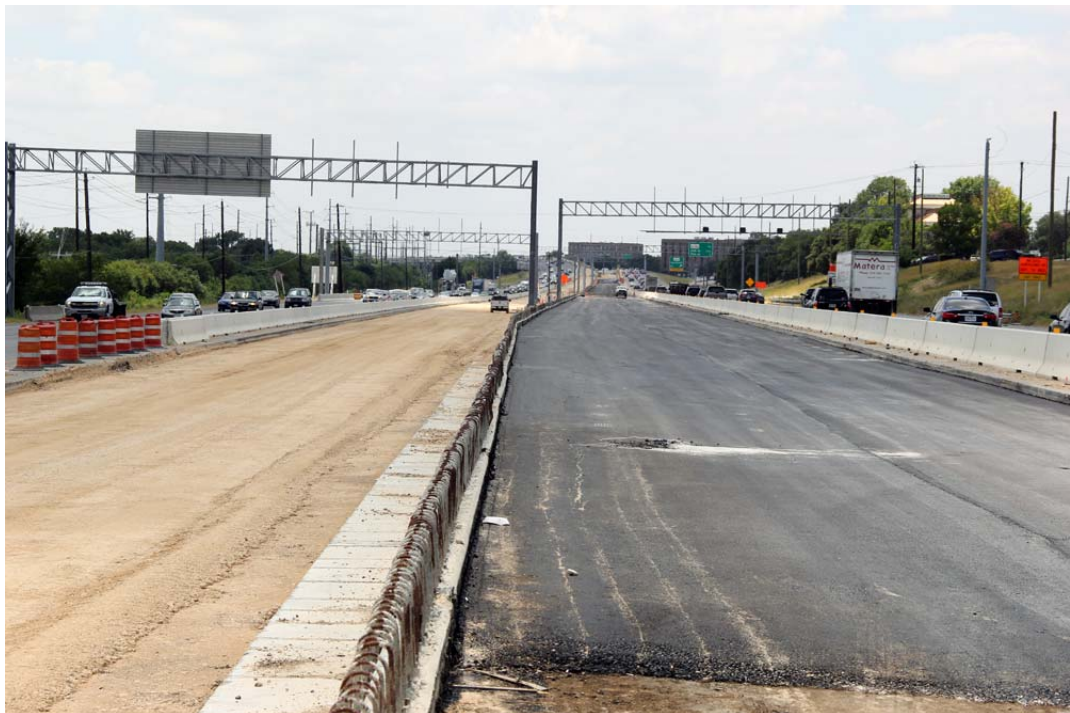
Paving of Southbound Express Lane between Far West and RM 2222
