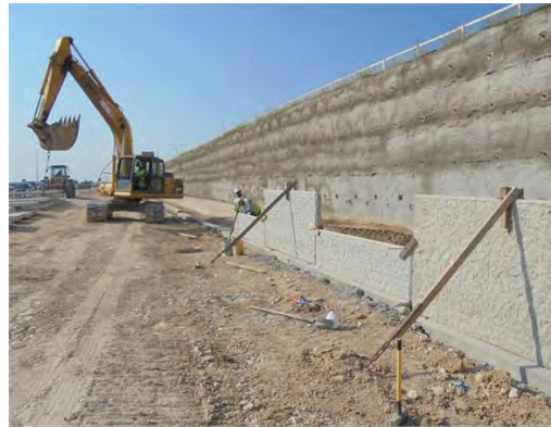
Crews installing retaining walls
