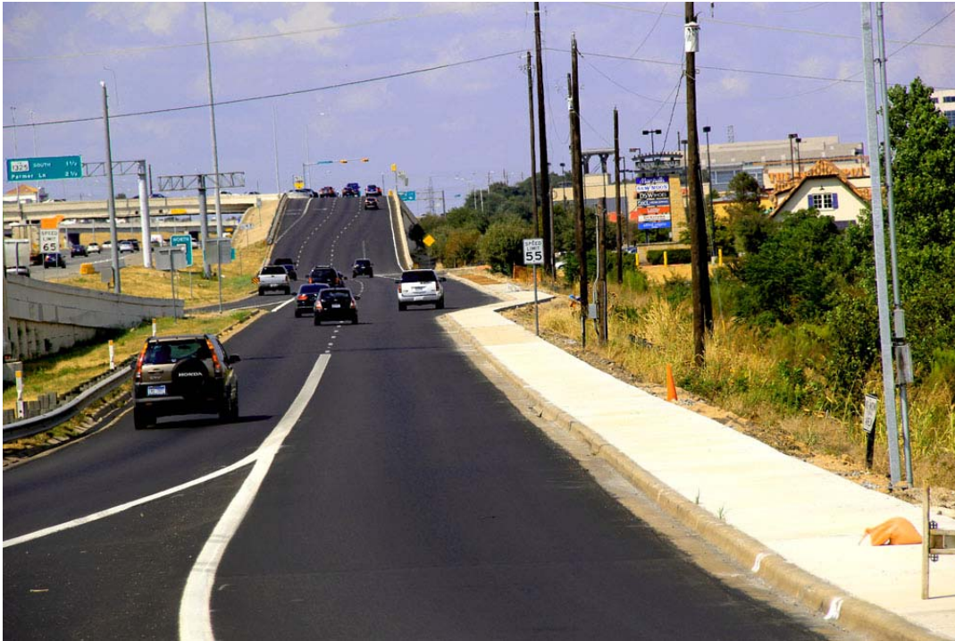
Sidewalk Construction along Northbound MoPac Frontage Road
