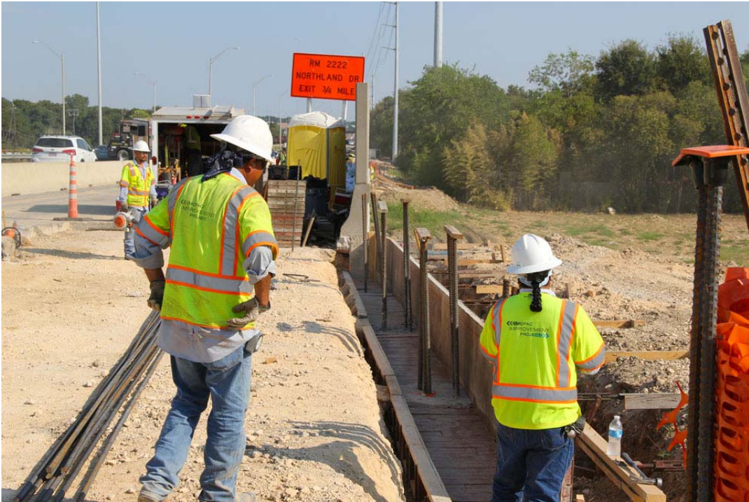
Sound Wall Foundation Work at 45 th Street
