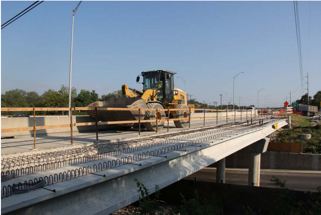
Expansion of Northbound Bridge over Windsor Road
