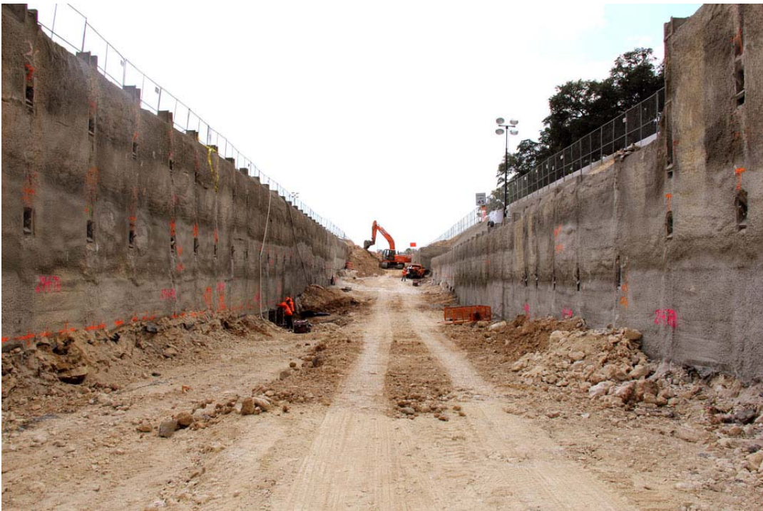
Southbound Underpass Excavation
