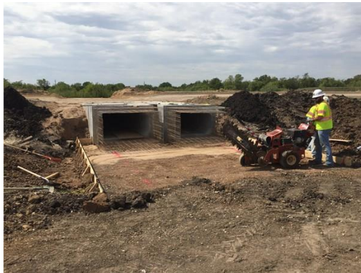
Crews working on cross drainage culverts
