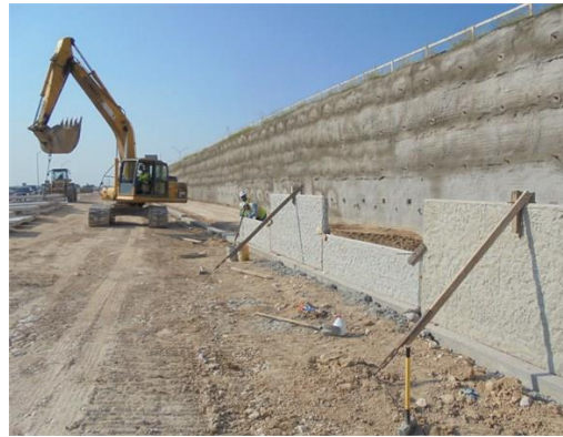
Crews installing retaining walls
