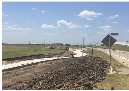
Shared use path being installed
