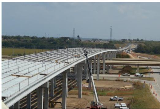
Bridge deck forming completed over SH 130
