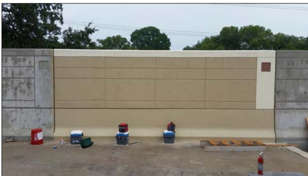
An example section of sound wall along the along MoPac Expressway.
