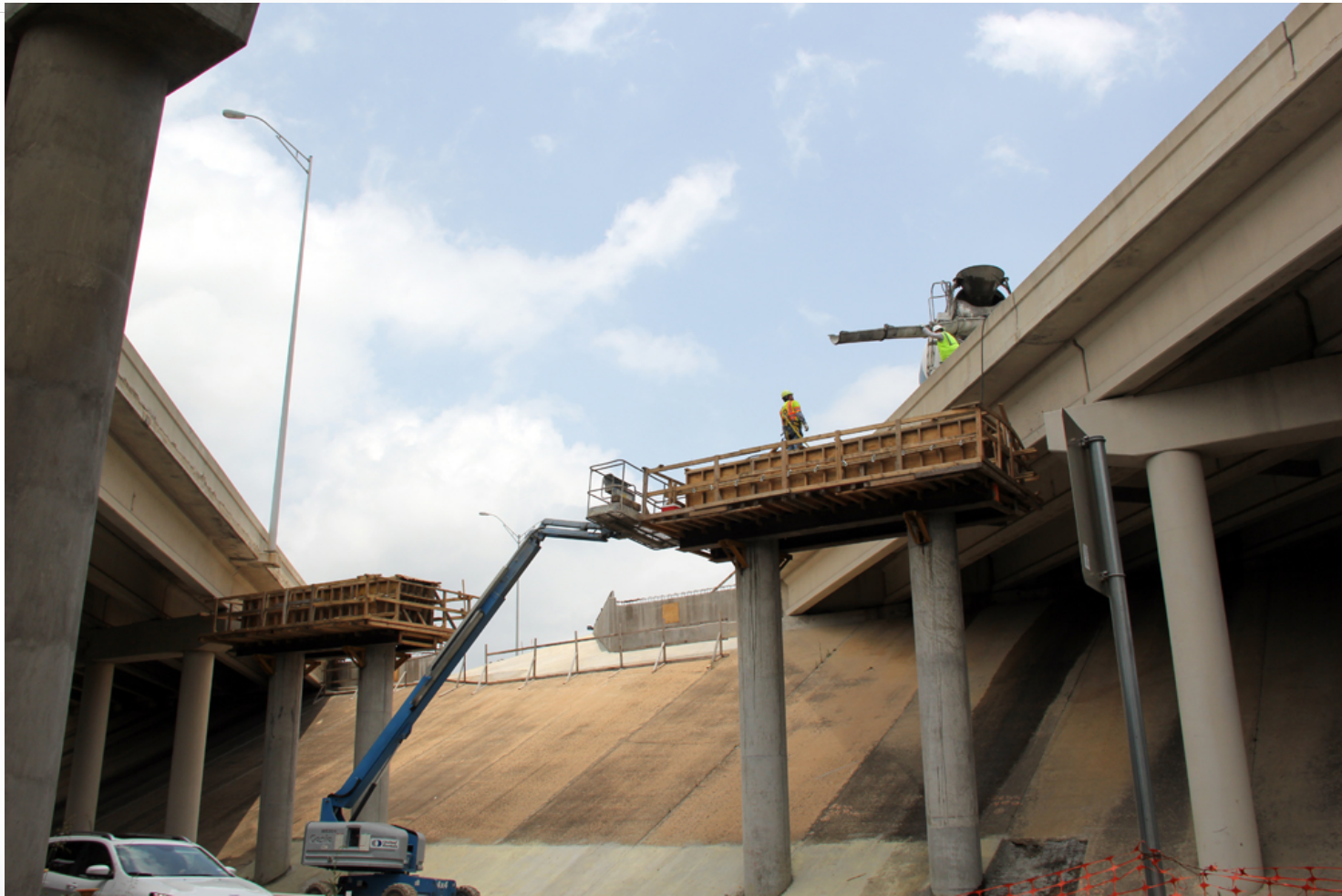
Concrete Cap Pour for Bridge Bent at MoPac Crossing over UPRR
