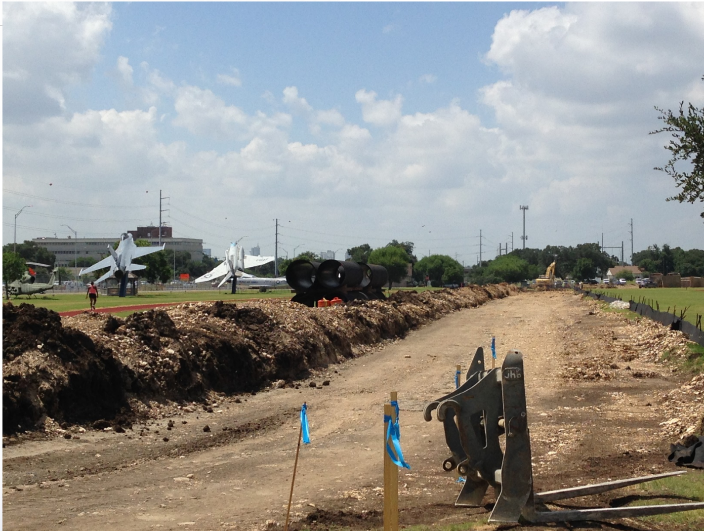
42-inch Waterline Trench – Camp Mabry
