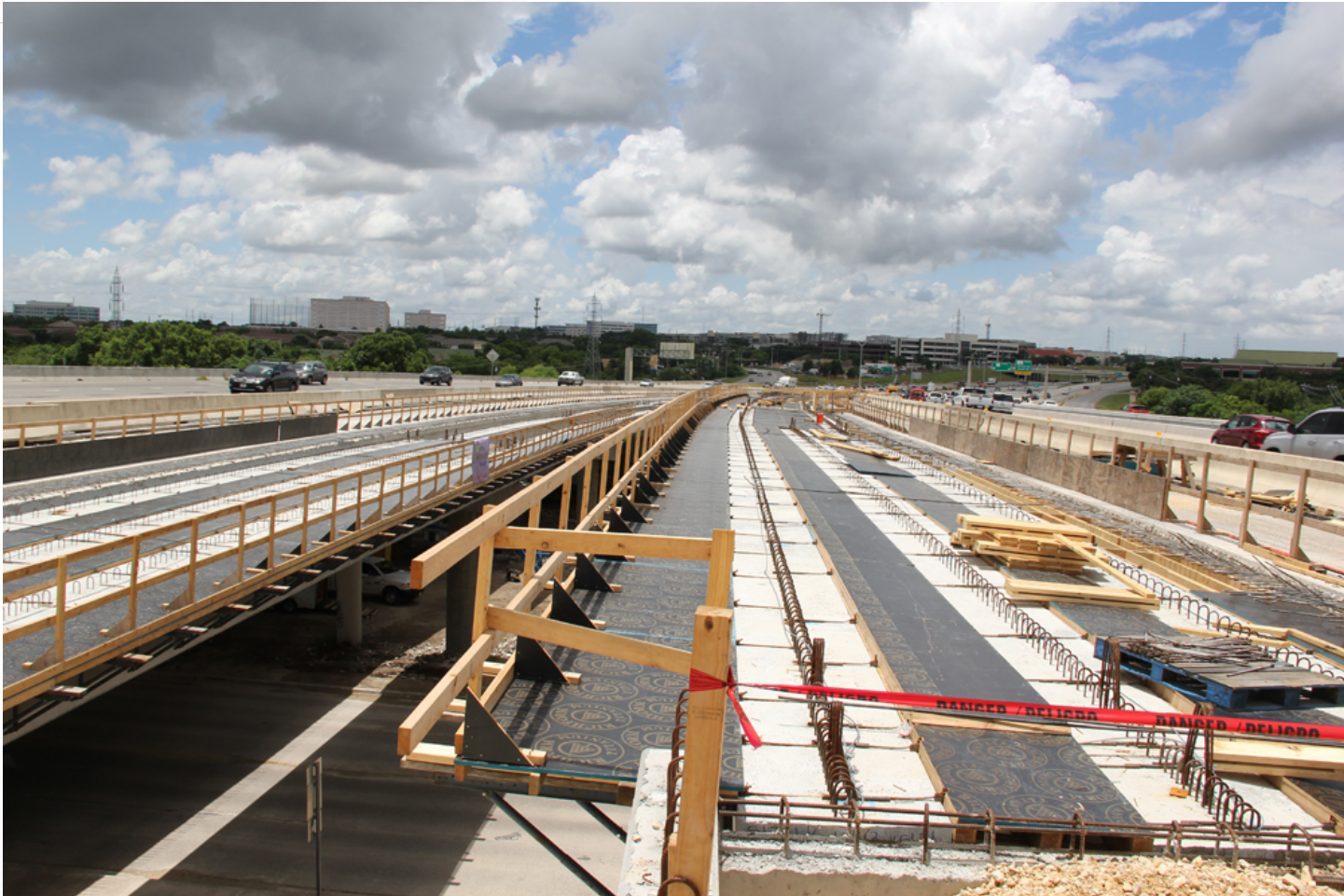
Deck Forms for Southbound MoPac Bridge over Capital Metro Red Line
