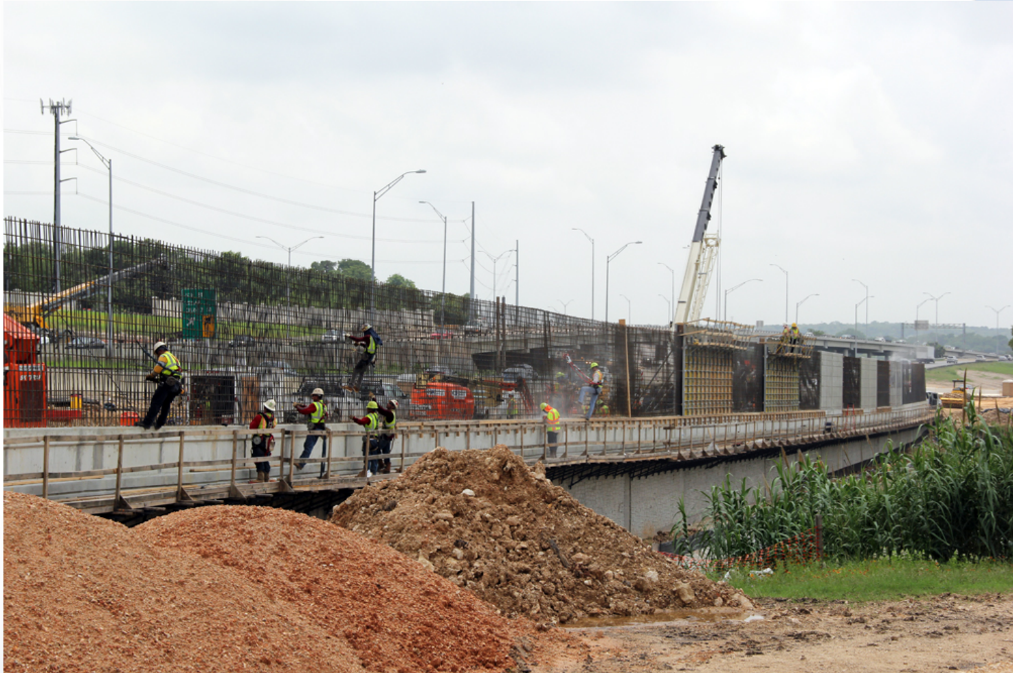
Sound Wall Construction along Southbound MoPac
