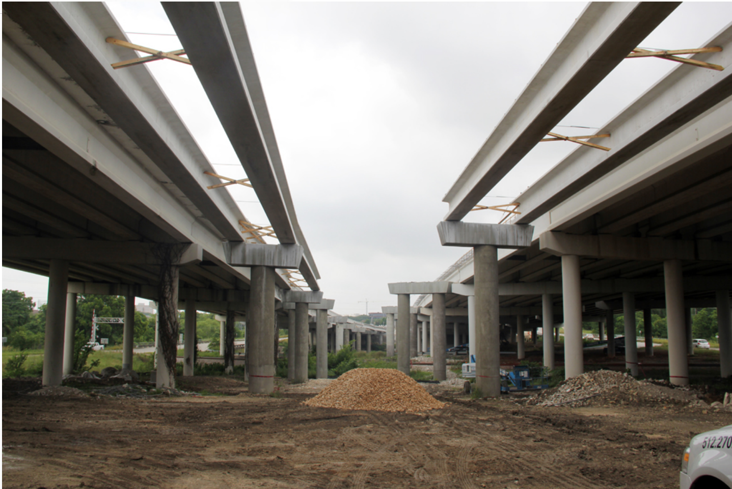
Beams set for MoPac Bridge Over Waters Park Road
