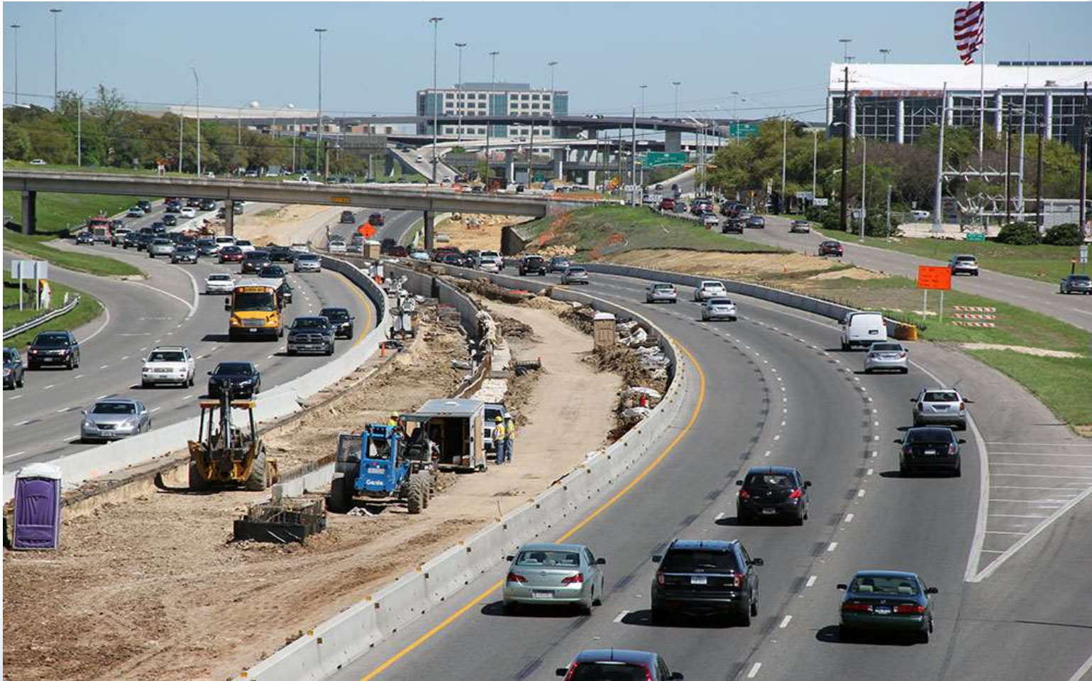
Retaining Wall and Flex Base Pavement Preparation at Steck Avenue
