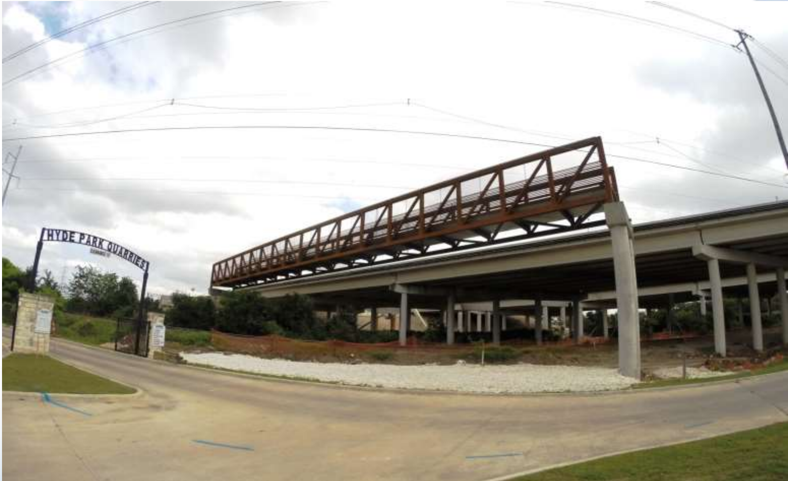
Bicycle and Pedestrian Bridge Segment In Place over UPRR
