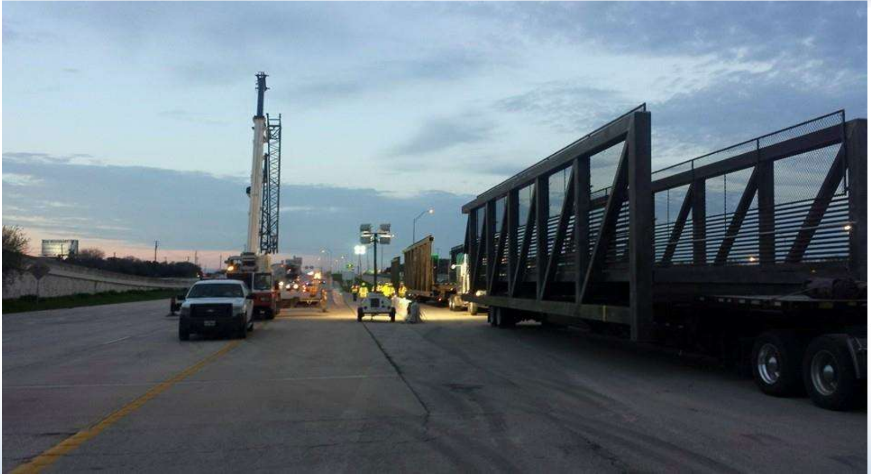
Bicycle and Pedestrian Bridge Segment Final Assembly
