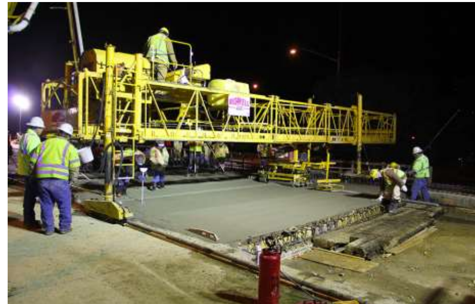
Pouring Concrete Bridge Deck
