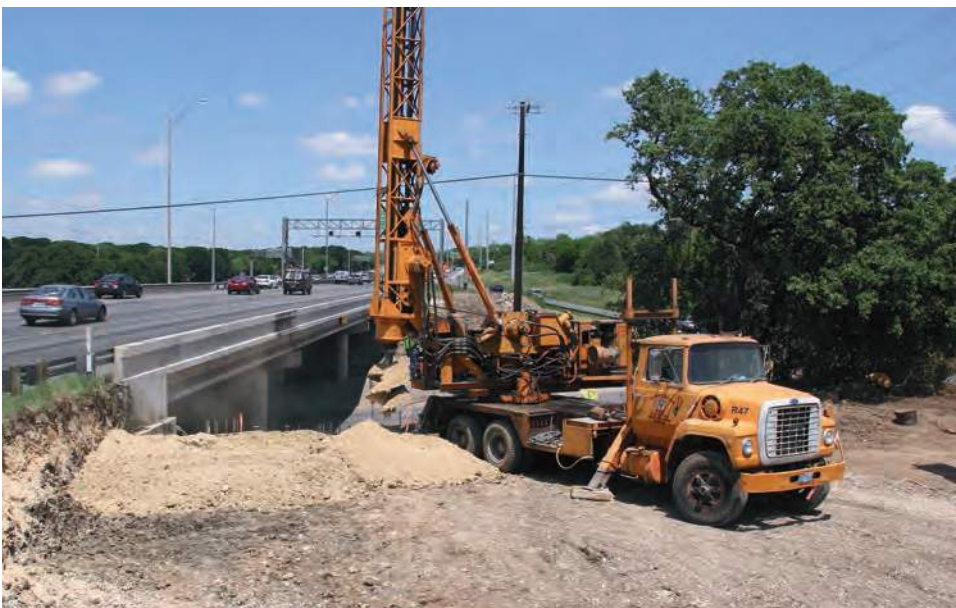
Construction of the MoPac Express Lanes
