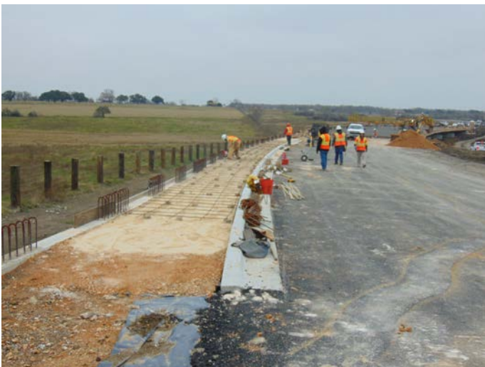
Maha Loop Construction
