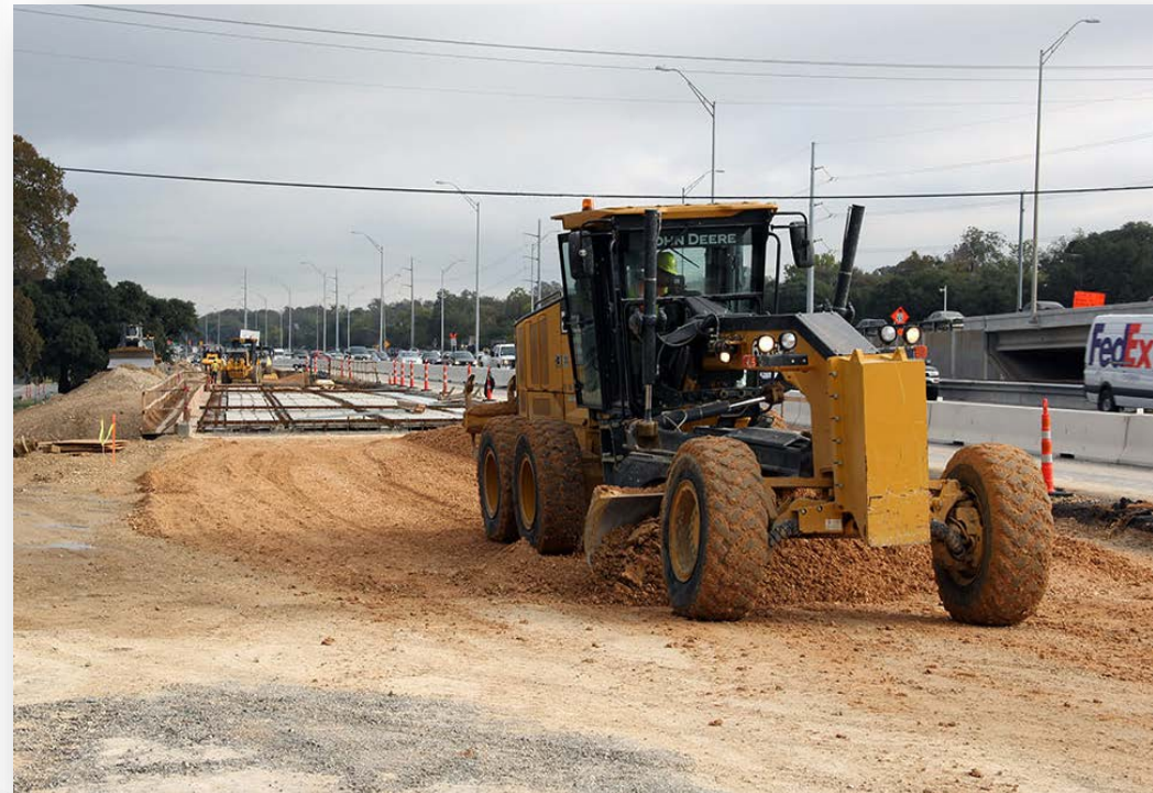
Grading Base Material for MoPac Roadway Widening at Enfield Road
