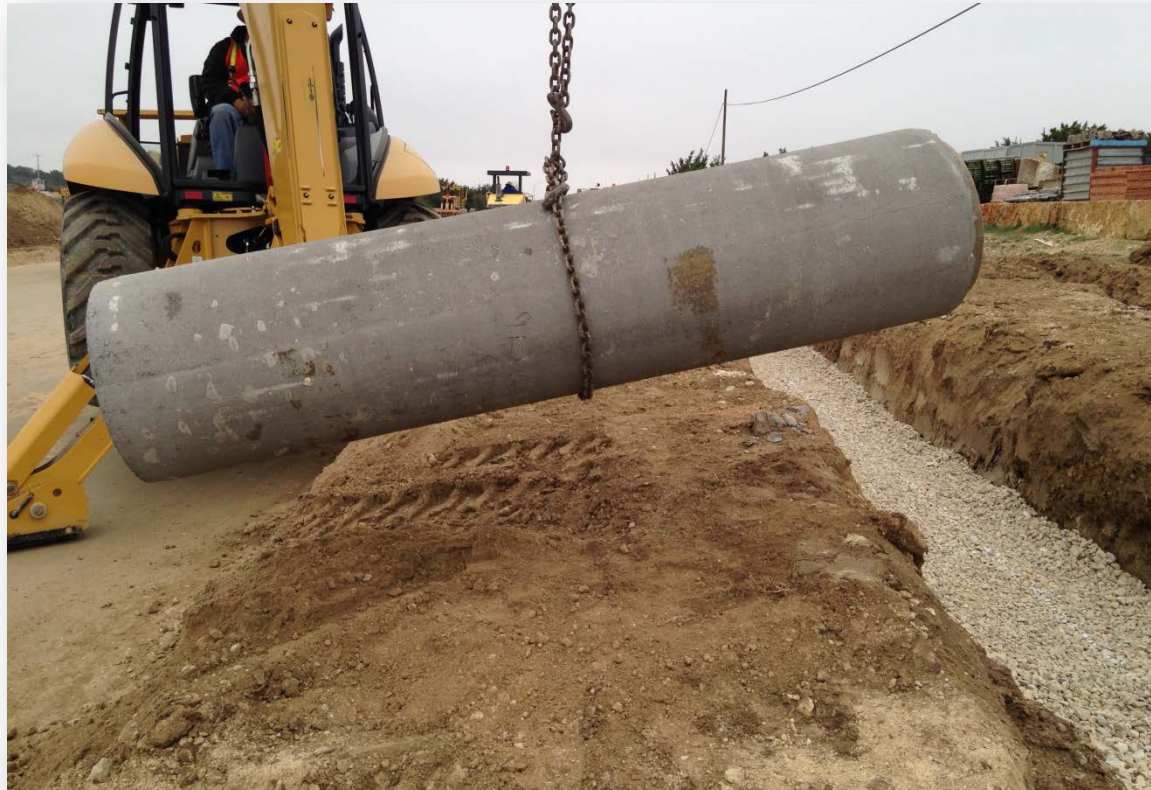
Driveway Culvert Installation
