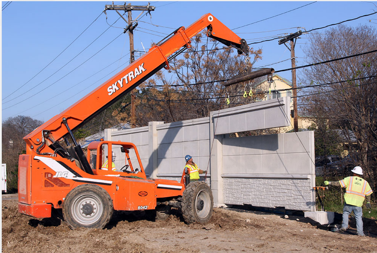
First Sound Wall Installation along Newfield Lane Jan. 7, 2015
