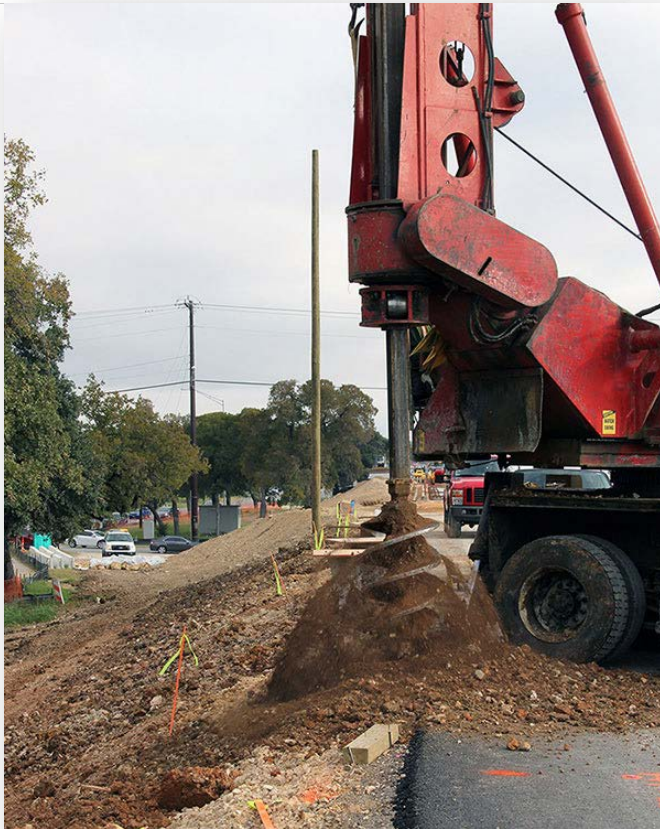
Drilling Shaft for Soundwall Foundation South of Enfield Road
