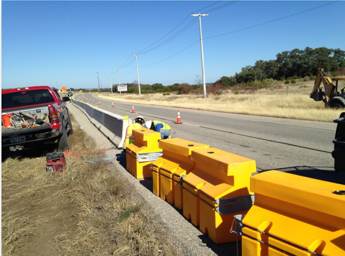
Installation of Portable Concrete Traffic Barrier
