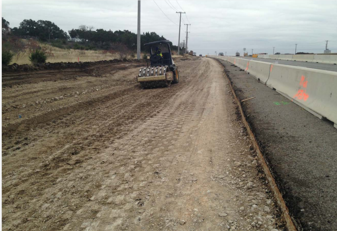
Road Widening For Deceleration Lane to Bryson Ridge Trial Roadway
