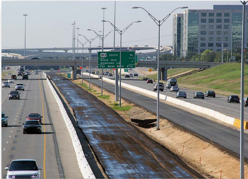
Paving Express Lanes near Braker Lane
