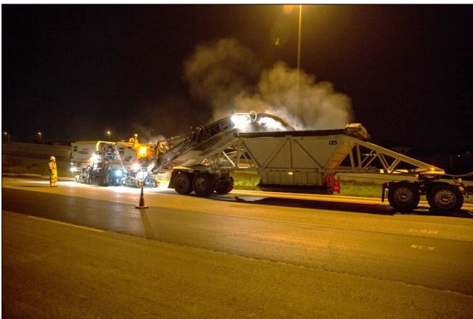
Mill and Overlay crew on 183A
