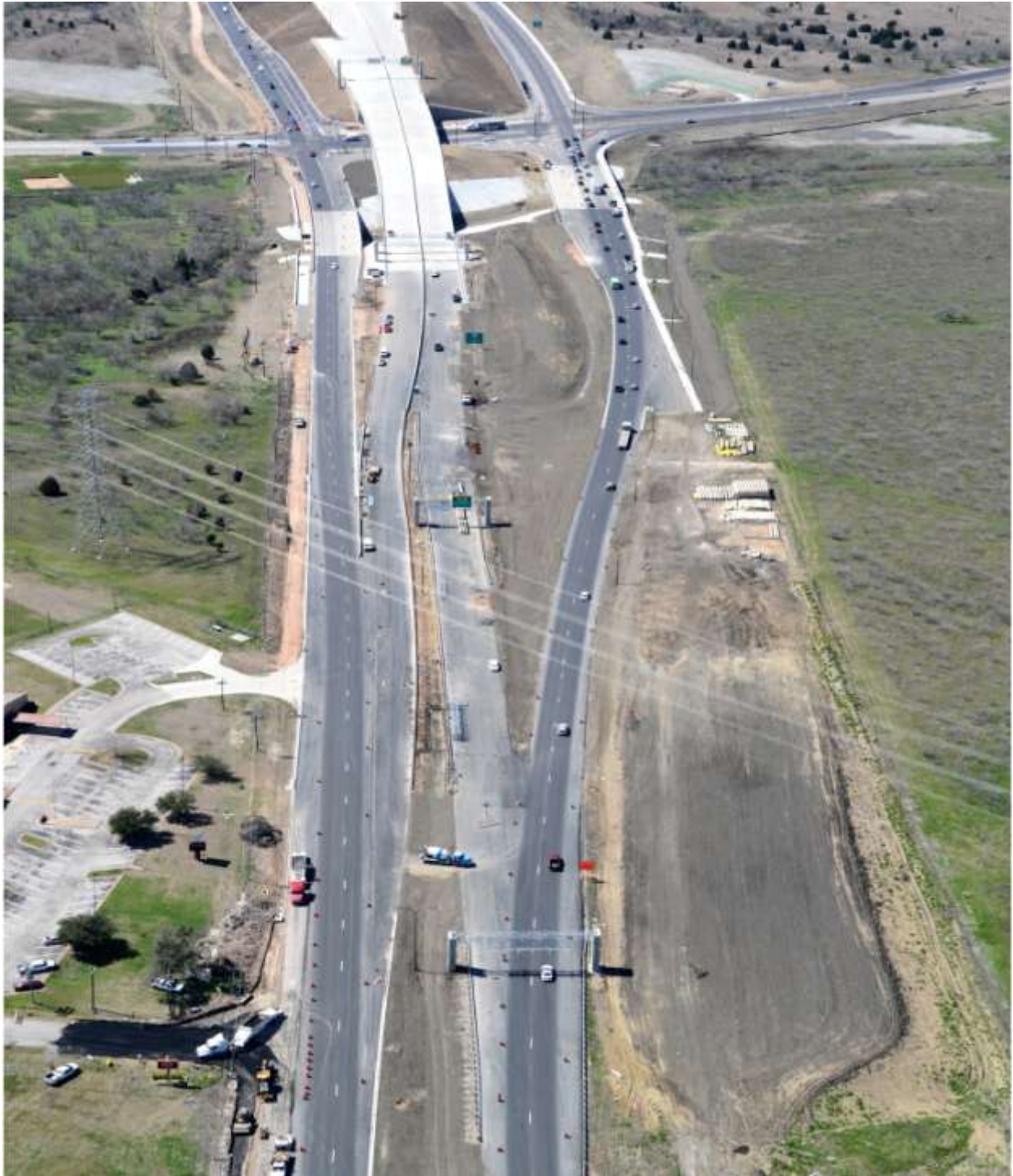
US 290 East looking west from Gilleland Creek (Taken 3/11/2014)
