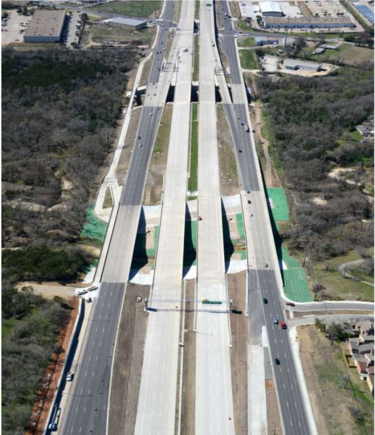
US 290 East at Chimney Hill Blvd looking west (Taken 3/11/2014)
