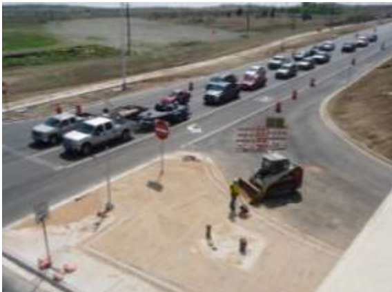
Crews install hardscaping at the Parmer Lane intersection (Looking Northeast)
