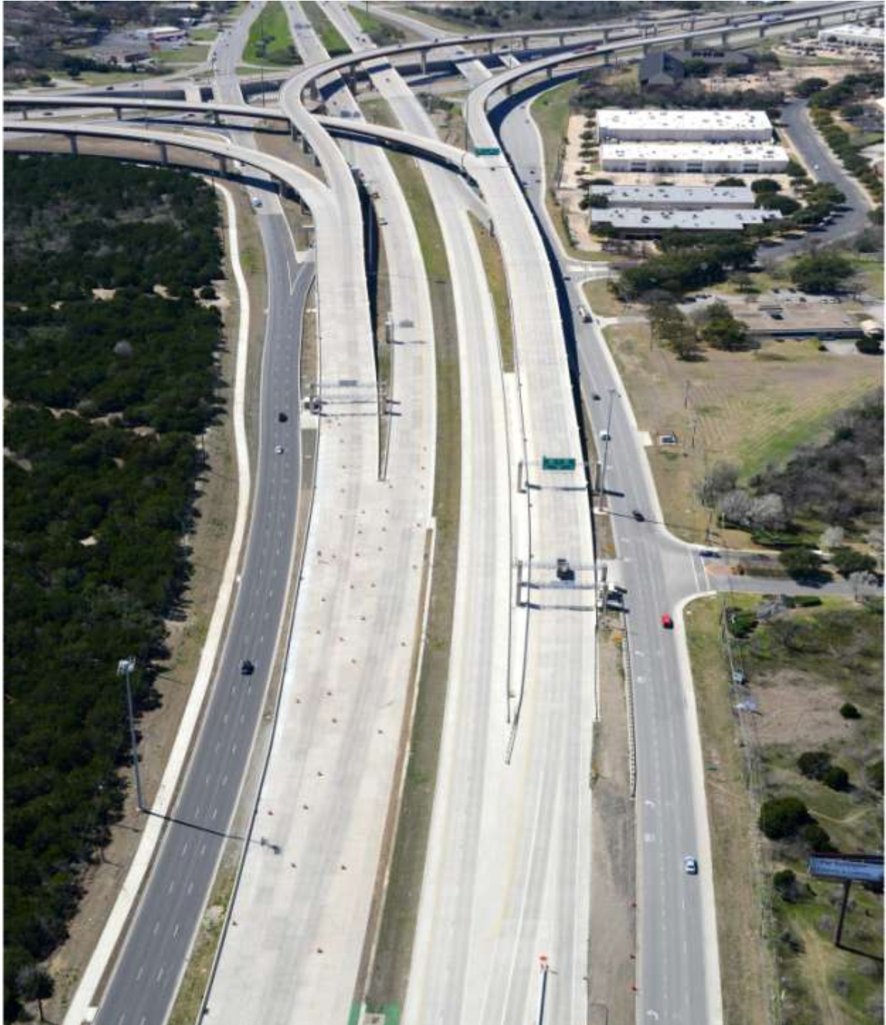
US 290 East at Ridgepoint Drive looking west (Taken 3/11/2014)
