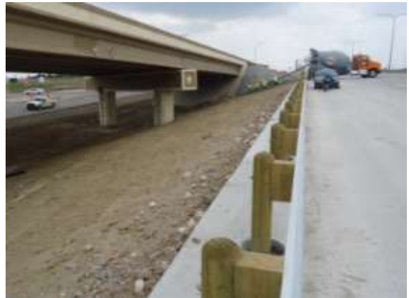
Crews pour concrete riprap near SH 130 (Looking West)
