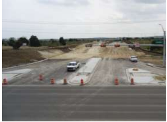
CTMC constructs the connection to the relocated FM 3177 (Looking South)
