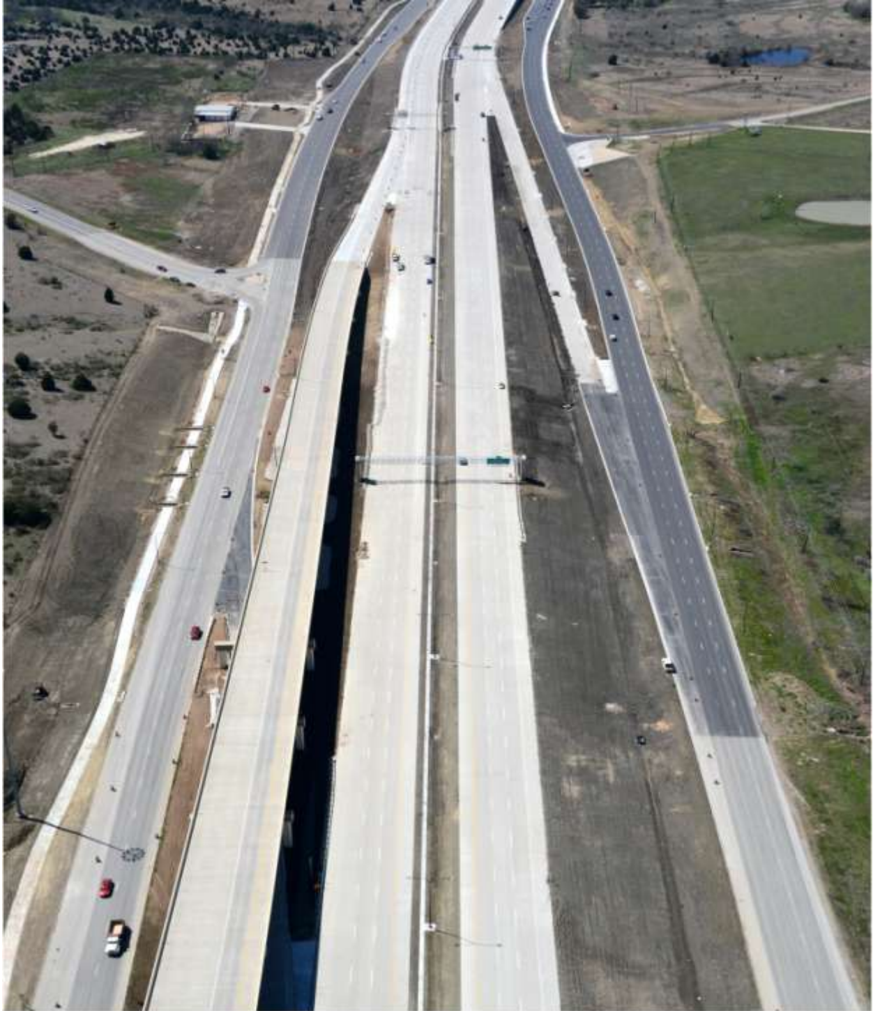
US 290 East at Decker Lane Intersection looking west (Taken 3/11/2014)
