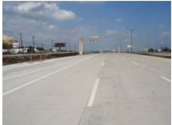
Westbound mainlanes west of Giles Road (Looking East)
