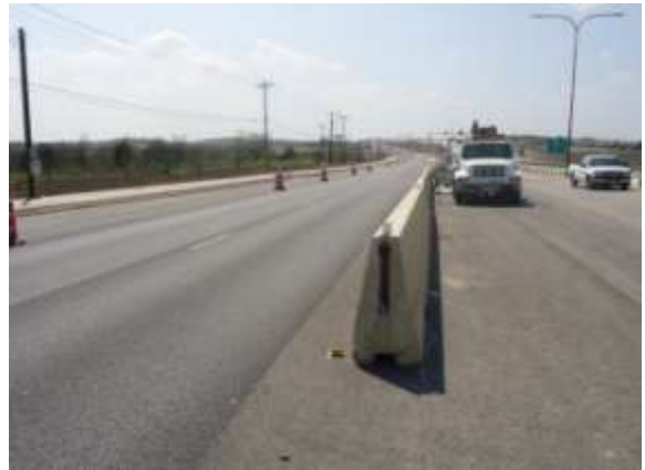
CTMC works on the revised eastern project terminus (Looking West)
