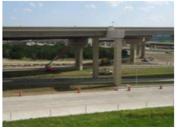
Crews paint the column caps at the US 183 interchange (Looking South)
