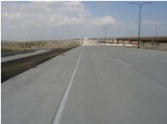
Westbound mainlanes west of SH 130 (Looking East)
