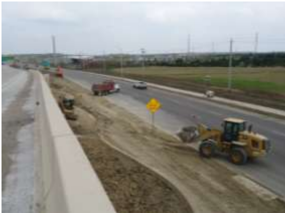
Crews install landscaping beds along the mainlanes east of Giles Road (Looking East)
