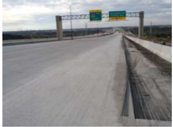
Concrete paving east of the Arterial "A" intersection (Looking West)
