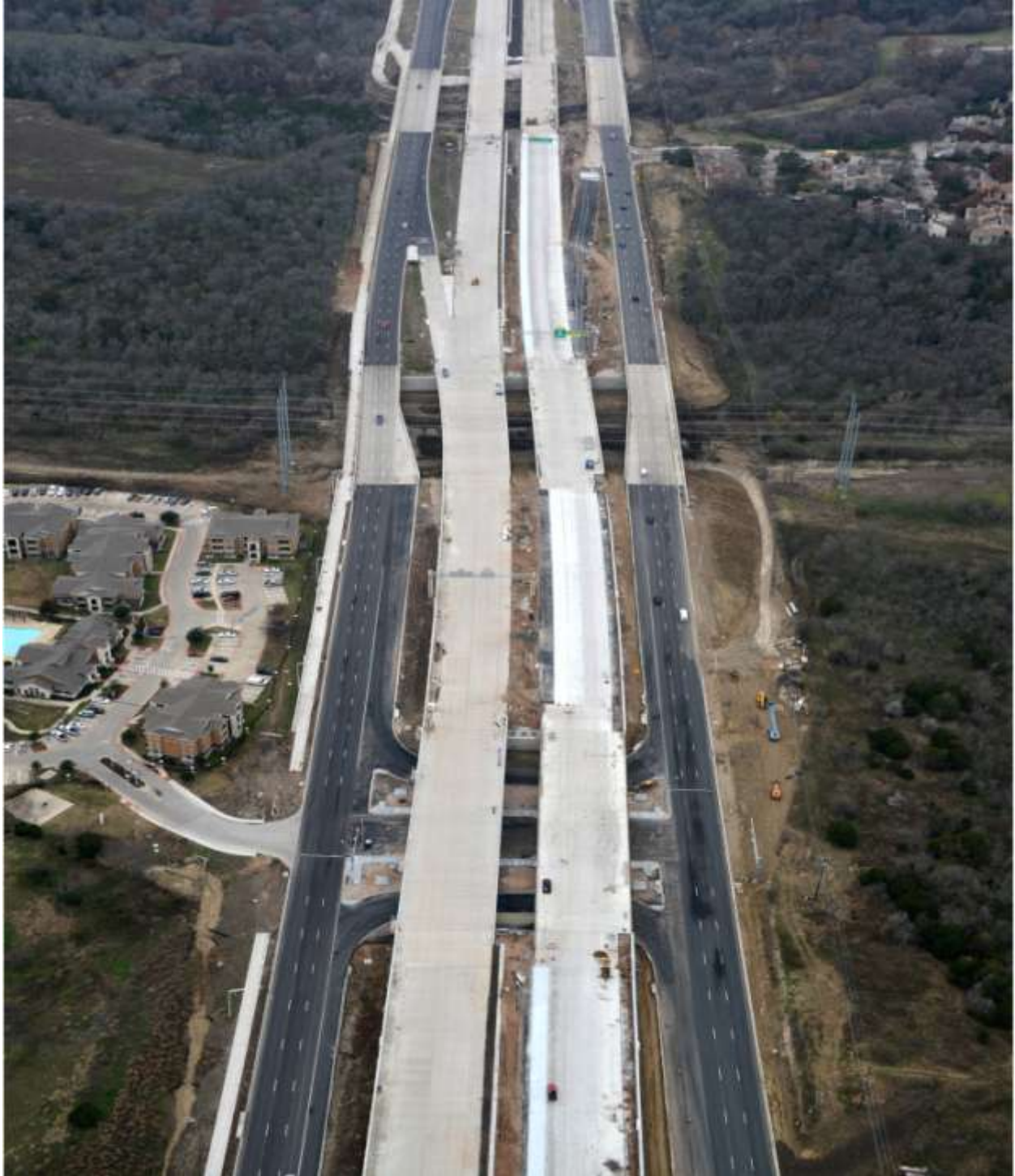
US 290 East looking west at the MOKAN Crossing (Taken 12/16/2013)
