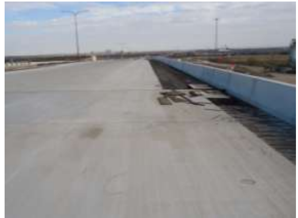
Concrete paving east of the SH 130 interchange (Looking East)
