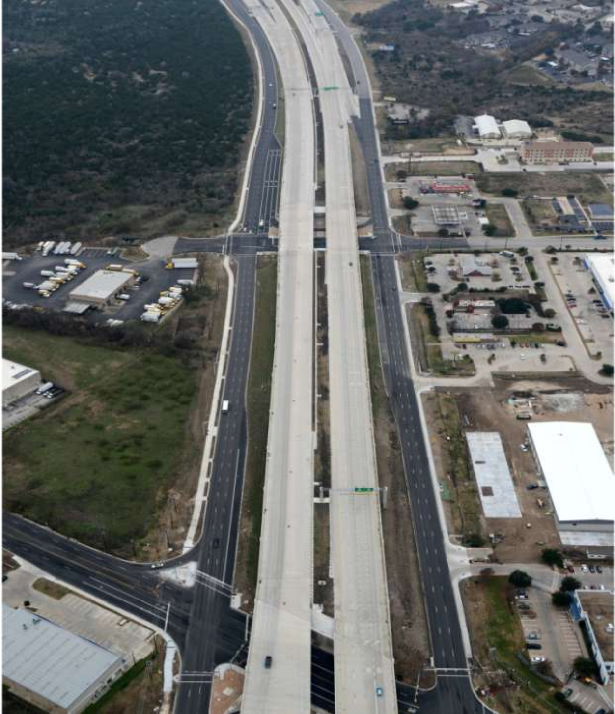
US 290 East at Springdale Road looking west (Taken 12/16/2013)
