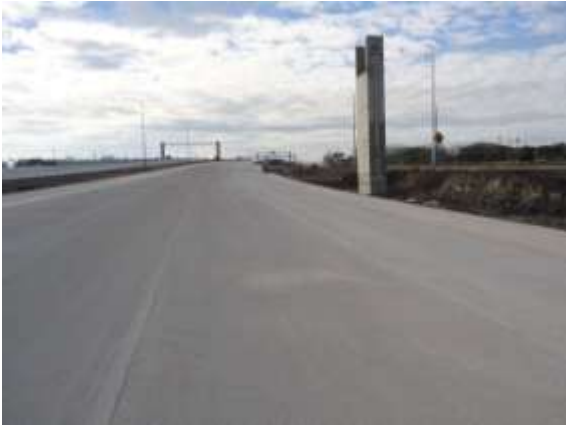
Concrete paving east of the Giles Road intersection (Looking West)
