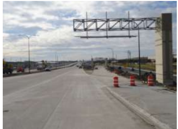
The overhead sign structure west of Harris Branch Parkway (Looking West)
