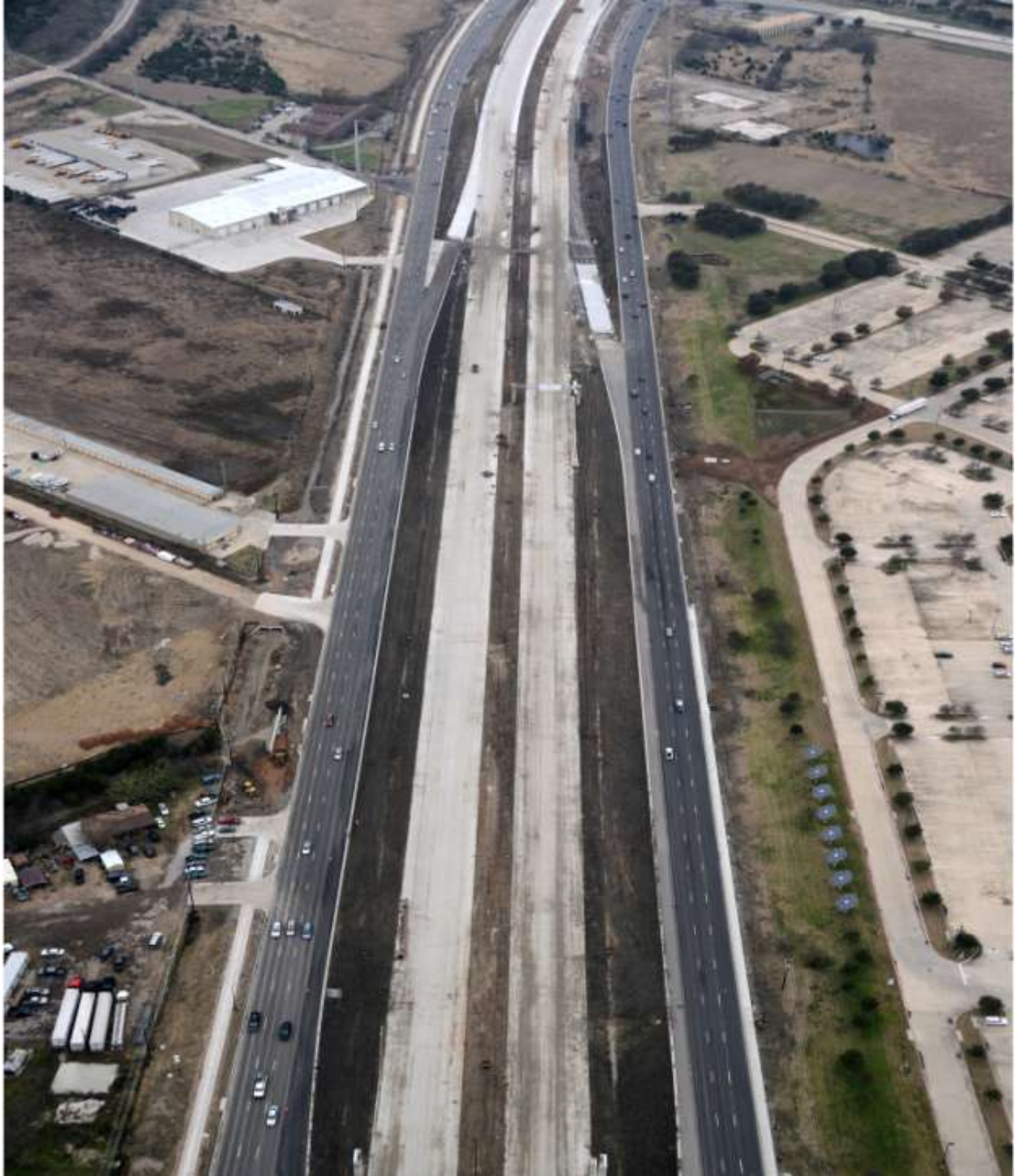
US 290 East at Crofford Lane Intersection looking west (Taken 12/16/2013)
