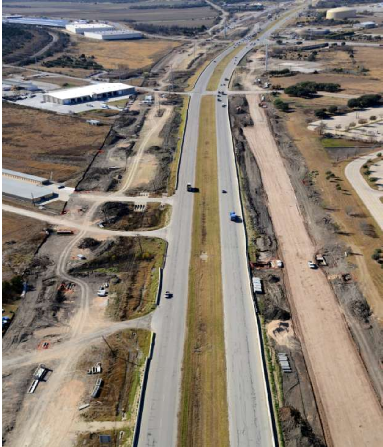
US 290 East at Crofford Lane Intersection looking west (Taken 12/18/2012)
