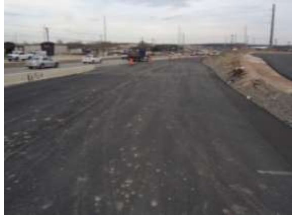
Construction of the eastbound detour west of Giles Road (Looking West)
