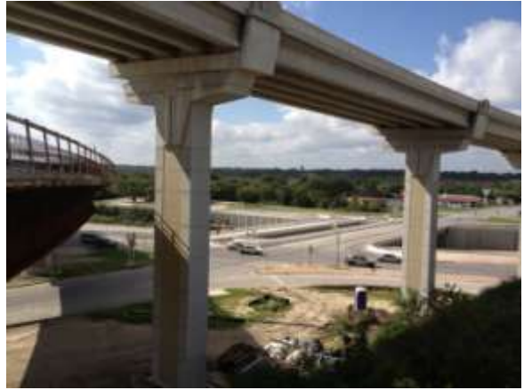
Painted columns on the south to east direct connector
