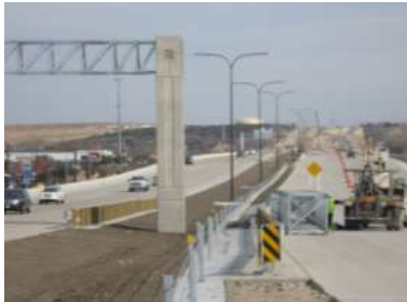
Completed eastbound and westbound mainlanes (Looking East)
