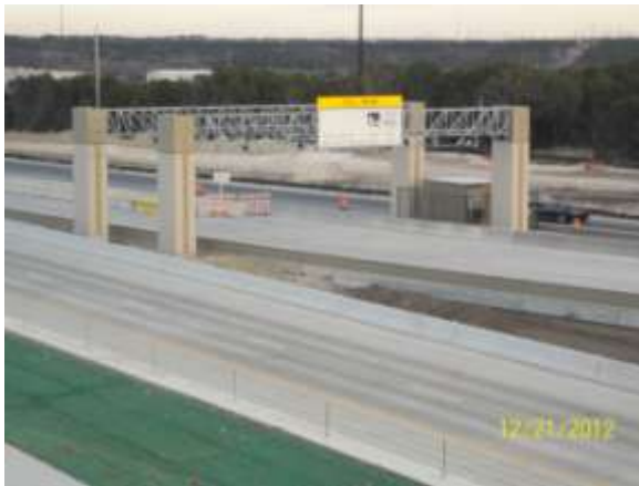
Completed South to East Toll Plaza and 290 EBML (Looking Southeast)
