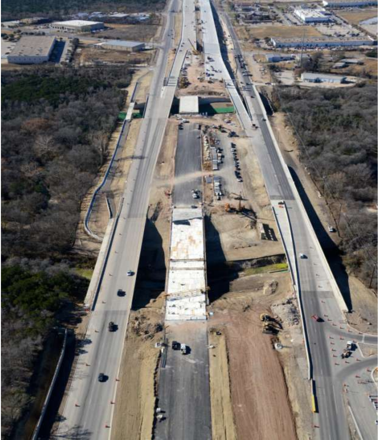
US 290 East at Chimney Hill Blvd looking west (Taken 12/18/2012)
