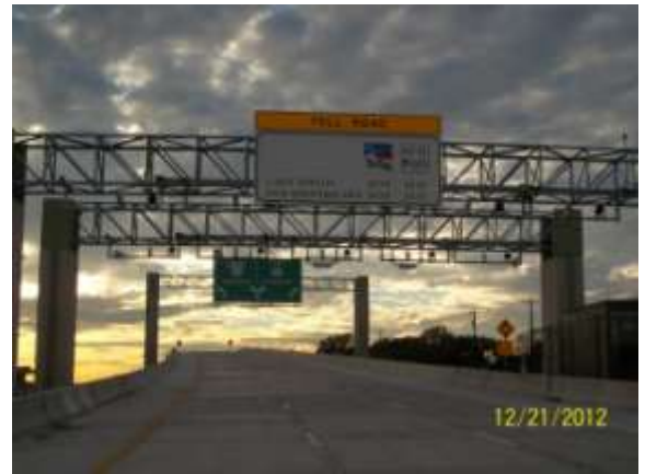
West Bound Direct Connector Approach Slab after striping (Looking West)
