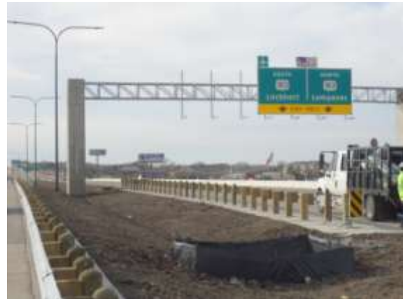
Overhead sign bridge located on the westbound mainlanes (Looking West)
