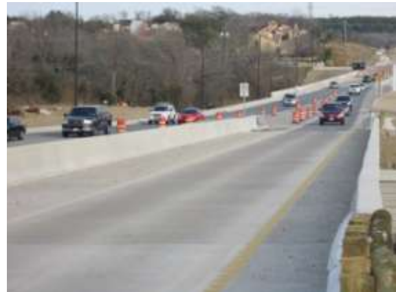
Traffic entering Ramp #3 – westbound tolling point (Looking East)
