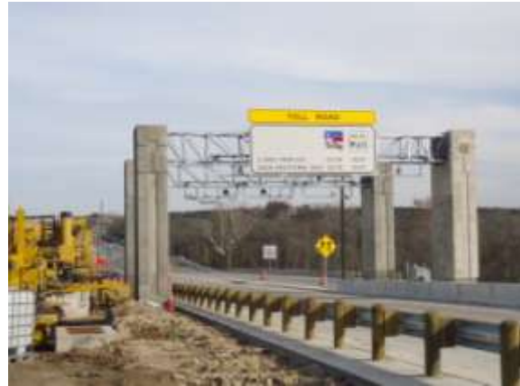
Ramp #4 Toll Gantry - eastbound tolling point (Looking East)
