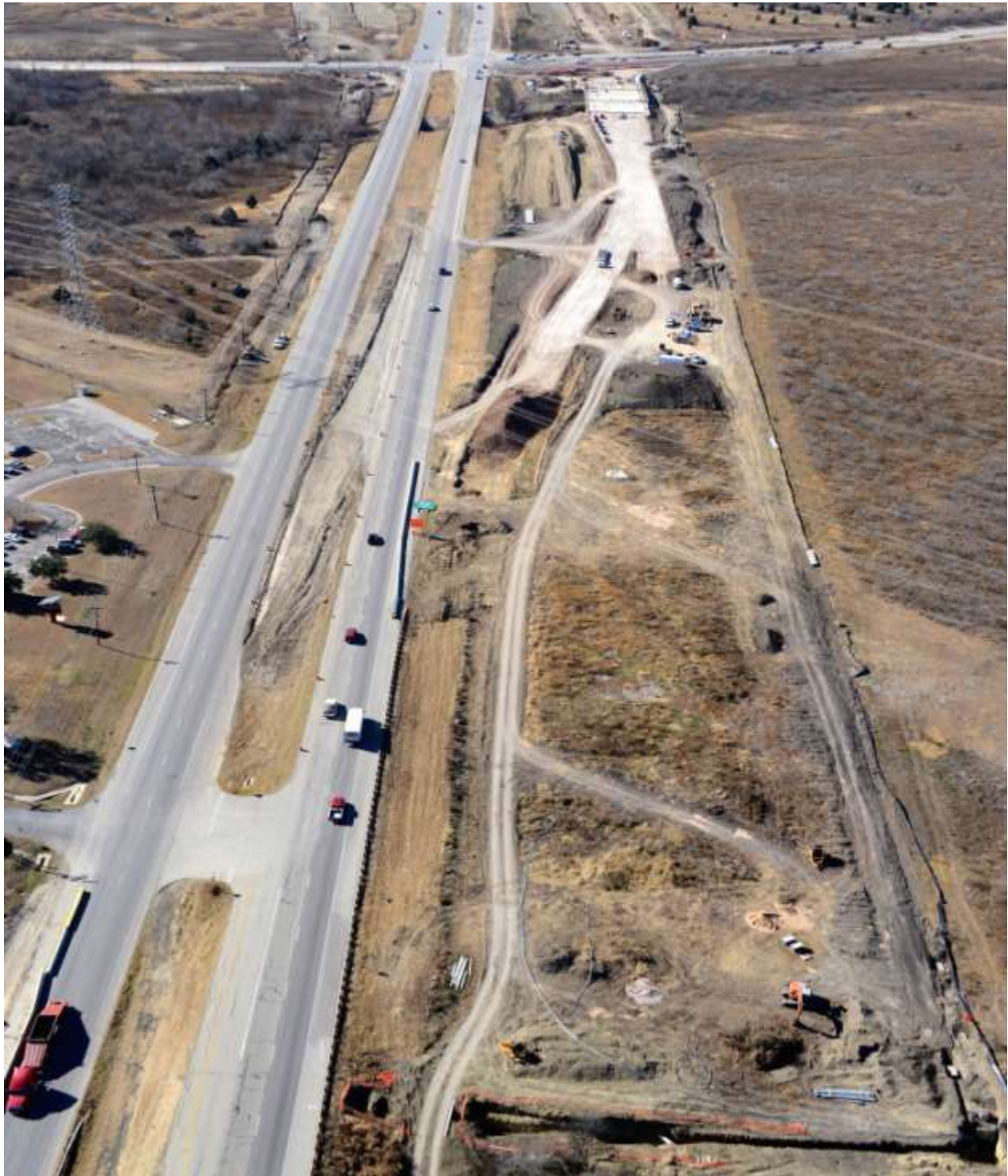
US 290 East looking west from Gilleland Creek (Taken 12/18/2012)
