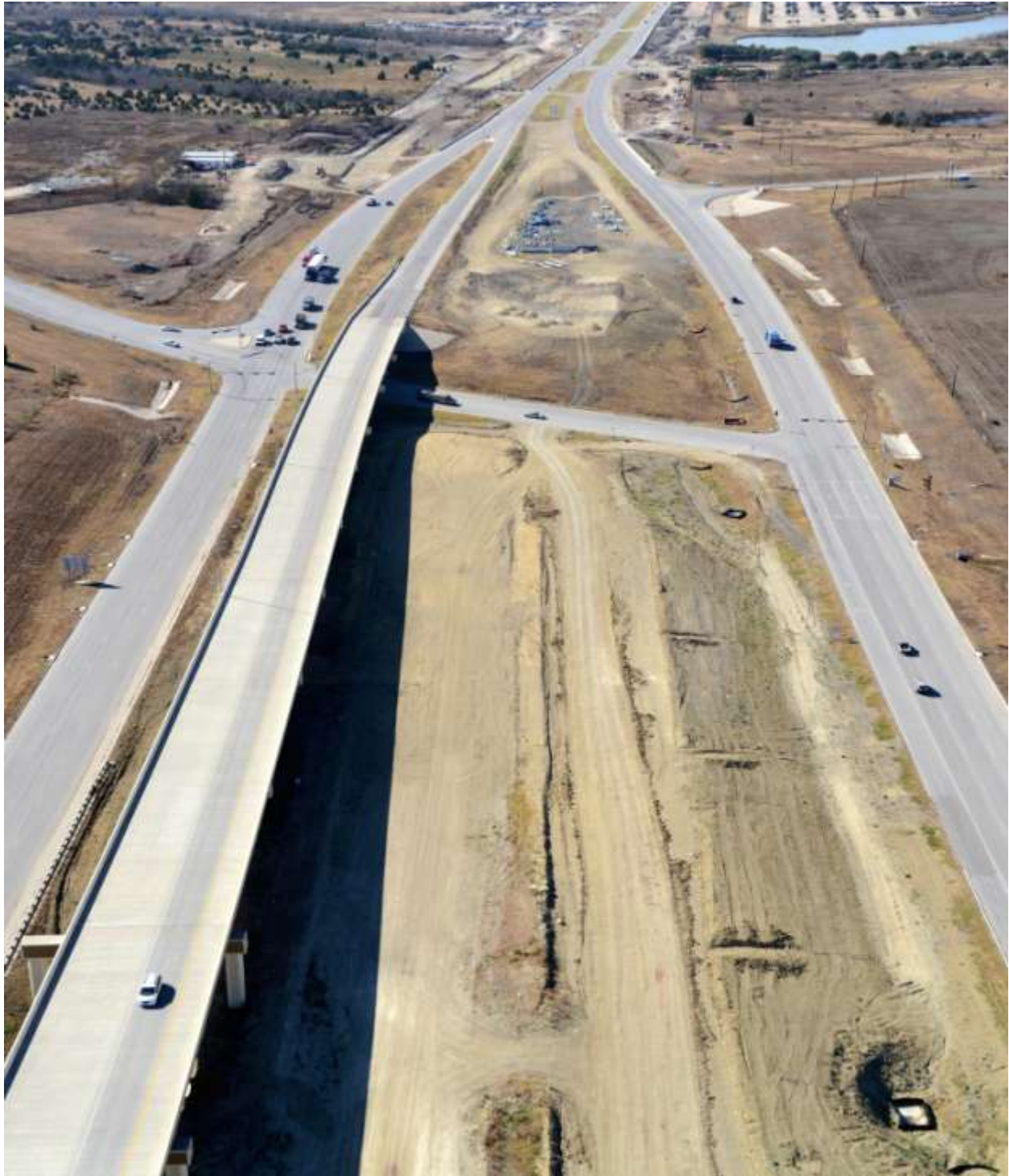
US 290 East at Decker Lane Intersection looking west (Taken 12/18/2012)
