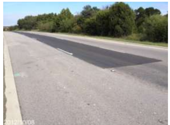
Striping on northbound US 183 frontage road (Looking North)
