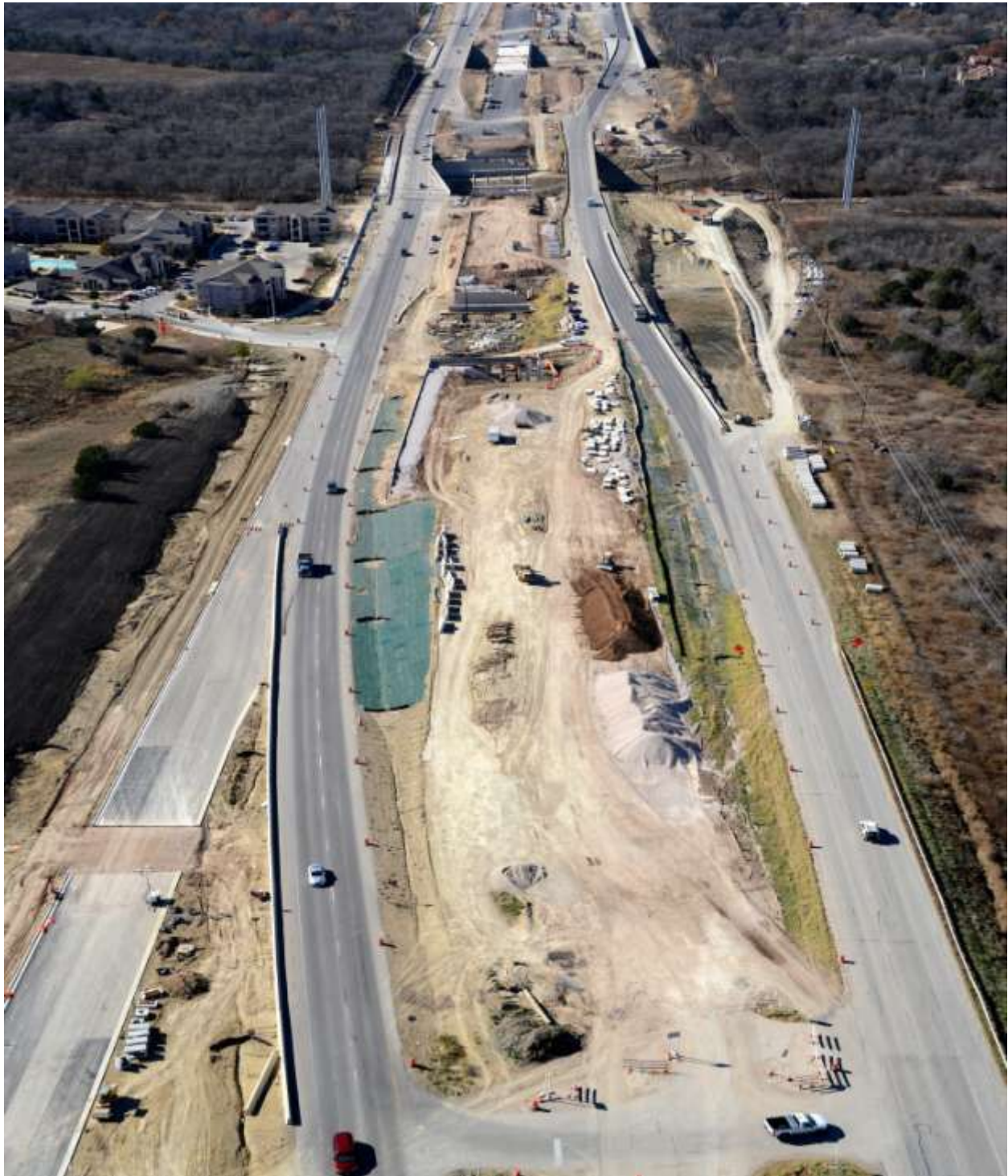
US 290 East looking west at Mokan Crossing (Taken 12/18/2012)
