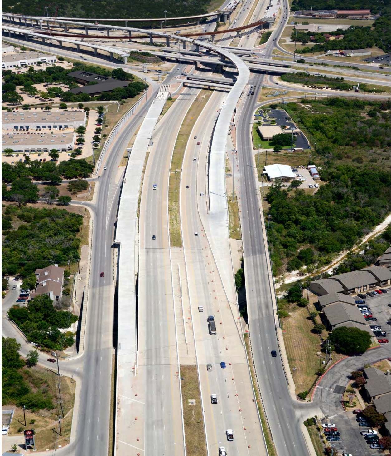
Manor Expressway Phase I Project (Looking South from US 183) (Taken 7/06/2012)
