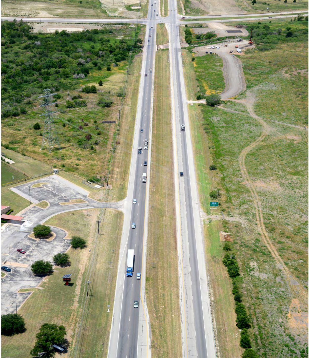
US 290 East looking west from Gilleland Creek (Taken 6/19/2012)
