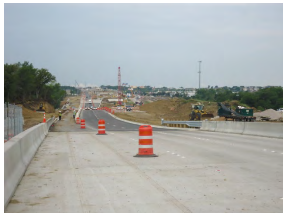
Eastbound frontage road construction at MOKAN crossing (Looking West)
