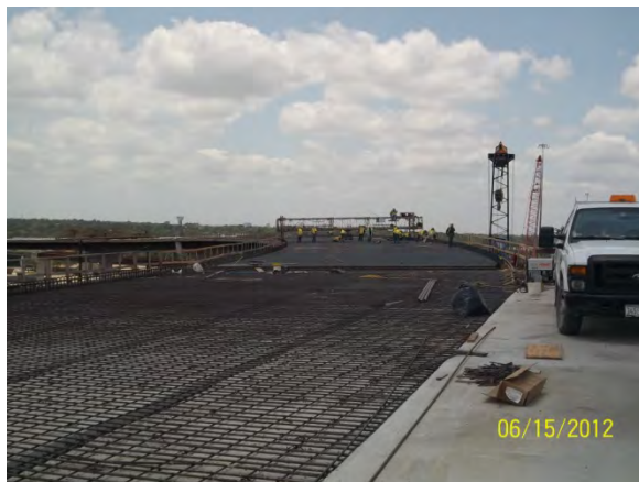
North to East Direct Connector Deck (Looking West)
