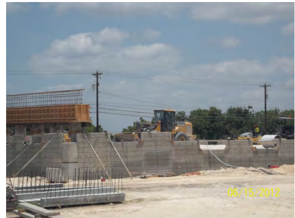
Backfilling Operations @ Retaining Wall 109 (Looking North)
