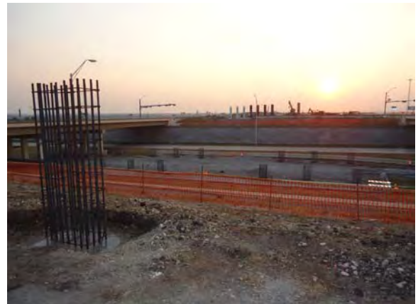
Mainlane Bridge drilled shafts at SH130 (Looking East)
