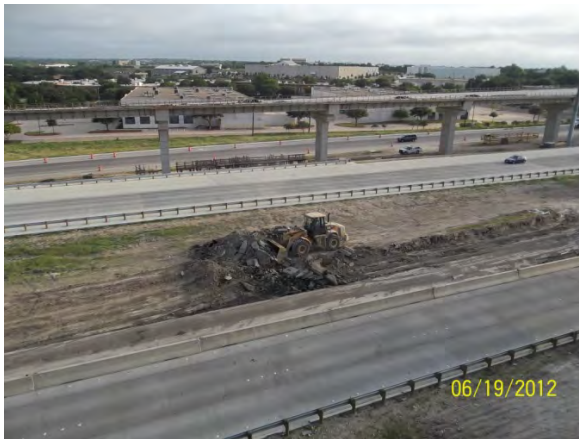
Excavating Median @ US 290 (Looking North)
