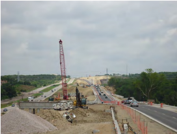
Eastbound mainline construction at Springdale intersection (Looking East)
