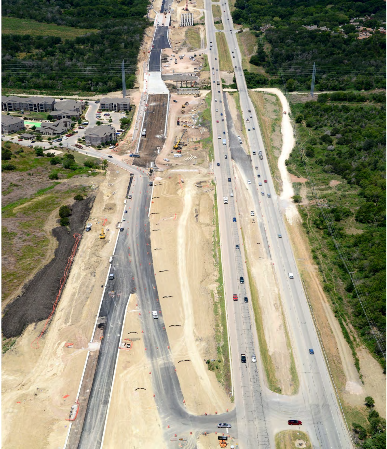
US 290 East looking west at Mokon Crossing (Taken 6/19/2012)
