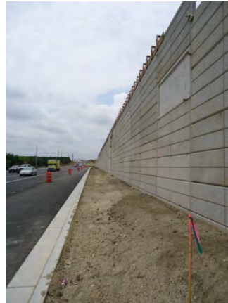
Retaining Wall S1-01 along the eastbound frontage road (Looking West)
