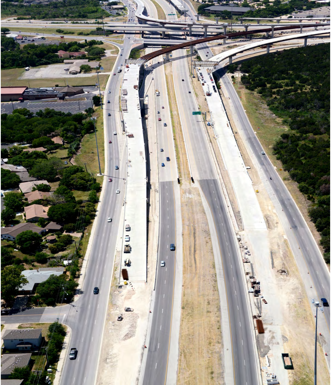
Manor Expressway Phase I Project (Looking North from US 183) (Taken 7/06/2012)
