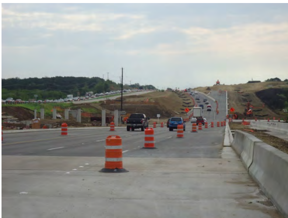
Eastbound frontage road construction at MOKAN crossing (Looking East)
