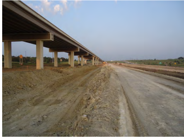
Excavation and Embankment for the eastbound mainlanes at SH130 (Looking West)
