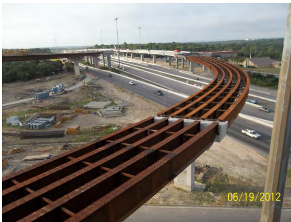
West to South Direct Connector Steel Girders (Looking South)
