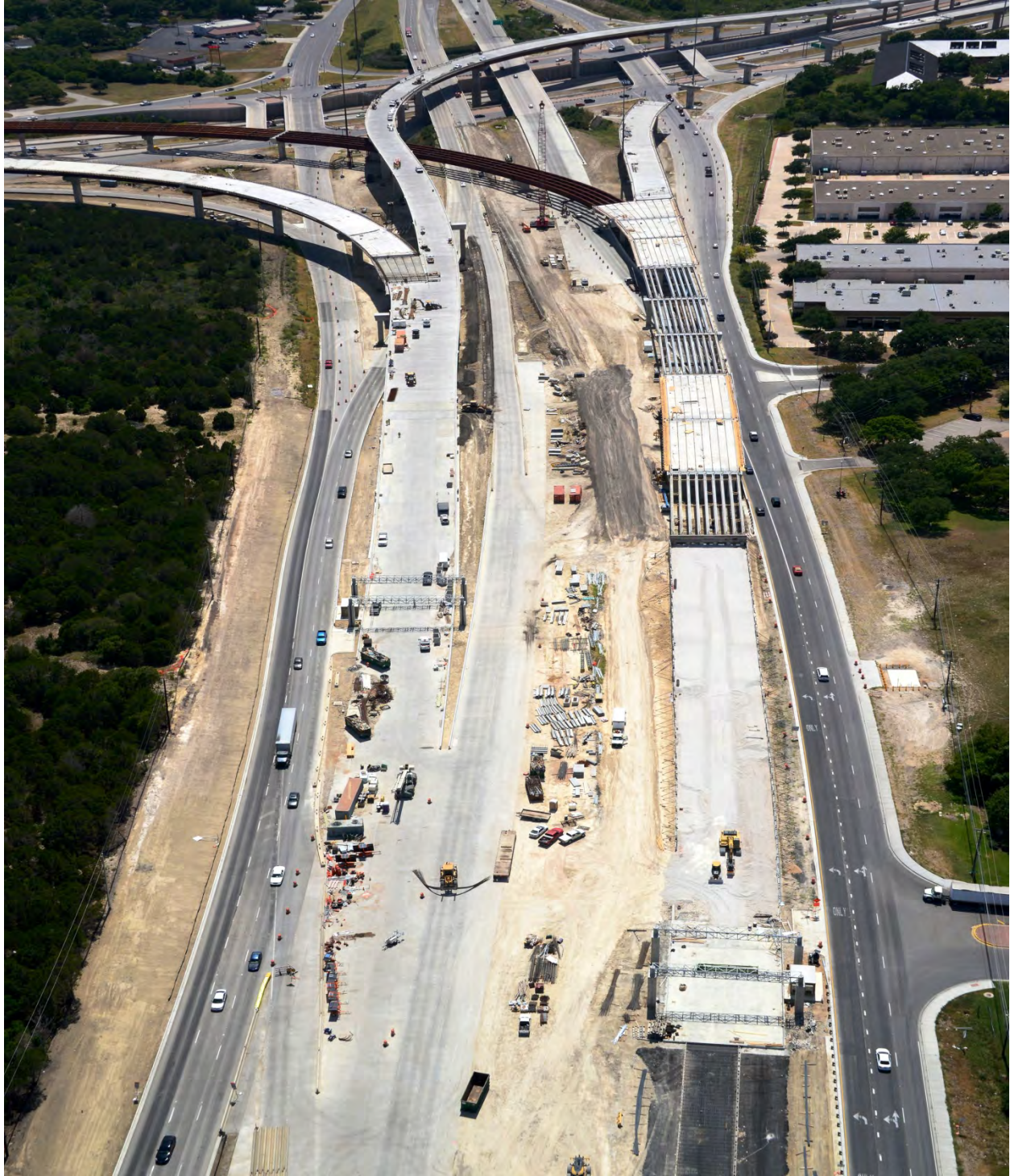
Manor Expressway Phase I Project (Looking West from US 290) (Taken 7/06/2012)
