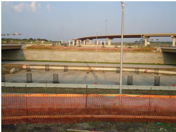
Mainlane Bridge drilled shafts at SH130 (Looking West)
