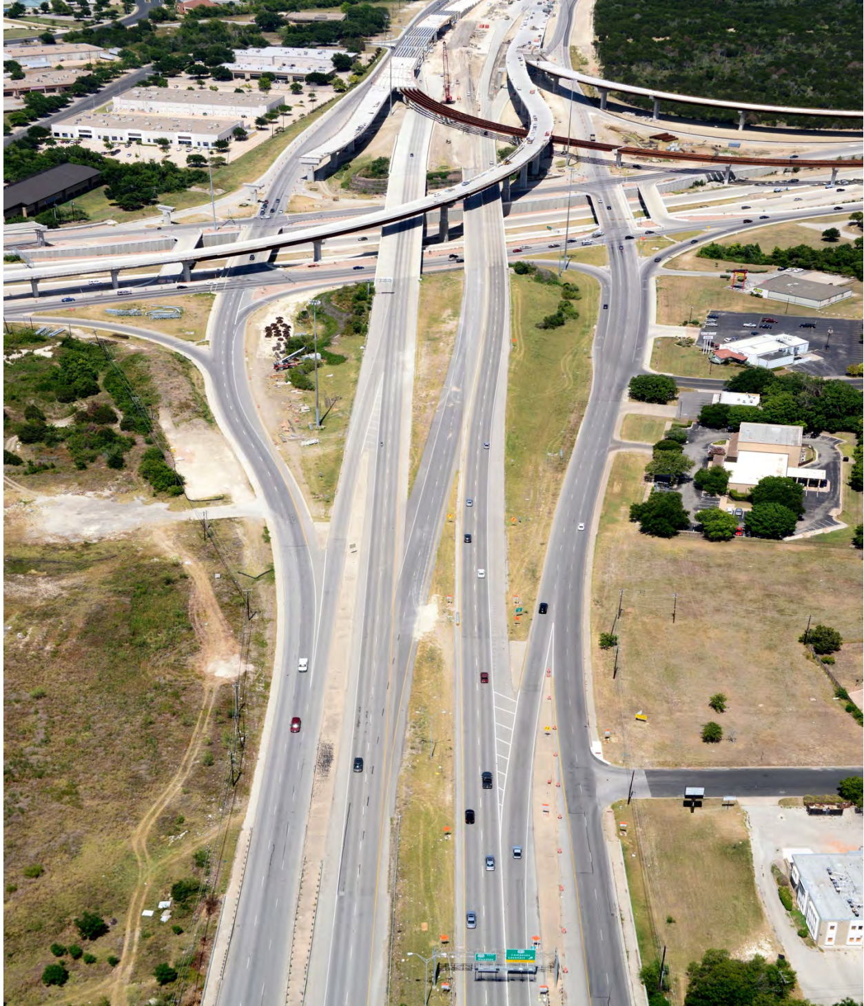
Manor Expressway Phase I Project (Looking East from US 290) (Taken 7/06/2012)
