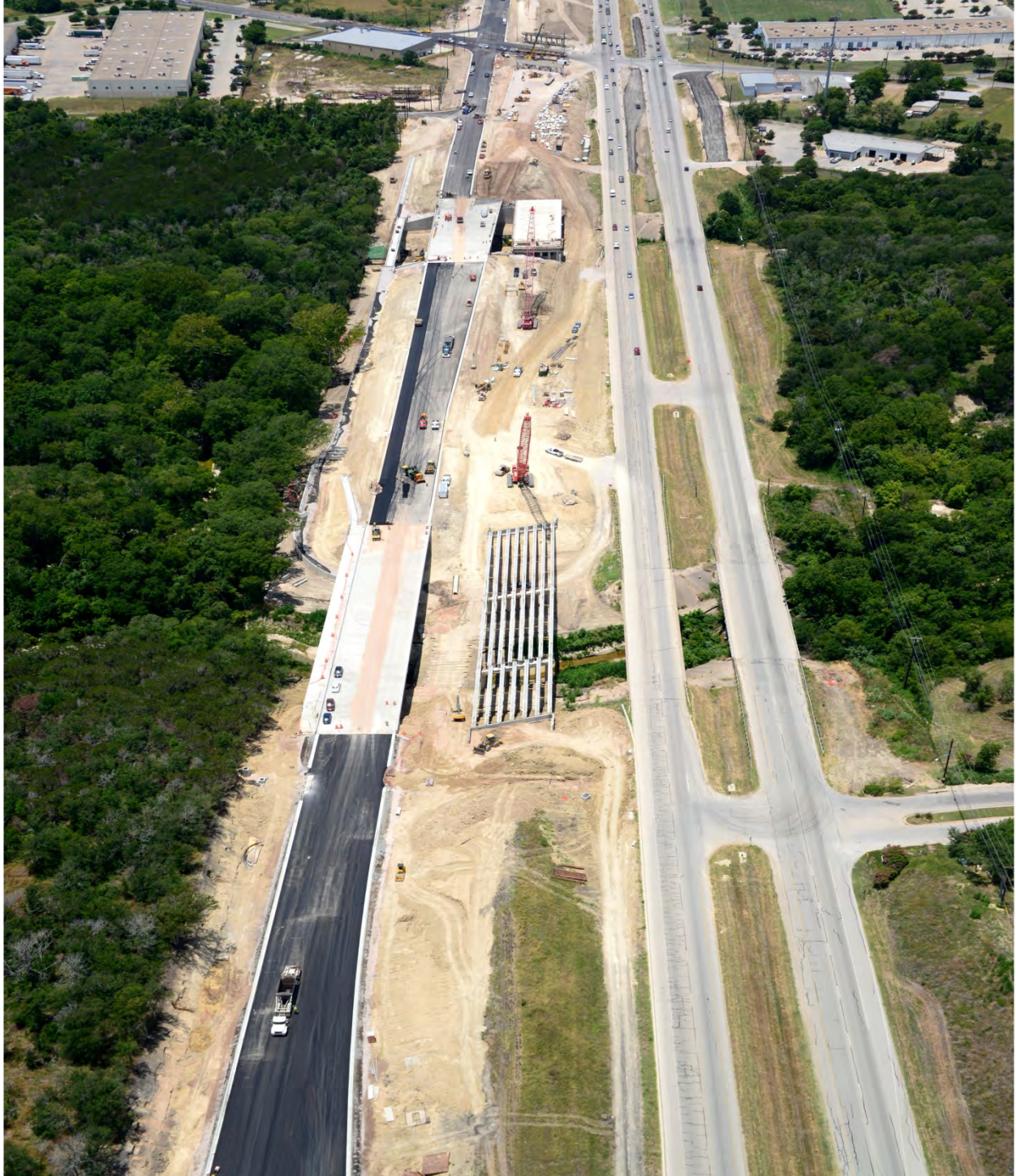
US 290 East at Chimney Hill Blvd looking west (Taken 6/19/2012)
