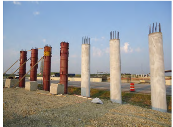
Mainlane Bridge drilled shaft extensions at SH130 (Looking West)
