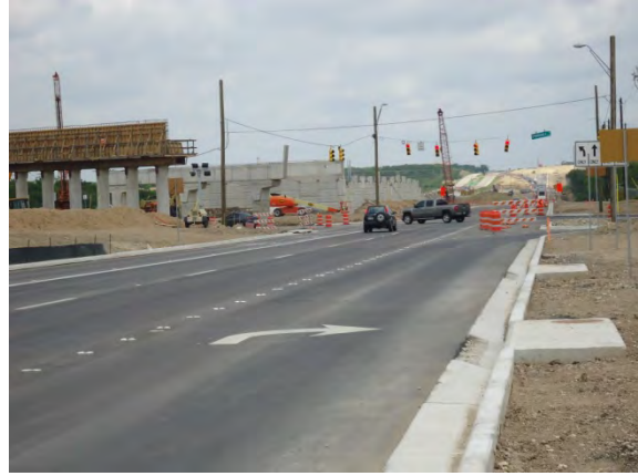
Eastbound frontage road at Springdale intersection (Looking East)
