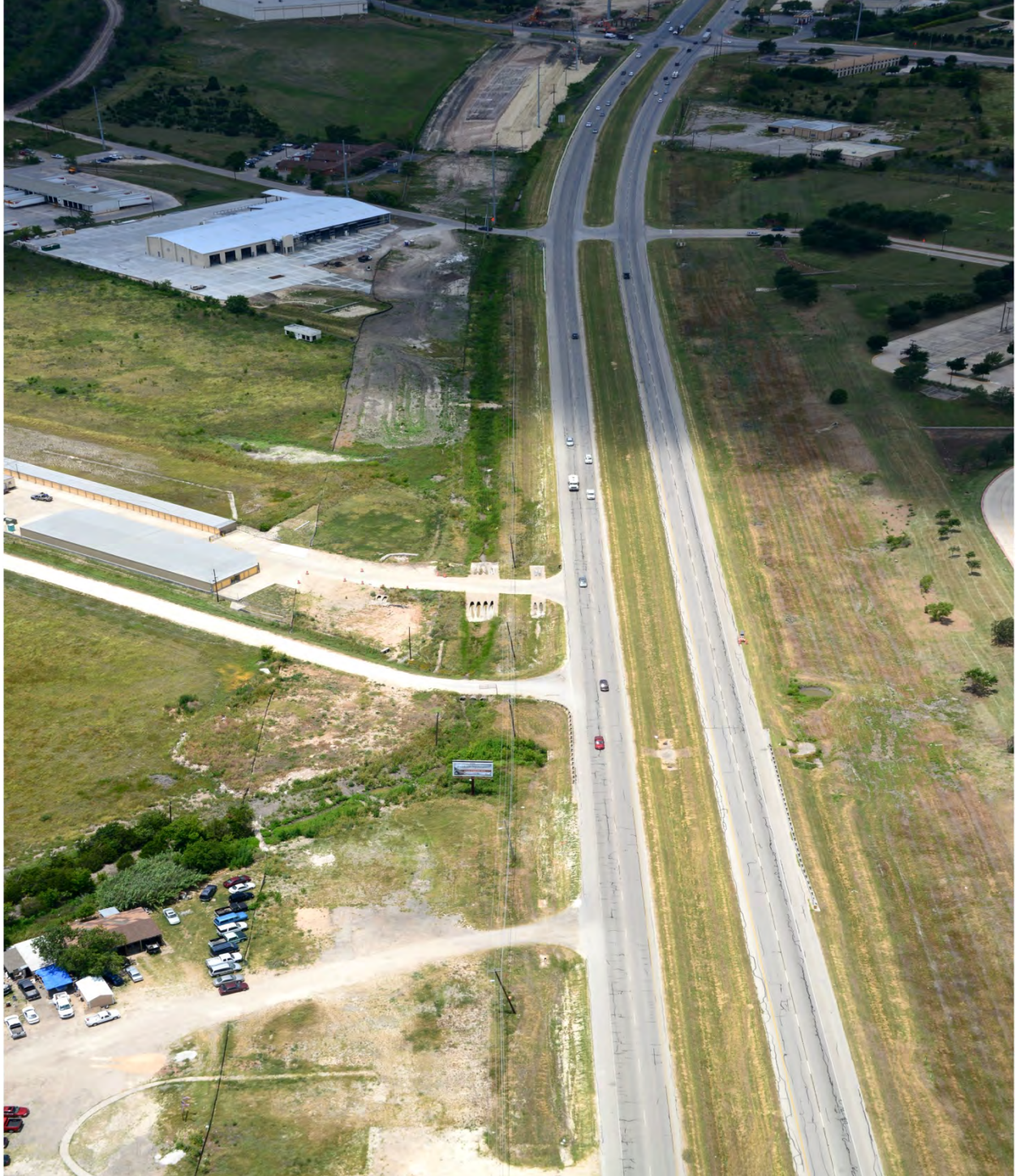
US 290 East at Crofford Lane Intersection looking west (Taken 6/19/2012)
