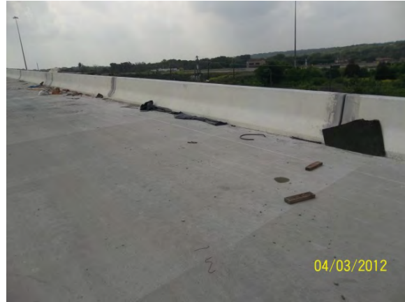
T 501 Mod Rail on US 290 WB Approach Slab (Looking North)
