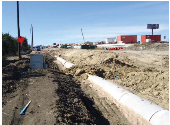
Reinforced concrete pipe installation (Looking East)
