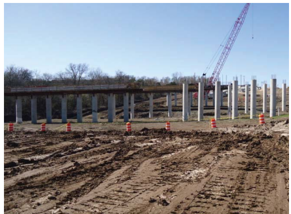
Bridges at Walnut Creek Tributary #5 (Looking East)
