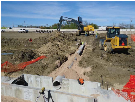
Reinforced concrete pipe installation (Looking North)
