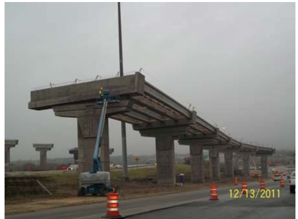
Beam Construction along West to North Direct Connector (Looking West)
