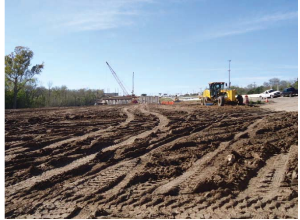
Earthwork embankment west of Walnut Creek (Looking East)
