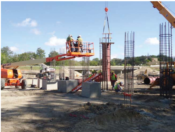
Drilled shaft extensions for bridge at Walnut Creek (Looking North)
