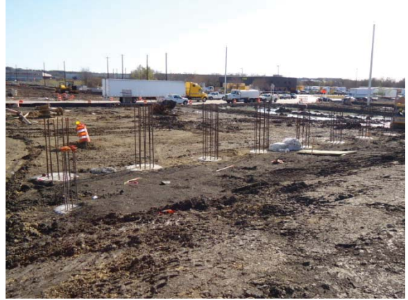
Drilled shafts for bridge at Tuscany Way (Looking East)
