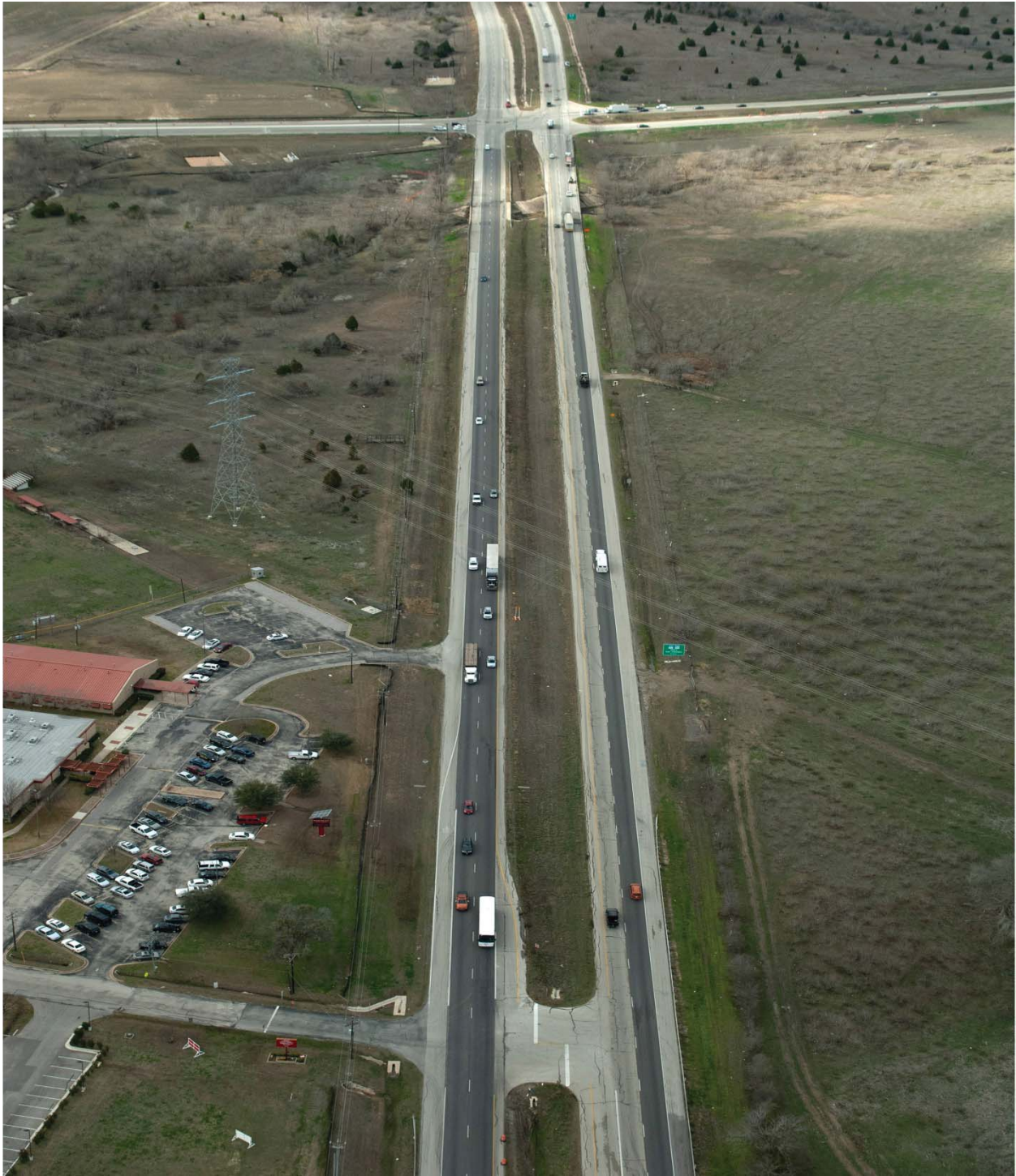
US 290 East looking west from Gilleland Creek (Taken 1/10/2012)
