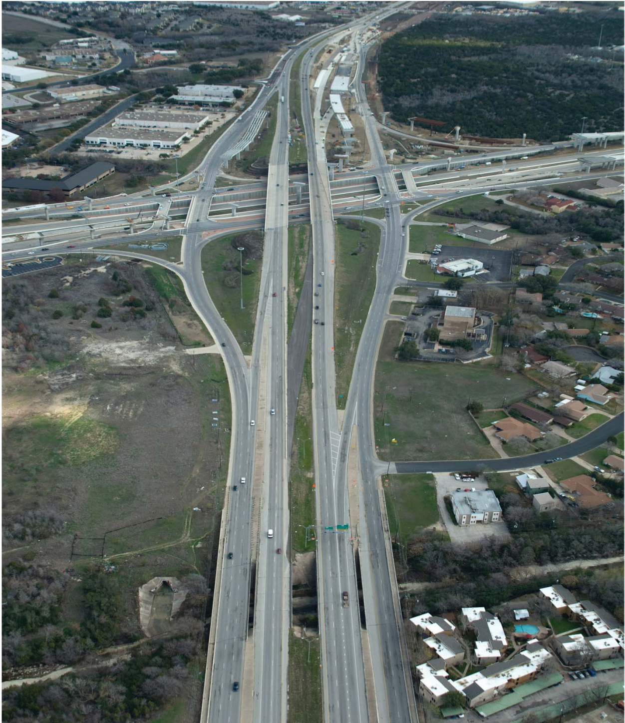
Manor Expressway Phase I Project (Looking East from US 290) (Taken 1/10/2012)
