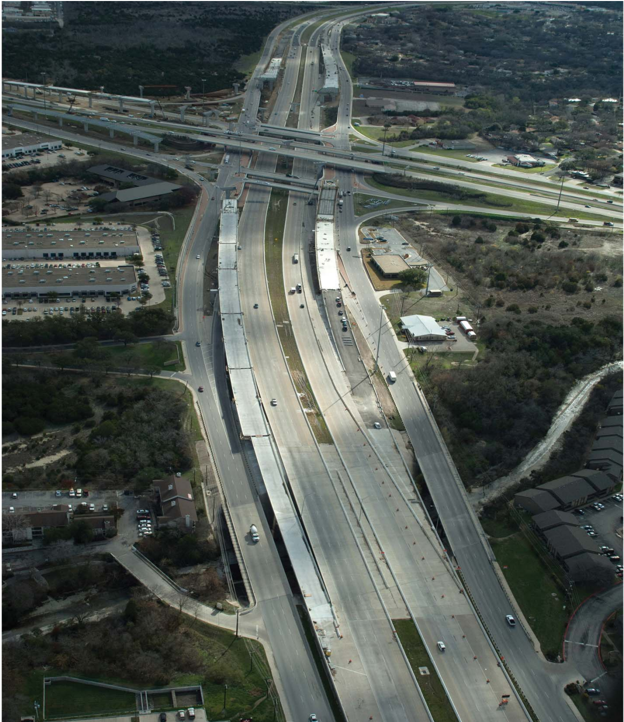
Manor Expressway Phase I Project (Looking South from US 183) (Taken 1/10/2012)
