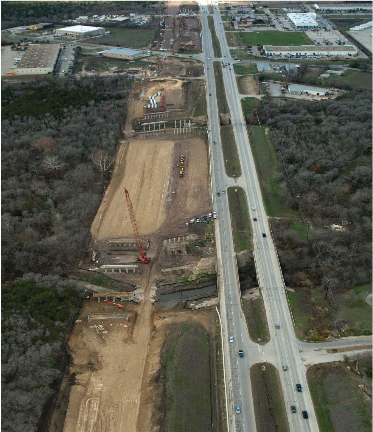
US 290 East at Chimney Hill Blvd looking west (Taken 1/10/2012)
