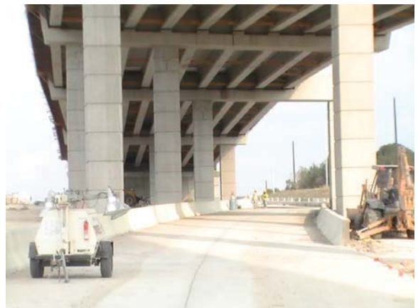
Pavement and rail construction along main lane off-ramp (Looking East)
