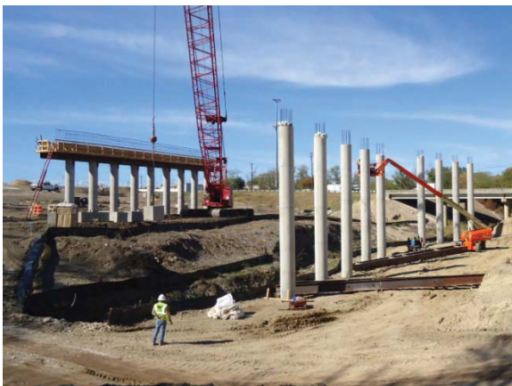
Bridges at Walnut Creek Tributary #5 (Looking North)
