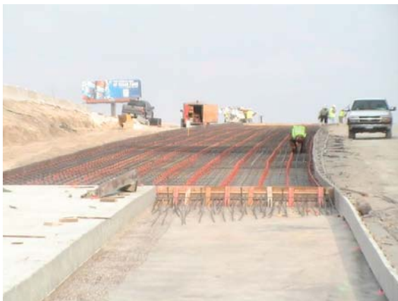
Eastbound main lane roadway construction (Looking East)
