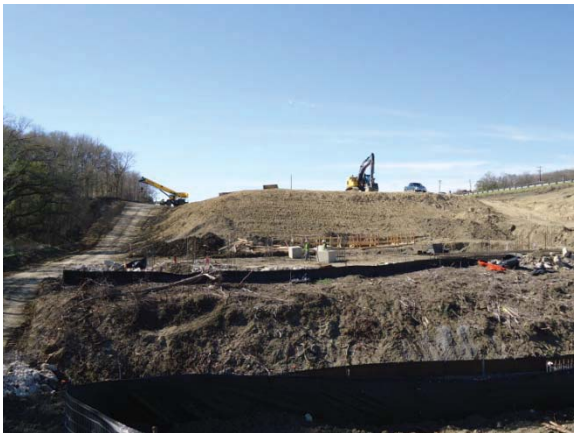
Earthwork embankment west of MOKAN (Looking East)
