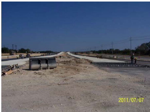
Mainlane concrete pavement from Block House Creek and Crystal Falls
