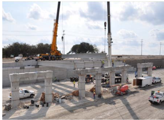
Bridge structure work at Scottsdale Drive
