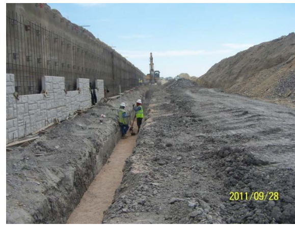
Installing stormwater drainage system at the cut at Scottsdale Drive
