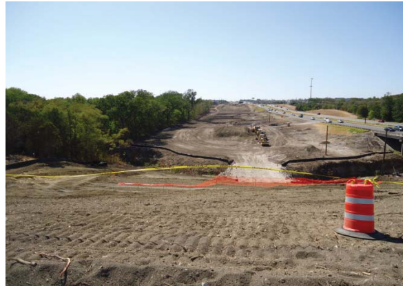
Cleared right-of-way east of Walnut Creek (Looking West)
