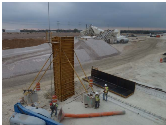
Preparations for an exit ramp toll gantry
