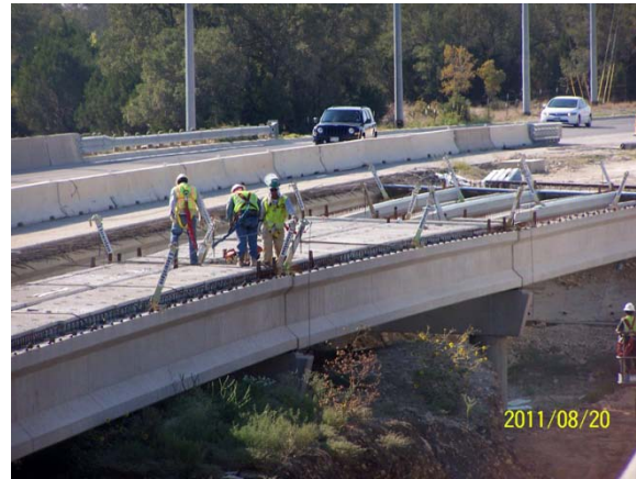
Placing prefabricated bridge deck panels at the Block House Creek bridges
