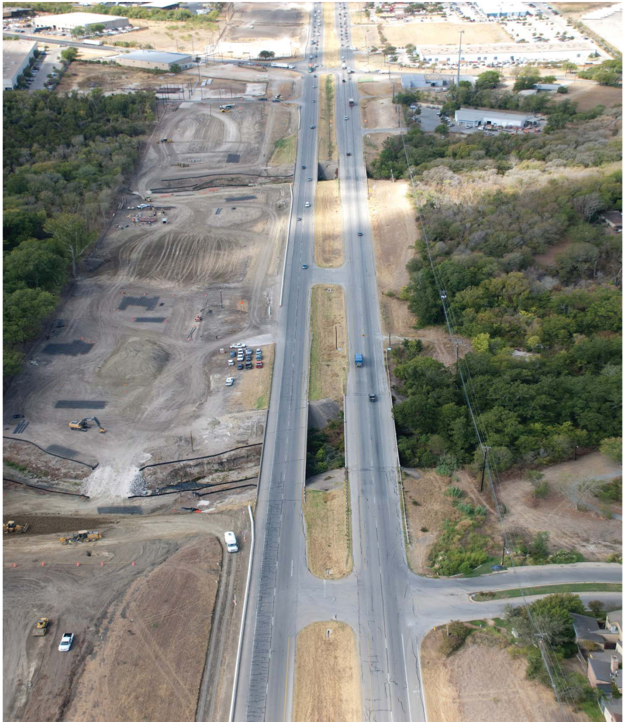
US 290 East at Chimney Hill Blvd looking west (Taken 10/7/2011)
