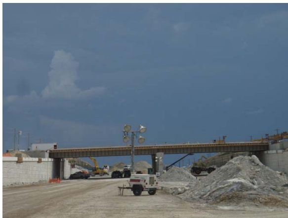
Looking northward at the Scottsdale Drive Bridges
