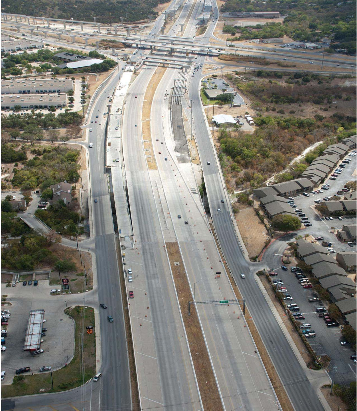
Manor Expressway Phase I Project (Looking South from US 290) (Taken 10/7/2011)
