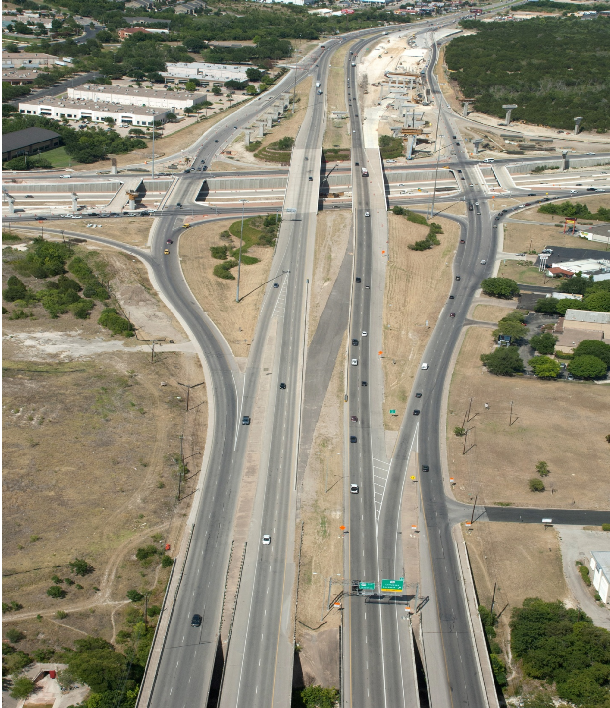
Interchange construction looking east (Taken 7/12/2011)
