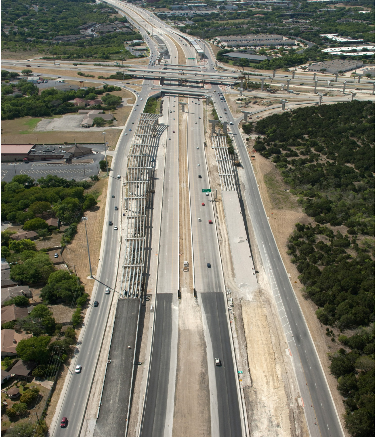
Interchange construction looking north (Taken 7/12/2011)
