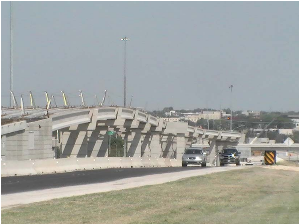
South to East direct connector looking north from US 183 median
