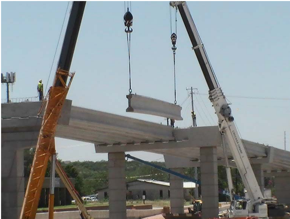
Setting of beams at the south to east direct connector [taken June 14, 2011]
