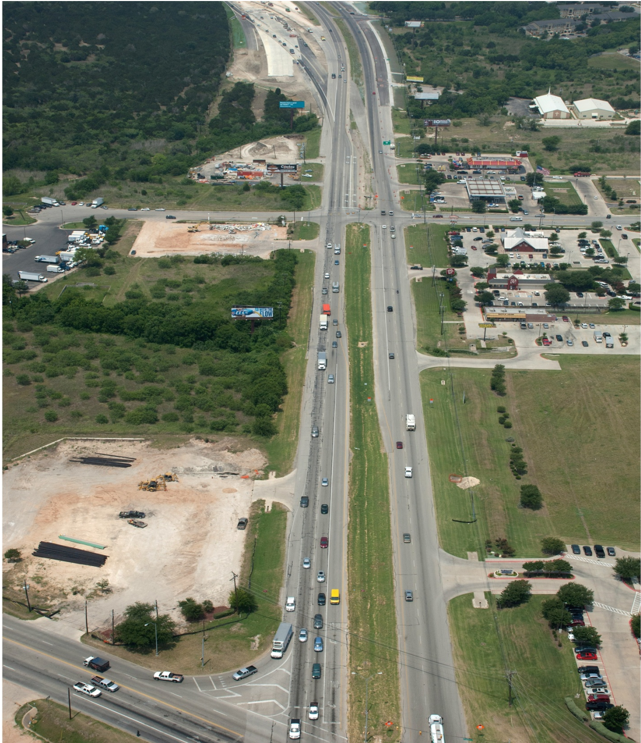
US 290 East at Tuscany Way looking west (Manor Expressway Direct Connectors at US 183 Project in background) (Taken 6/7/2011)
