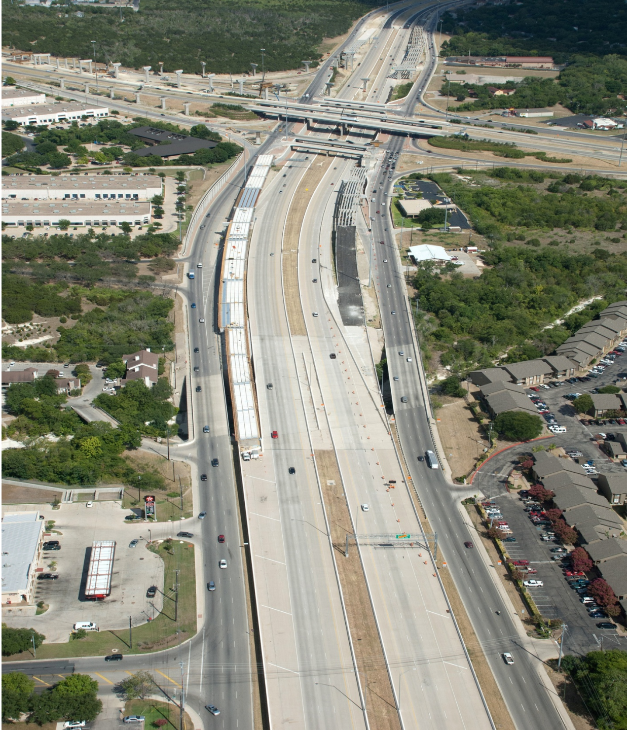
Interchange construction looking south (Taken 7/12/2011)
