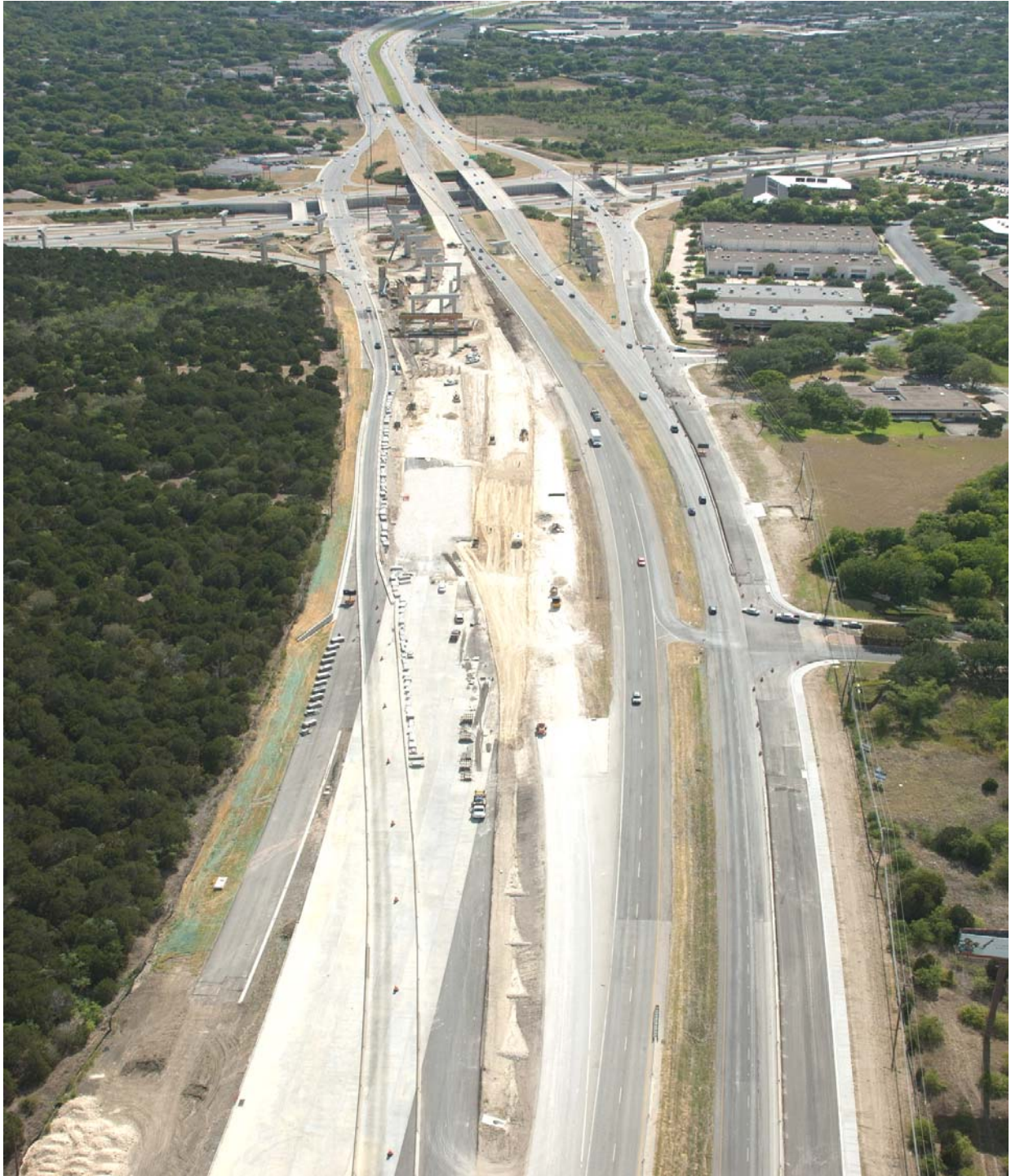
Interchange construction looking west (Taken 7/12/2011)
