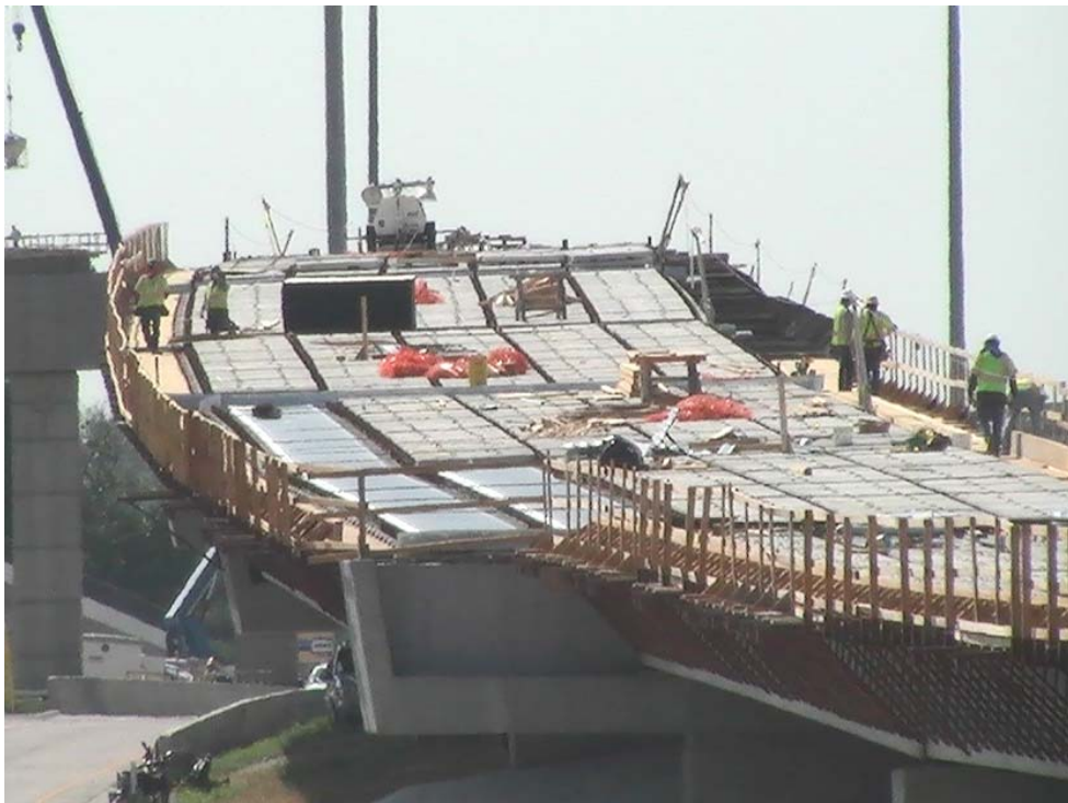
West to North direct connector Spans 5 & 6 (Taken 7/6/2011)
