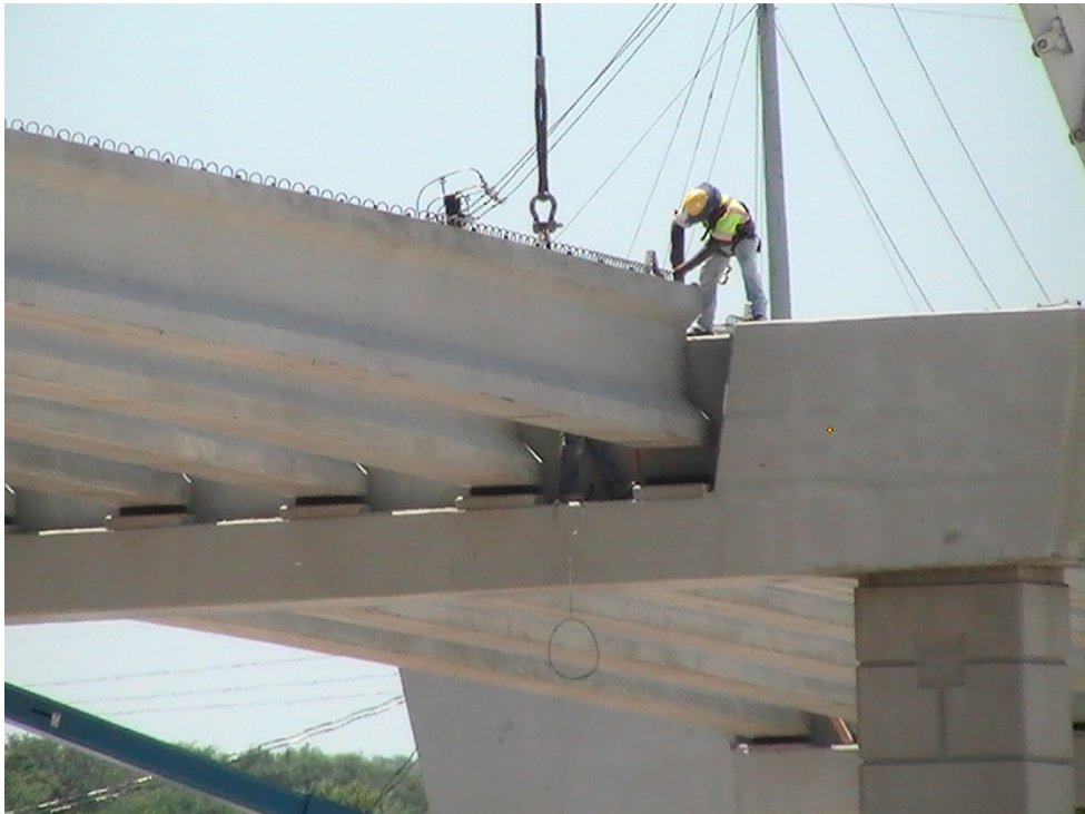
Type IV beam setting at South to East direct connector (Taken 6/14/2011)
