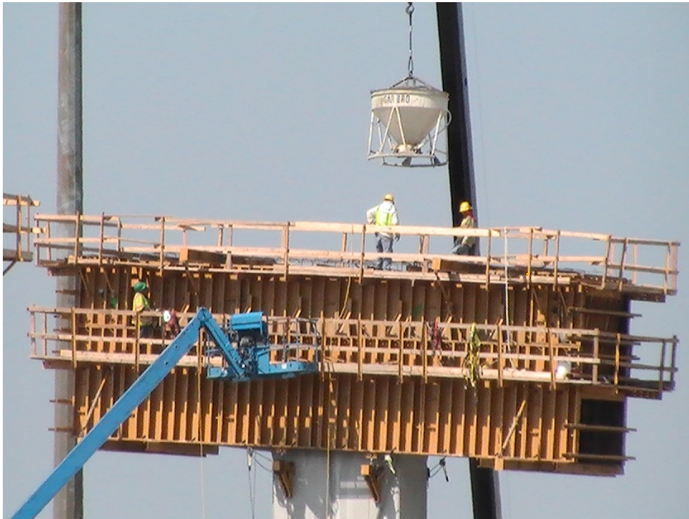
South to East Direct Connector Bent 14 Cap Pour (Taken 7/6/2011)
