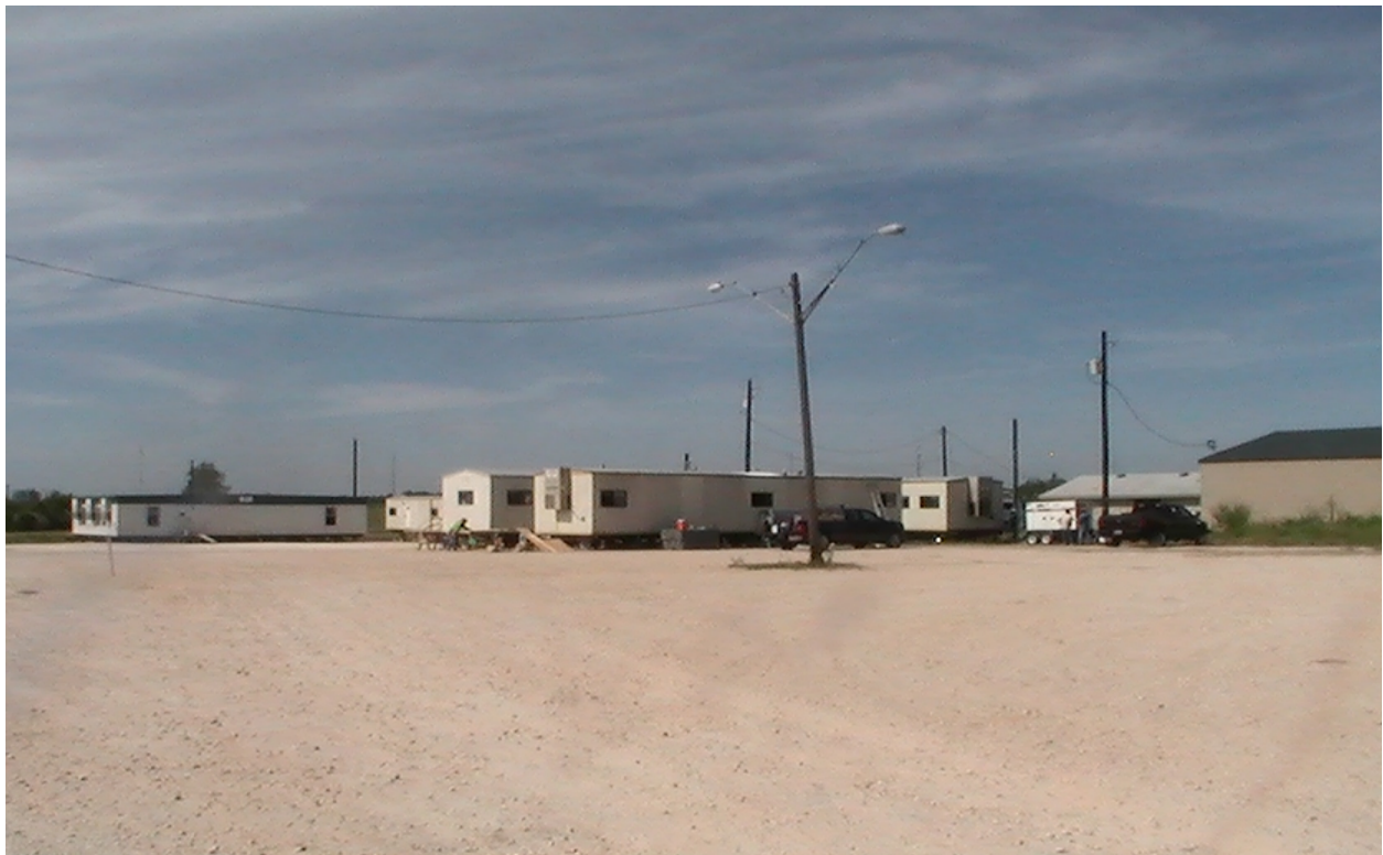
Mobilization of the Project field office along the existing US 290 East facility [taken July 14, 2011]
